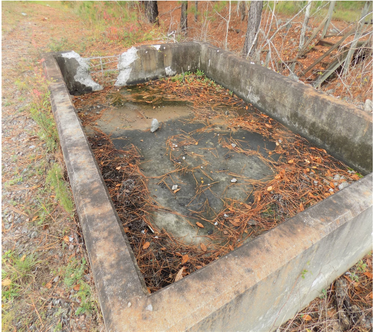
Photo 4 -Fuel Oil Tank Concrete Containment Dike (Looking East) After Decommissioning
