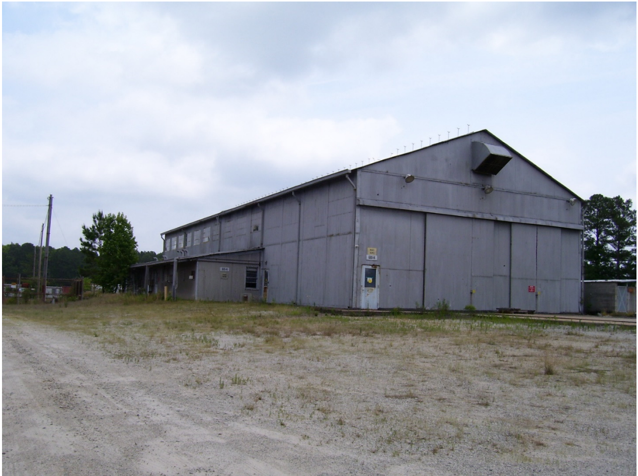
Photo 1 – Building 690-N, Process Heat Exchanger Repair Facility (Looking Southeast) Before Decommissioning
