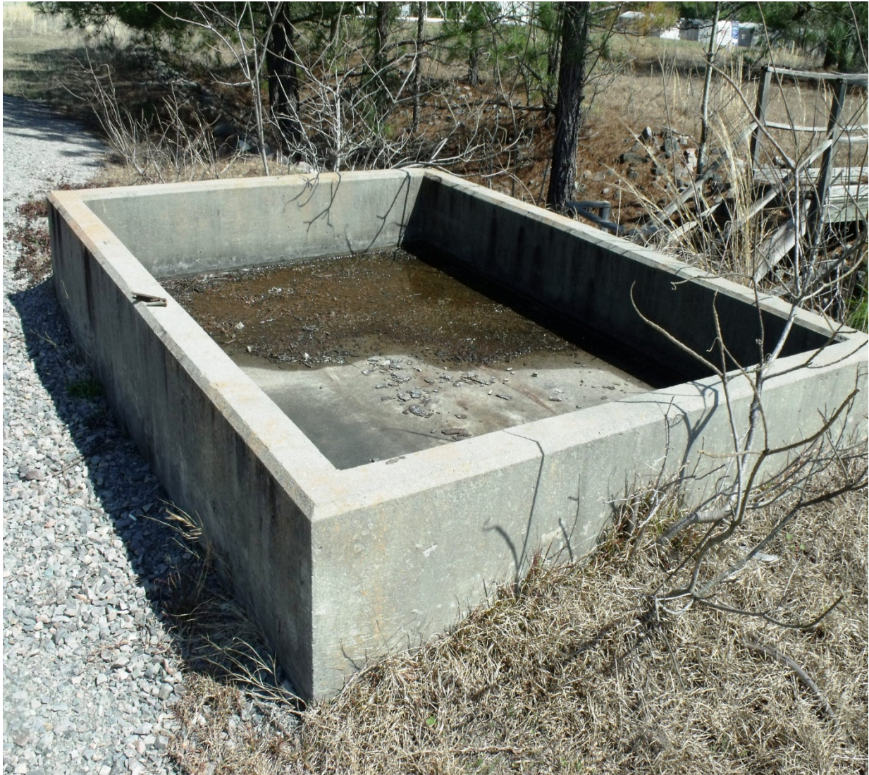
Photo 3 -Fuel Oil Tank Concrete Containment Dike (Looking East) Before Decommissioning
