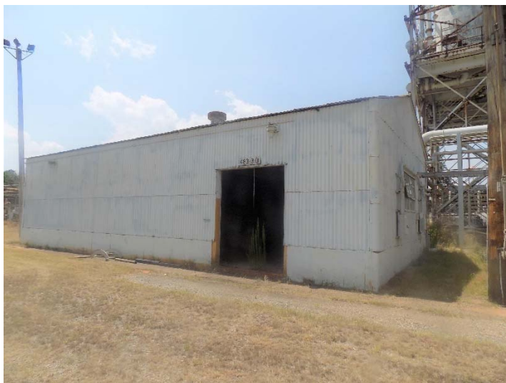
Figure 1. Building 483-3D, D-Area Electrical Control Building
