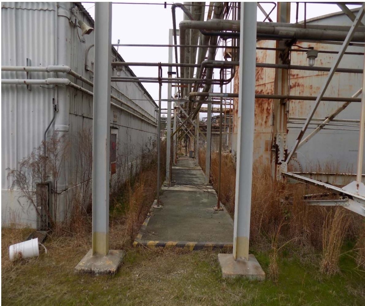
Figure 7. Building 483-3D Cable Trench
