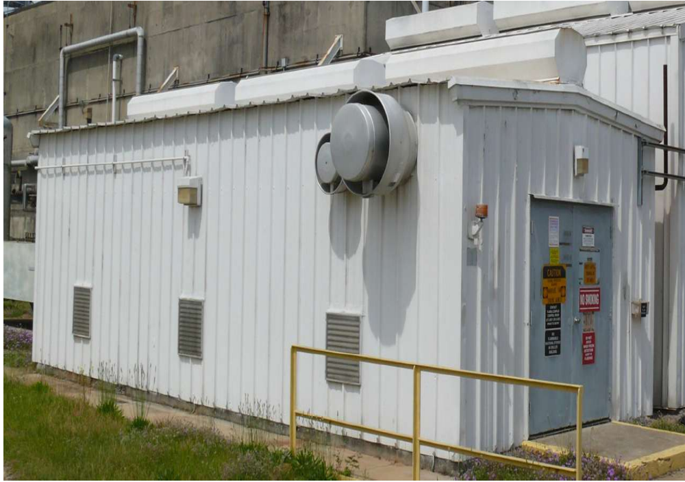
Figure 3: 235-2F from Southeast (Before)
