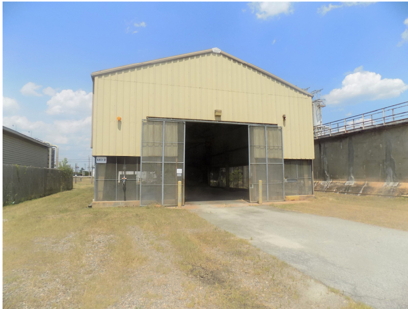
Figure A-1. Building 683-D (Looking East) Before
