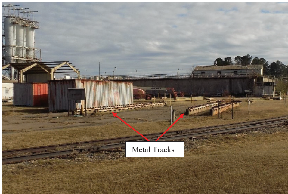
Figure A-6. Ancillary Metal Tracks (Looking Southeast) Before
