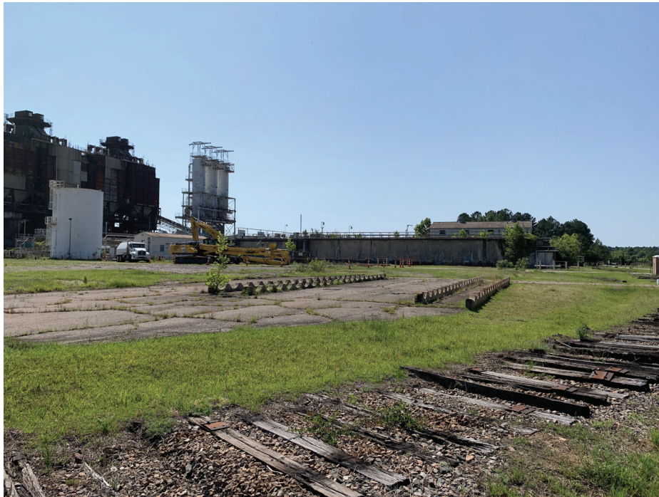
Figure A-7. Ancillary Metal Tracks (Looking Southeast) After
