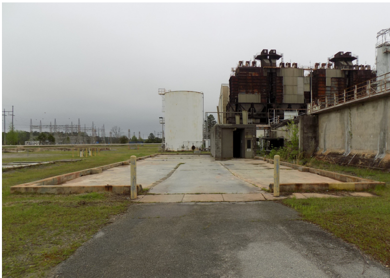
Figure A-2. Building 683-D (Looking East) After Partial Decommissioning by CRO
