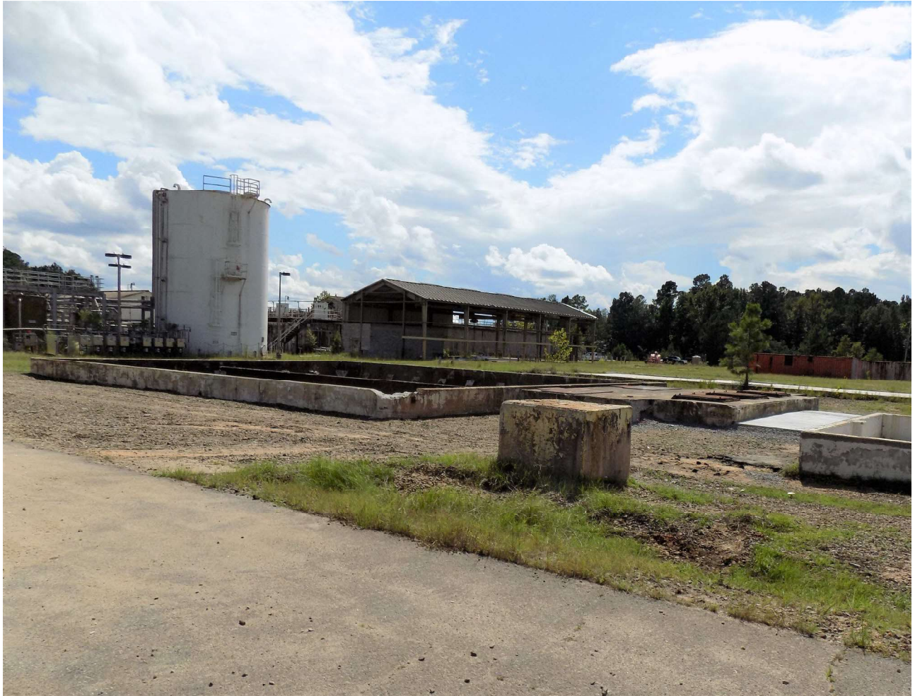
Figure 2: Building 485-D (Looking Southwest) After Decommissioning
