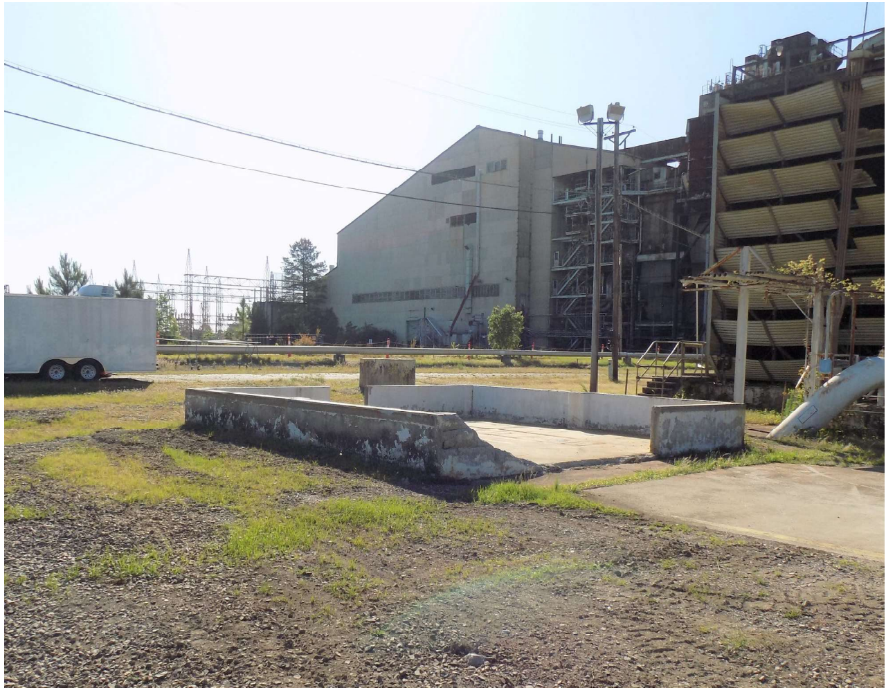
Figure 5: 482-2D (Looking Southeast) After Decommissioning
