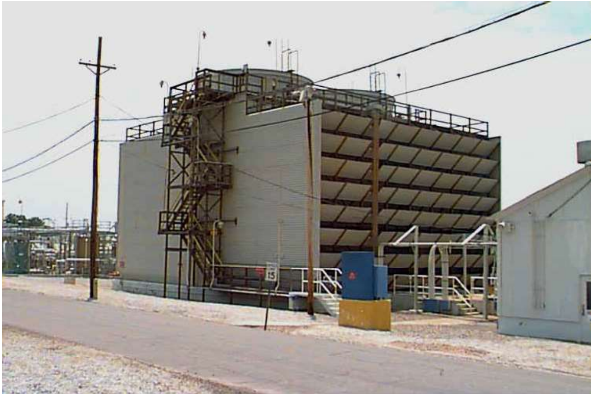
Figure 1: Building 485-D (Looking Southwest) Before Decommissioning
