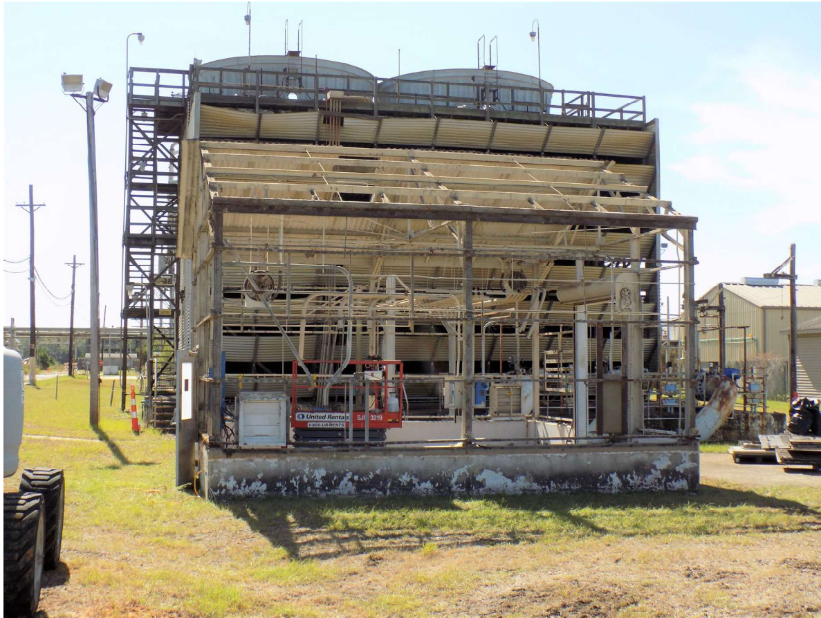
Figure 4: Building 482-2D (Looking South) After Asbestos Abatement
