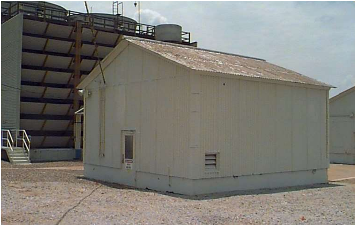
Figure 3: Building 482-2D (Looking Southwest) Before Asbestos Abatement
