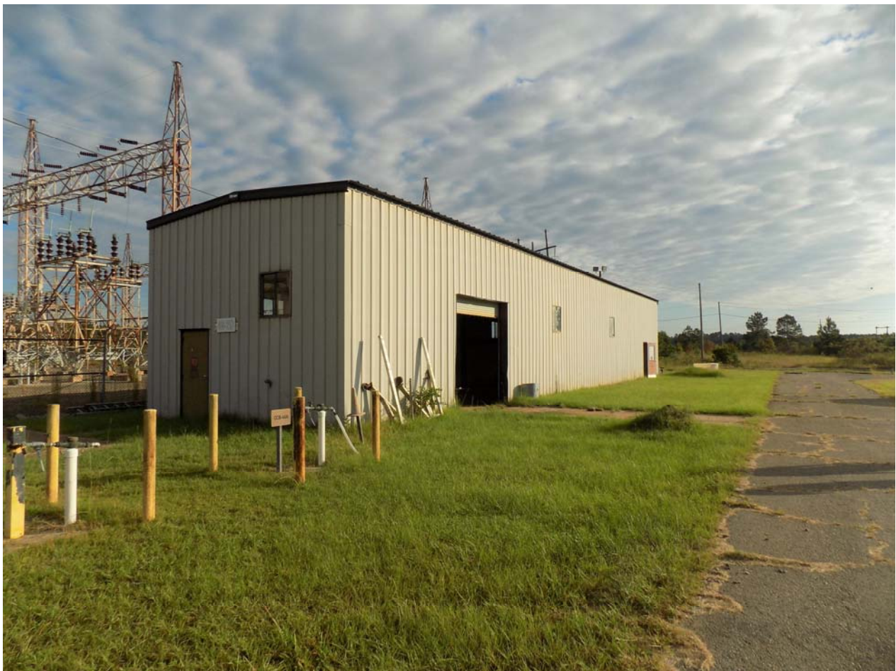
Figure 1. Building 484-15D, D-Area Storage Building
