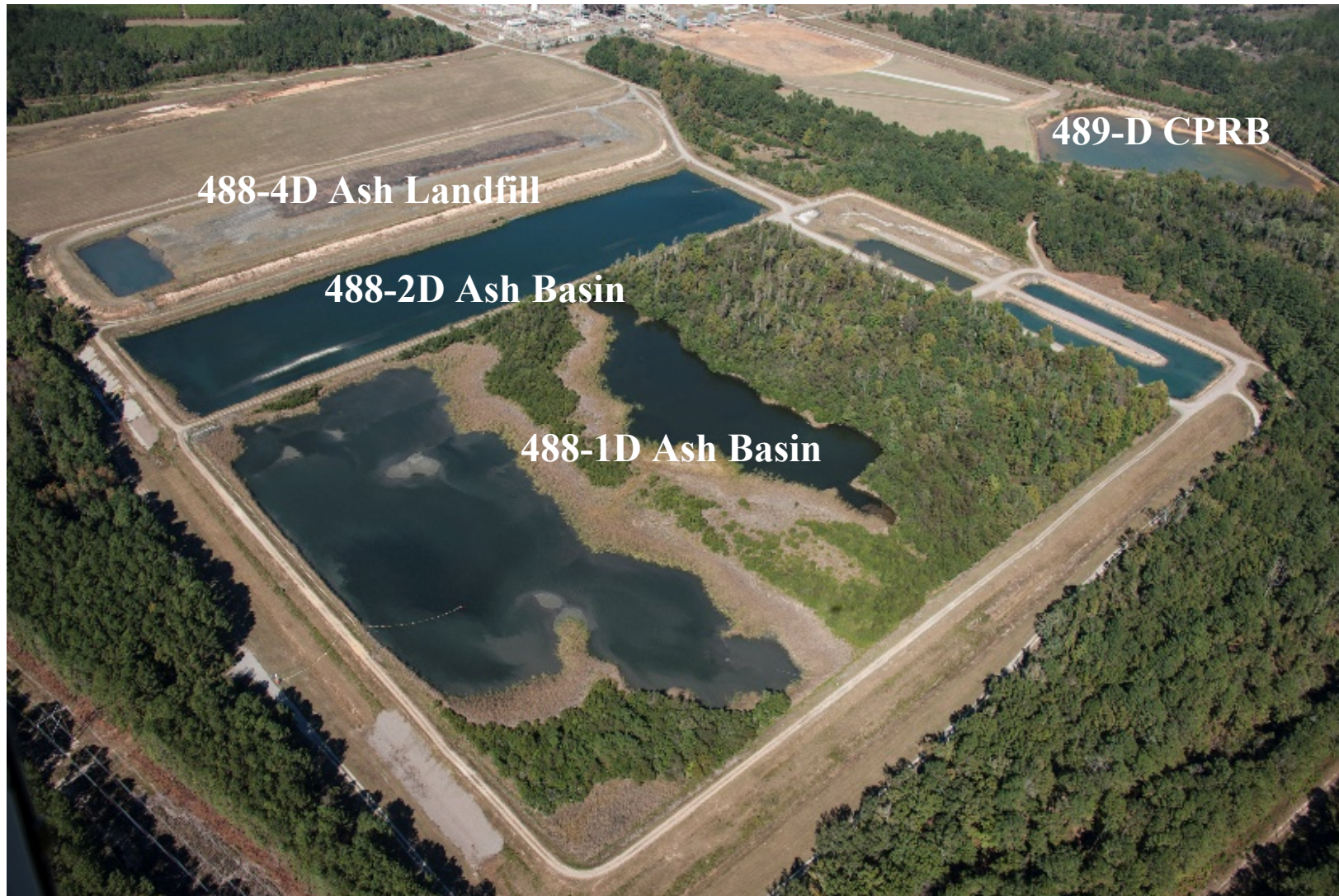
Figure 7. D-Area Project in October 2013 (Before Project Initiation)
