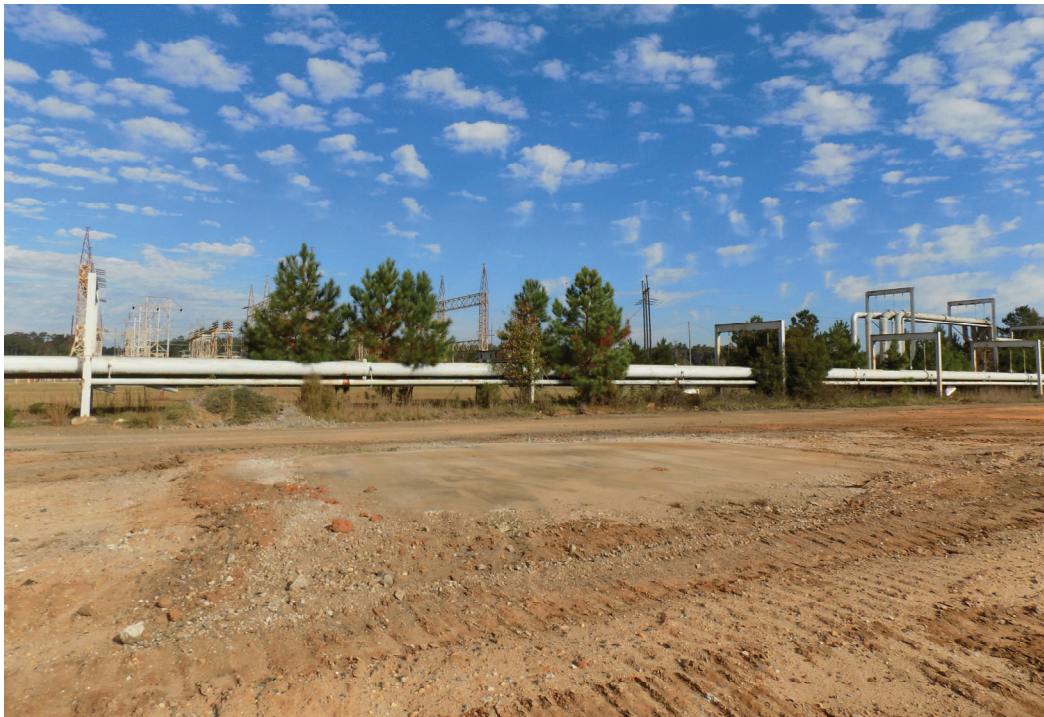
Figure A-8: Conveyor No. 1 Concrete Bunker (Looking Northeast) After Decommissioning
