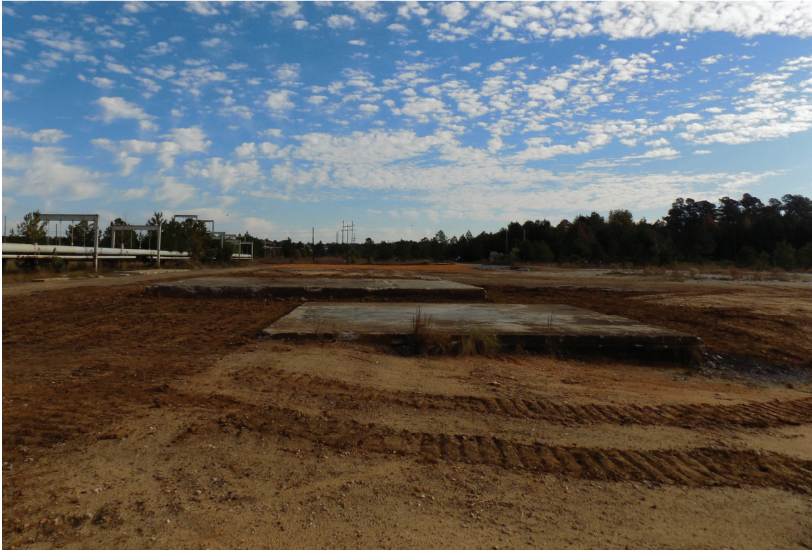
Figure A-14: 484-22D (Looking East) After Decommissioning
