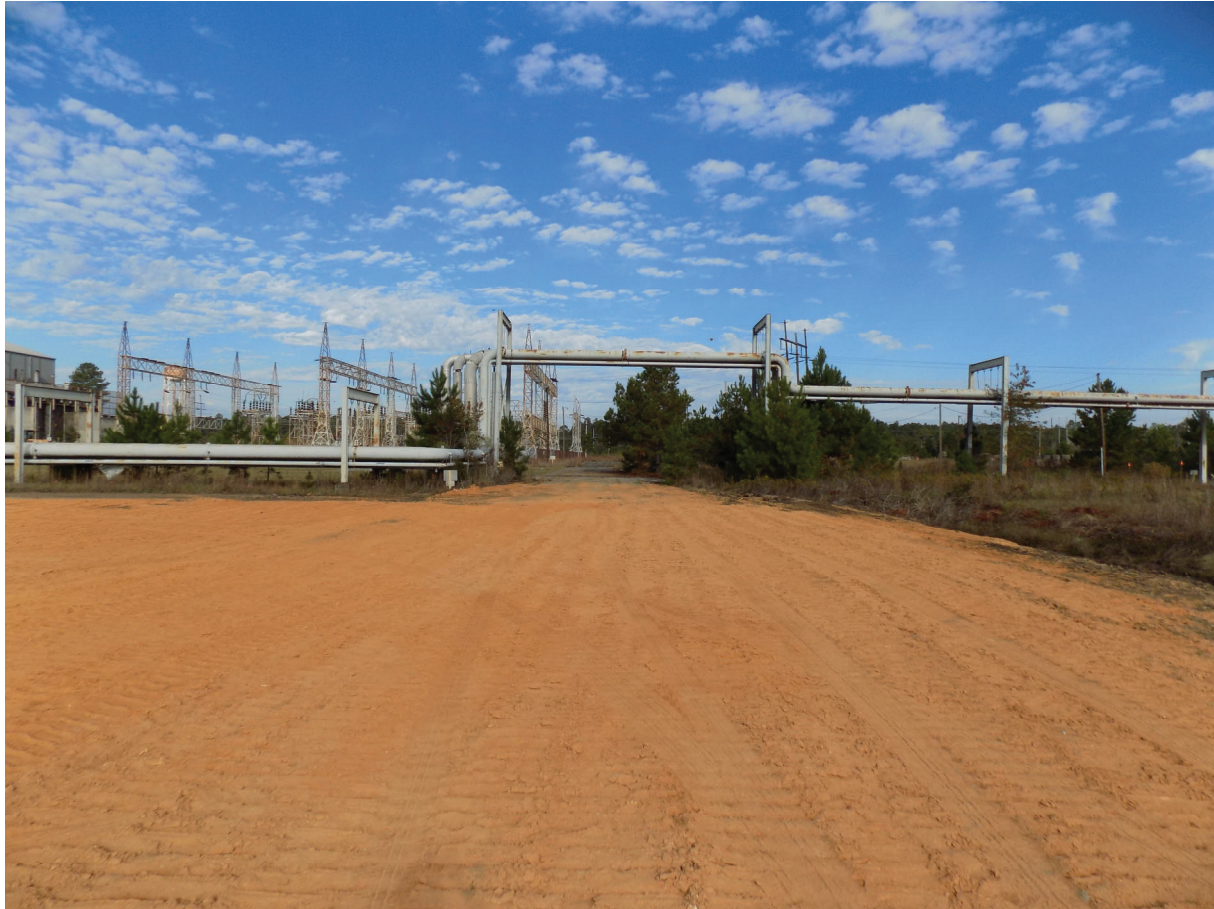
Figure A-2: Building 484-24D (Looking North) After Decommissioning
