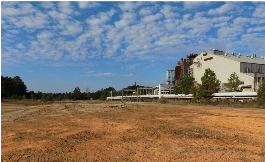
Figure A-10: Conveyor No. 1 and Bunker (Looking Northwest) After Decommissioning
