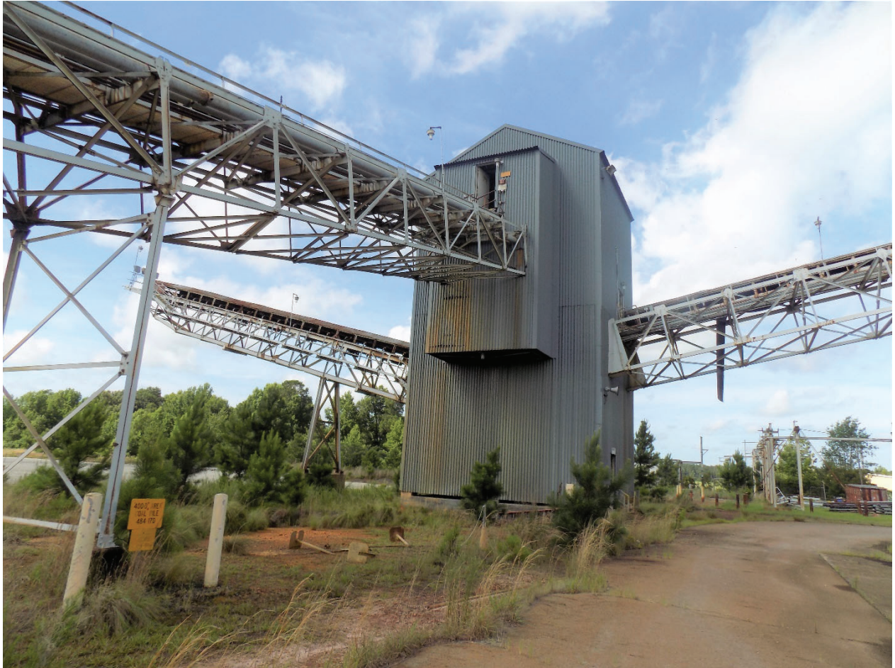
Figure A-21: 484-21D (Looking Southwest) Before Decommissioning
