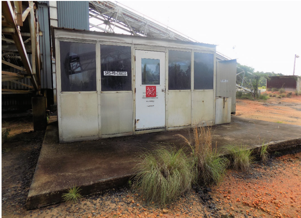
Figure A-18: SRS-PB-EX0033 (Looking Southeast) Before Decommissioning
