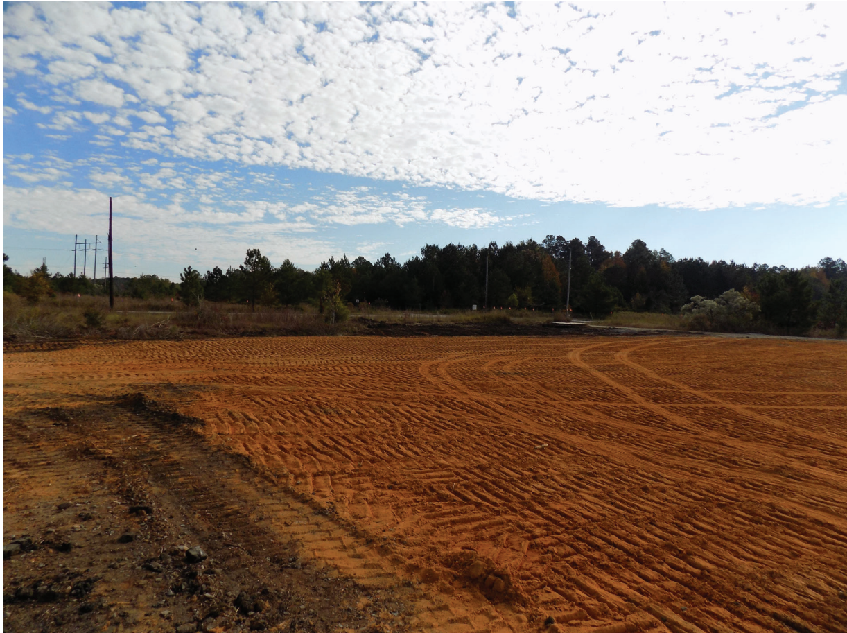
Figure A-6: 483-23D, aka SRS-PB-EX0032, (Looking East) After Decommissioning
