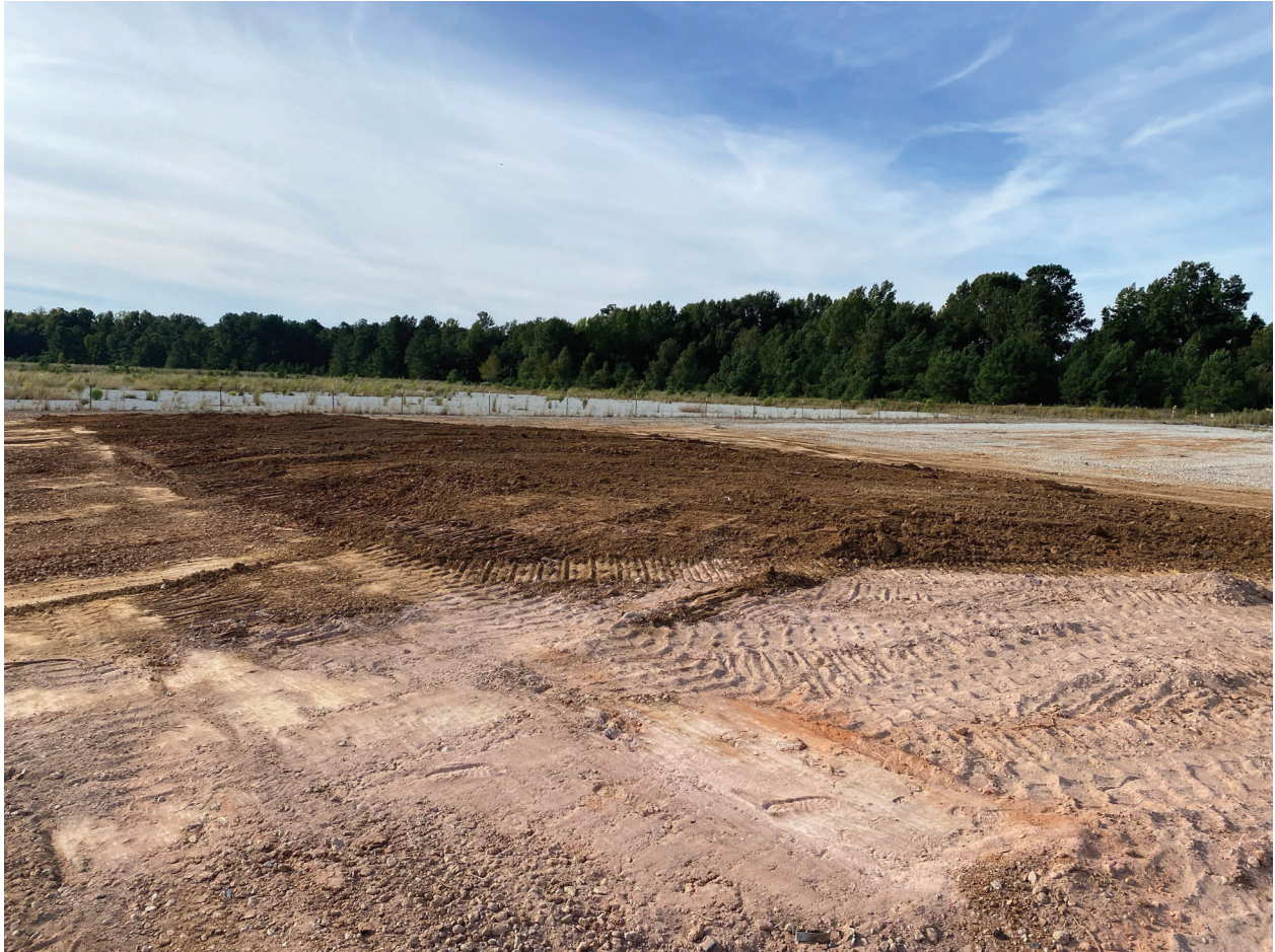
Figure A-17: Conveyor No. 4 Concrete Bunker and Reclaim Hopper (Looking Southwest) After Decommissioning
