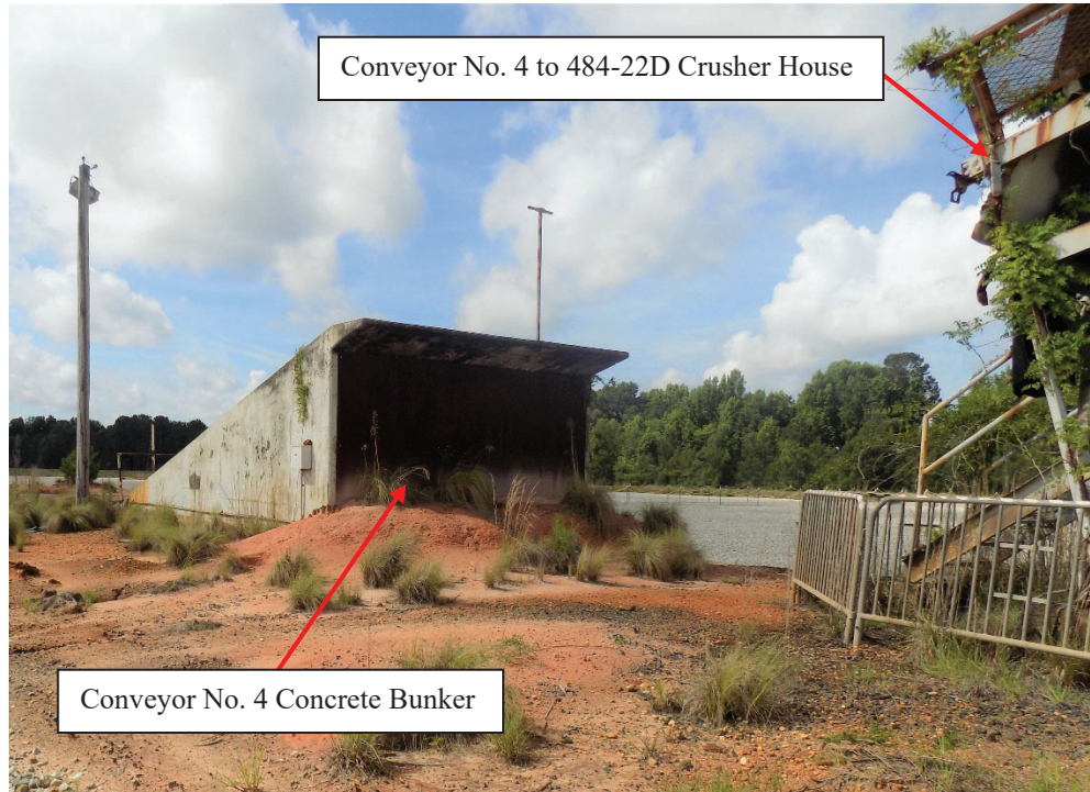
Figure A-15: Conveyor No. 4 Concrete Bunker (Looking Southwest) Before Decommissioning
