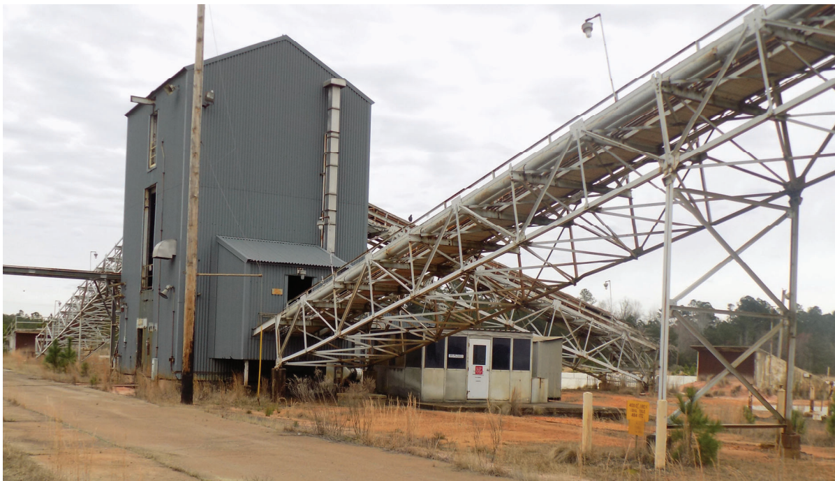
Figure A-13: 484-22D (Looking Southeast) Before Decommissioning
