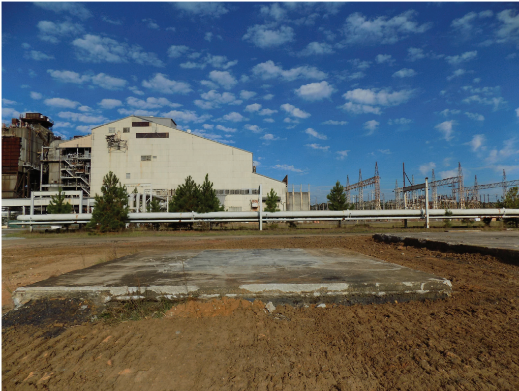
Figure A-20: SRS-PB-EX0033 and SRS-PB-EX0035 (Looking North) After Decommissioning
