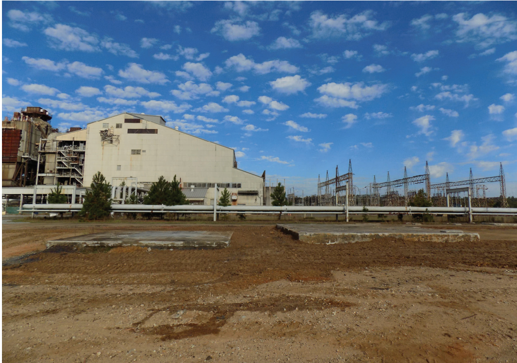
Figure A-12: 484-22D (Looking North) After Decommissioning
