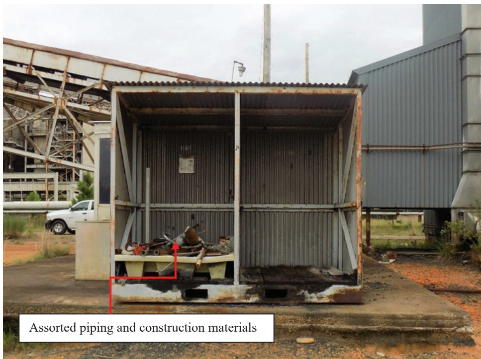
Figure A-19: SRS-PB-EX0035 (Looking North) Before Decommissioning
