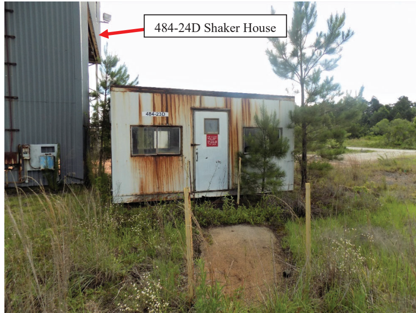
Figure A-3: 483-23D, aka SRS-PB-EX0032, (Looking East) Before Decommissioning
