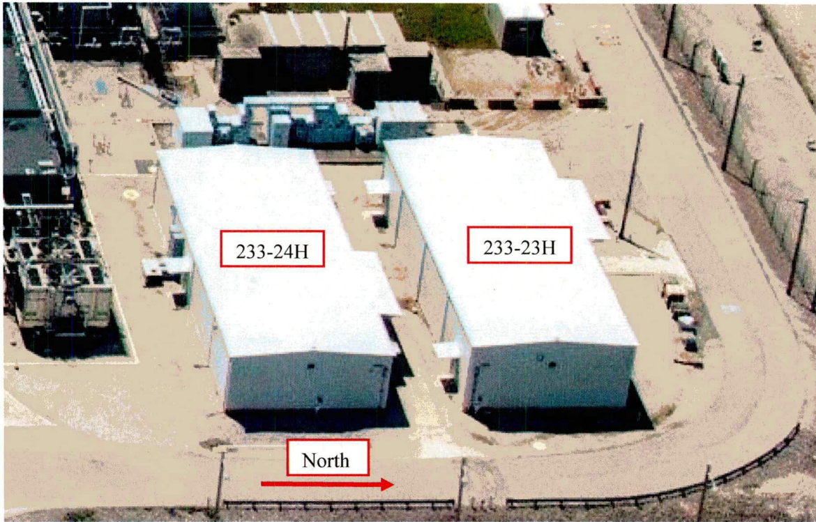
Figure A-1. Aerial of Buildings 233-23H and 233-24H Looking West
