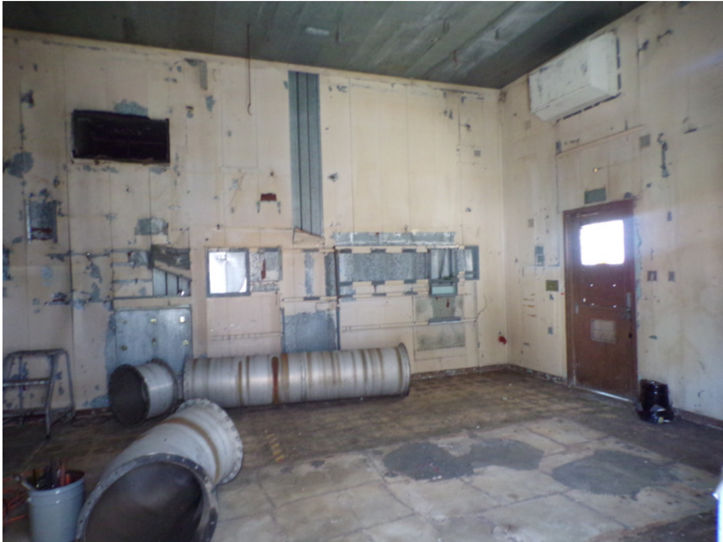
Figure 8. South Process Room Void of Hoods Post Deactivation
