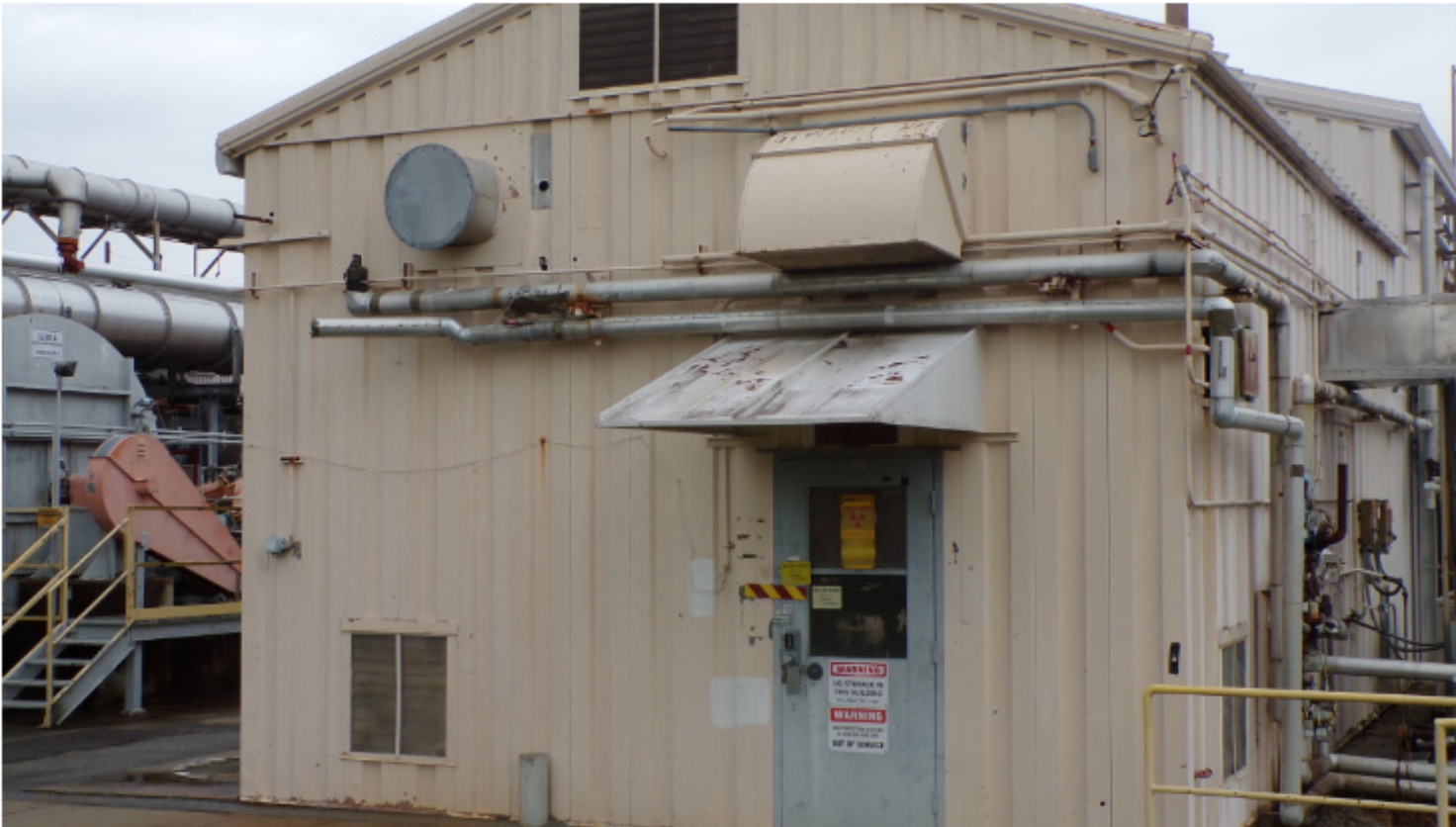
Figure 4. Ground View of Building 236-H Showing Utility Isolations
