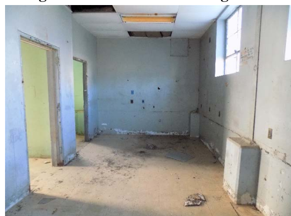
Figure 2D – Interior West Side
