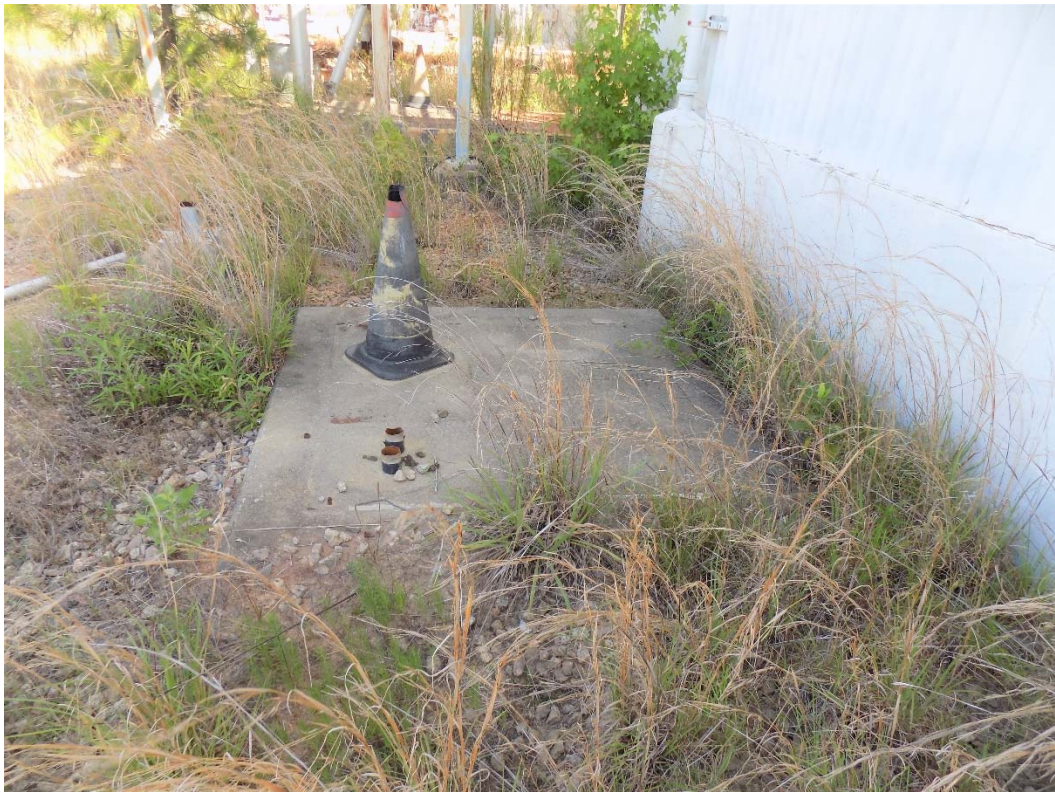
Figure 4F: Dry-type Transformer W4A - Concrete Pad Looking North
