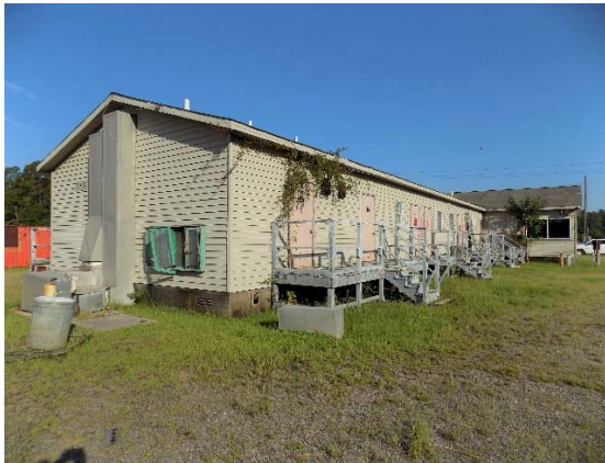
Figure 3A – Exterior Looking Northwest
