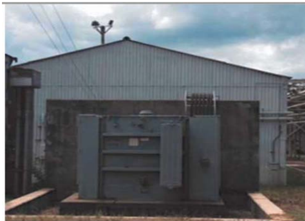
Figure 5A: Former Transformer AT1W
