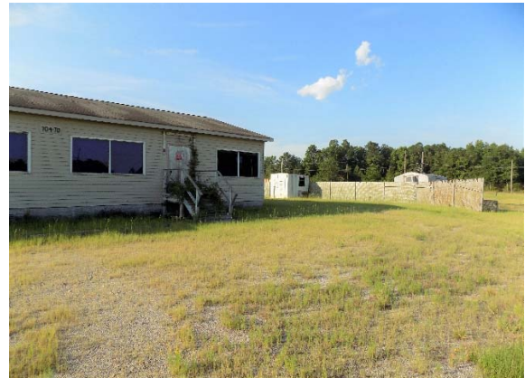
Figure 3B – Exterior Looking Southwest
