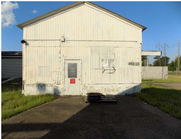
Figure 2A – Exterior Looking West
