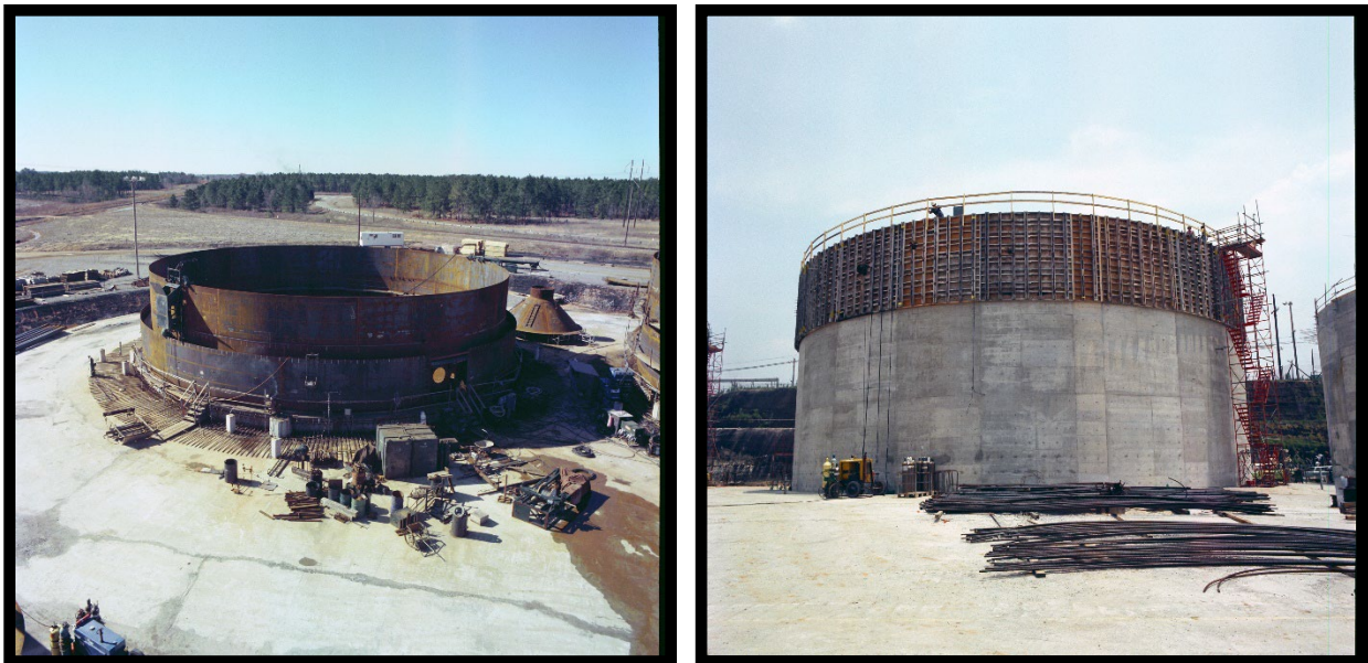
Figure 3.4-1: Typical Construction of Type III/IIIA Tanks
