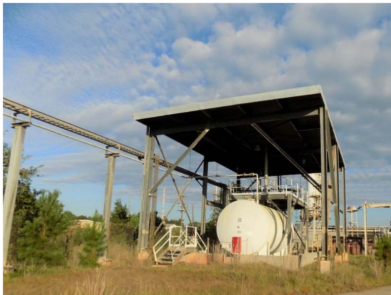
Figure 1. Building 454-D, D-Area Diesel Fuel Tank
