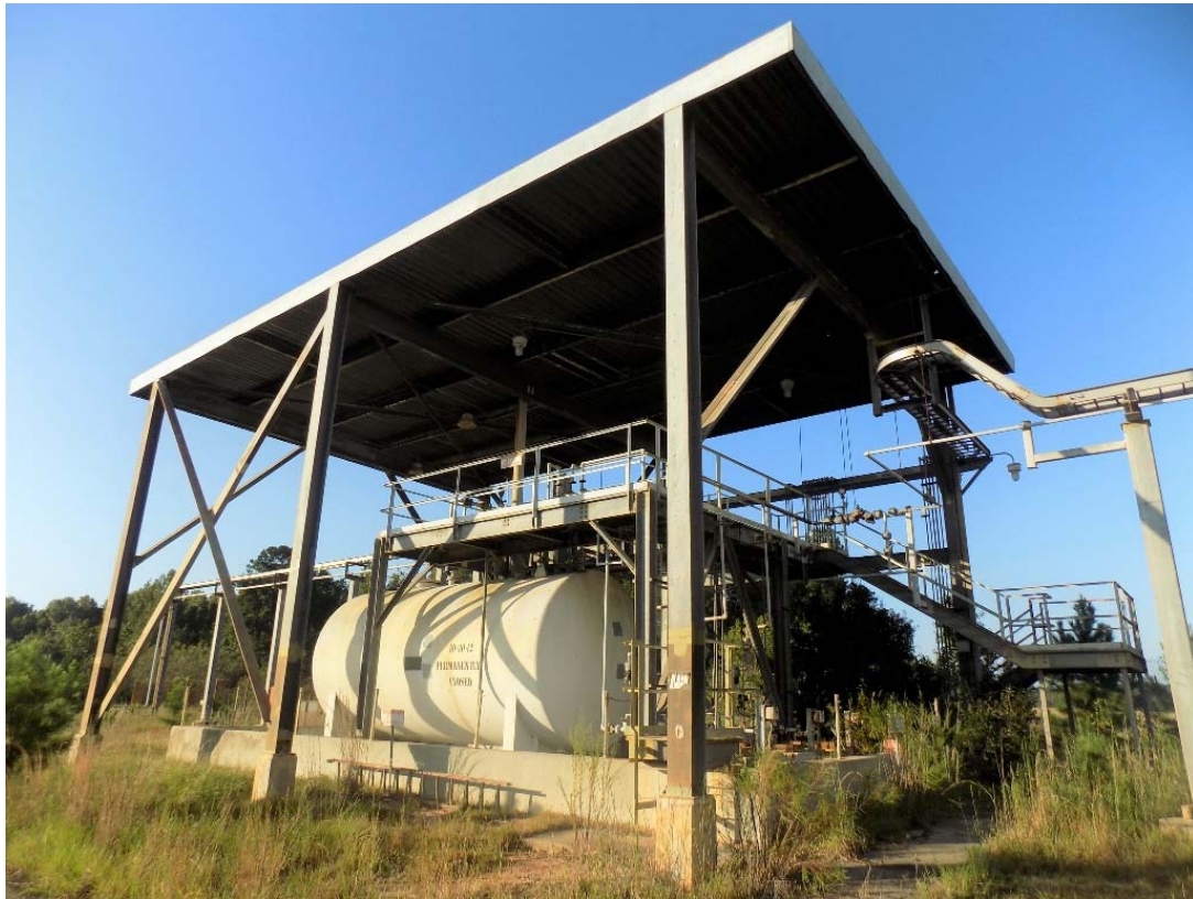
Figure 2. Building 454-D, D-Area Diesel Fuel Tank
