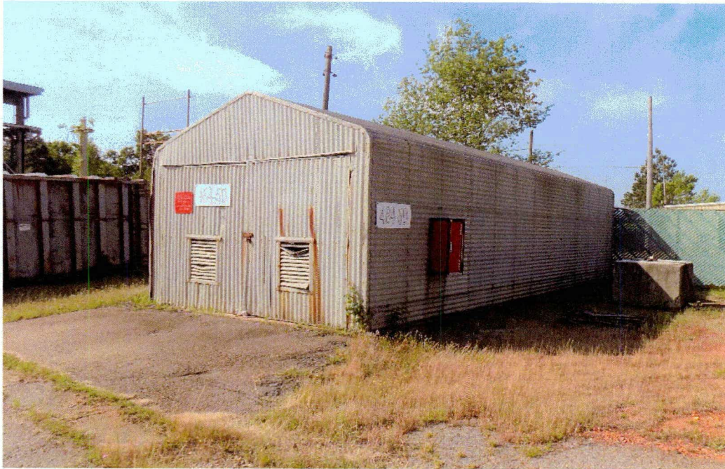
Figure 1. Building 484-5D Powerhouse Storage Building
