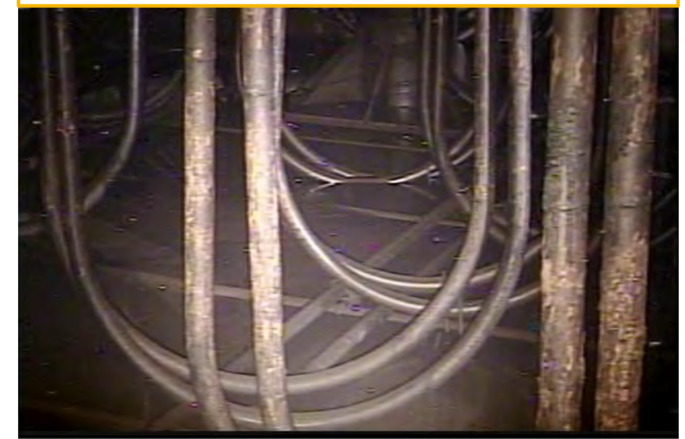
Center Riser to East
