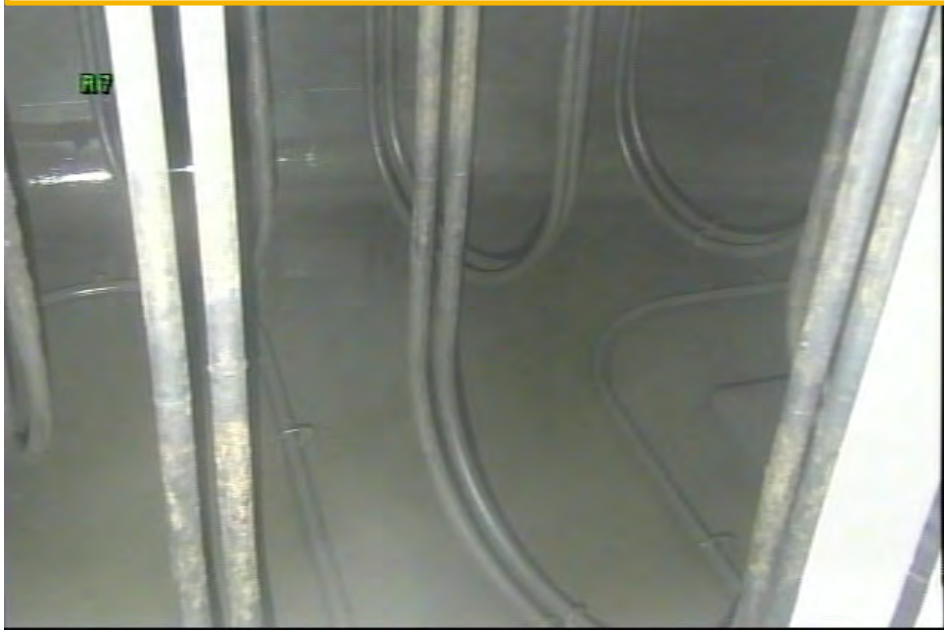
Riser 7 to Southern Wall
