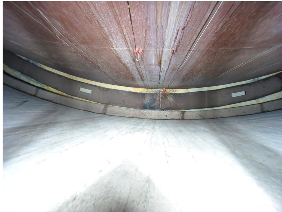
West Riser Before/After
