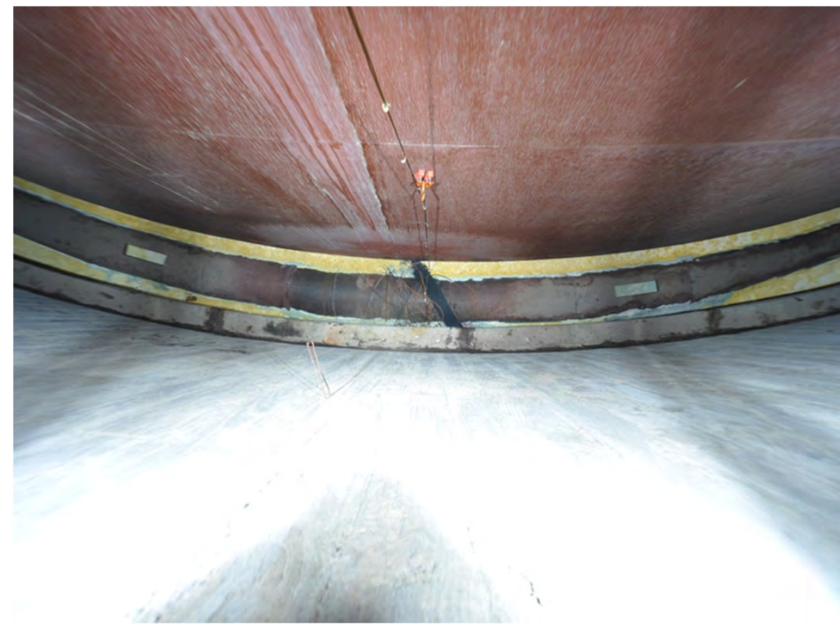
South Riser Before/After
