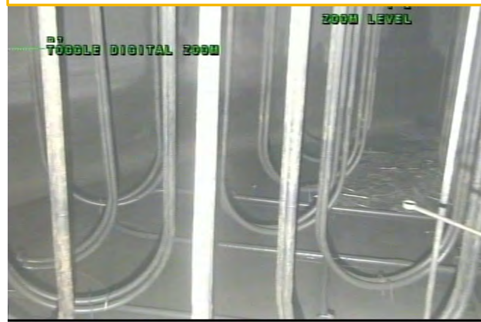
Riser 8 Mound from Riser 7
