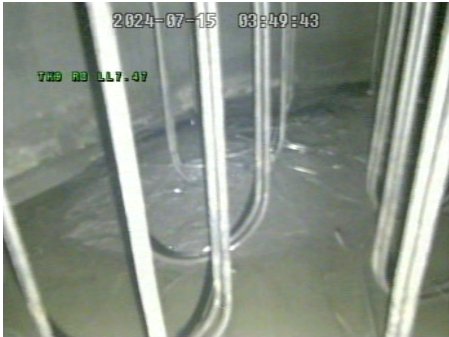
Mound Behind Riser 8 to Valve House
