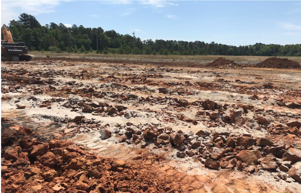
Photo 3. Amendment Spread over Decompacted Soils
