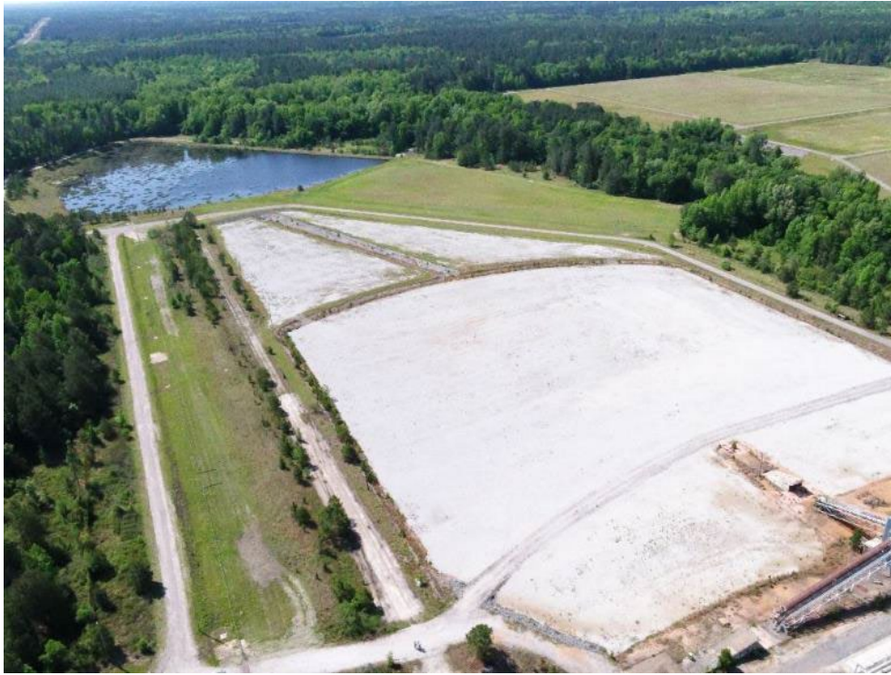
Photo 8. Stabilized Coal Yard with Gravel Vehicle Access Road (Pictured from above.)
