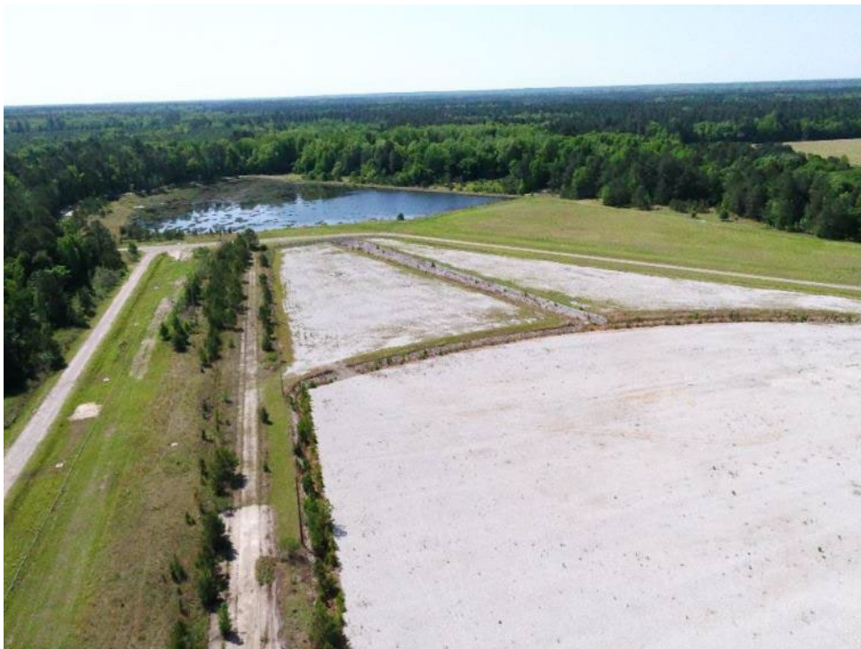
Photo 11. 484-17D DCSA Southern Portion
