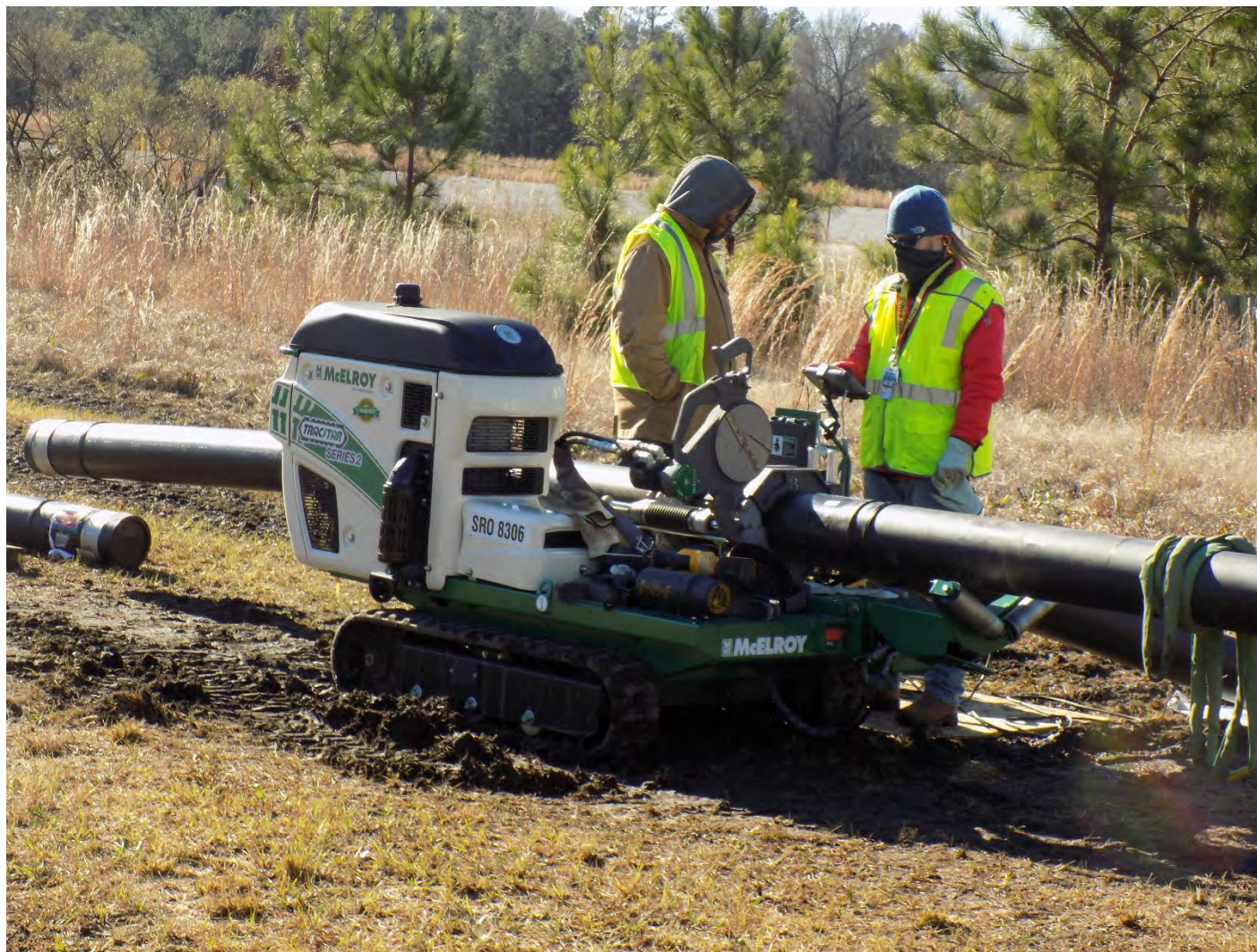
Figure 15. D-Area Treatability Study Pipeline Installation
