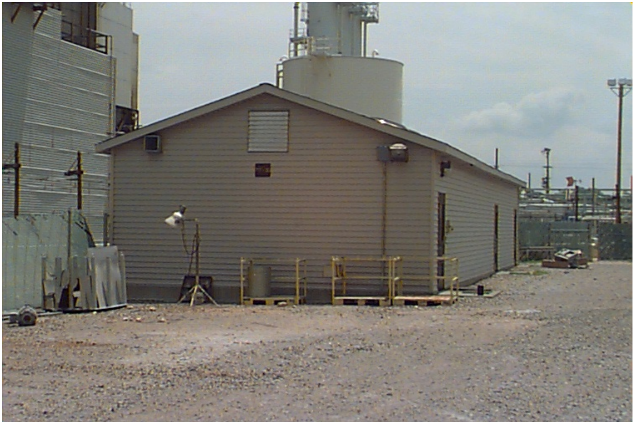
Figure 1. Building 717-3D, D-Area Storage Facility
