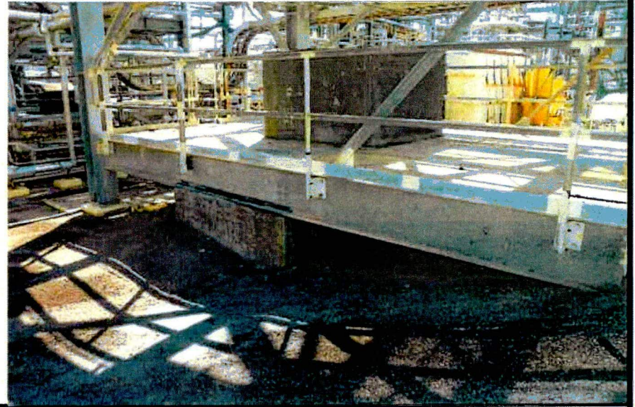
Tank 19, East Riser
