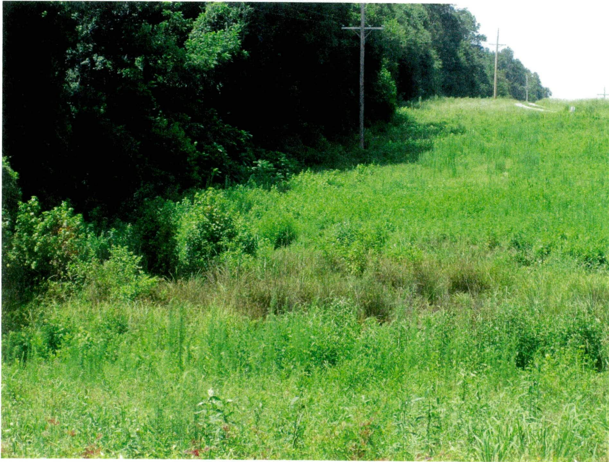
Photograph 1. Typical small wetland crossing of a 13.8-kV distribution line; the length of the crossing is approximately 100 feet.
