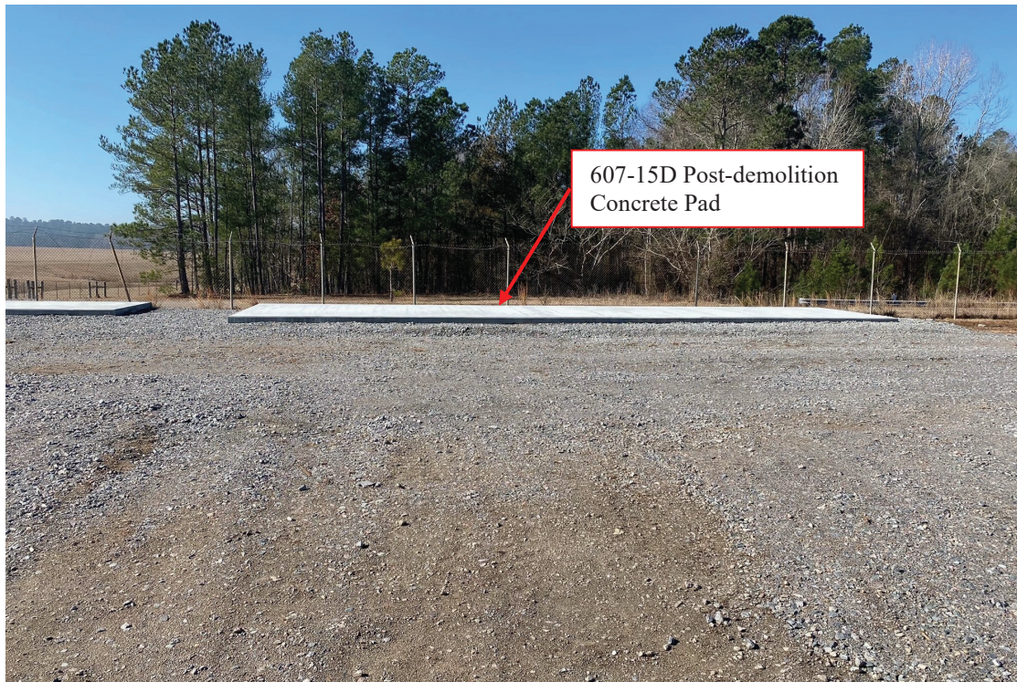
Figure A-10. 607-7D and 607-15D Blowers (Looking West) After Decommissioning
