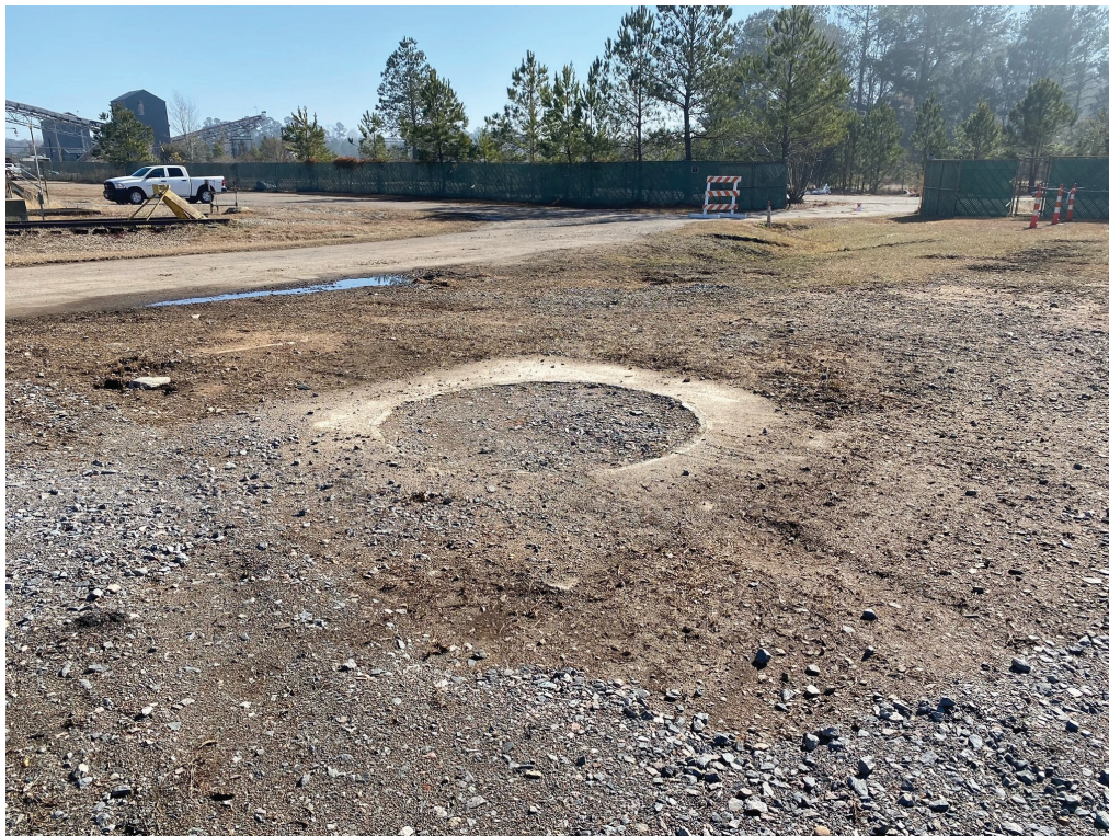
Figure A-8. 607-12D (Looking Southwest) After Decommissioning
