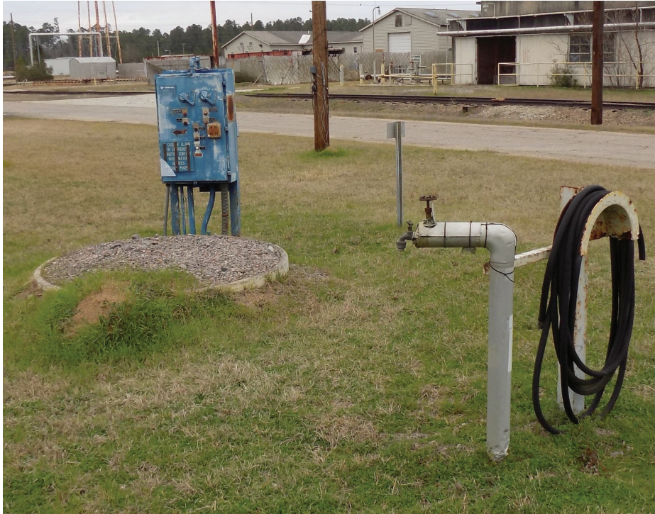
Figure A-11. 607-2D (Looking Southwest) Before Decommissioning
