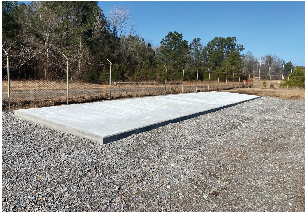
Figure A-4. 607-15D (Looking Southwest) After Decommissioning
