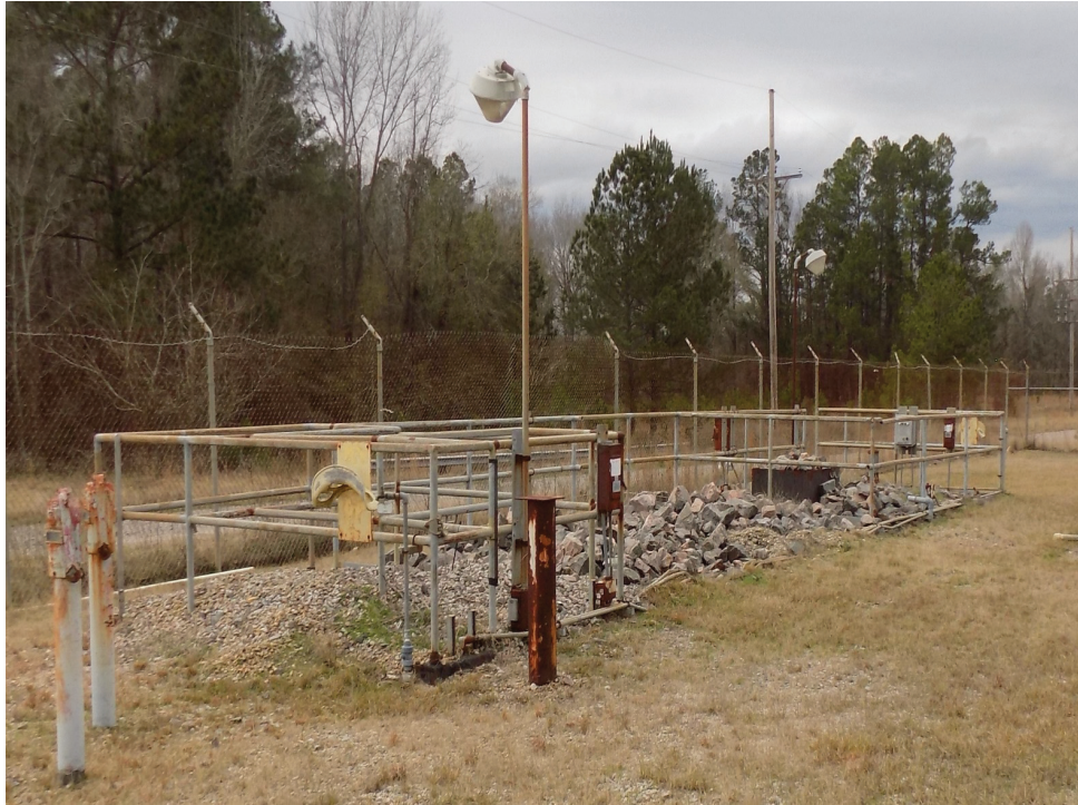
Figure A-3. 607-15D (Looking Northwest) Before Decommissioning
