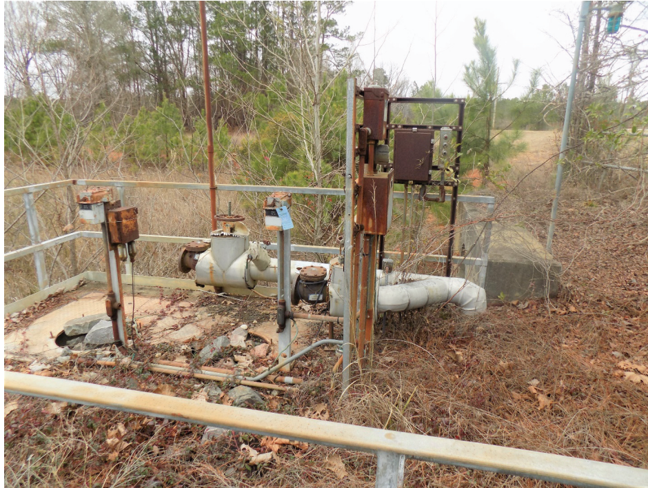
Figure A-13. 483-6D Surge Basin (Looking Northwest) Before Decommissioning
