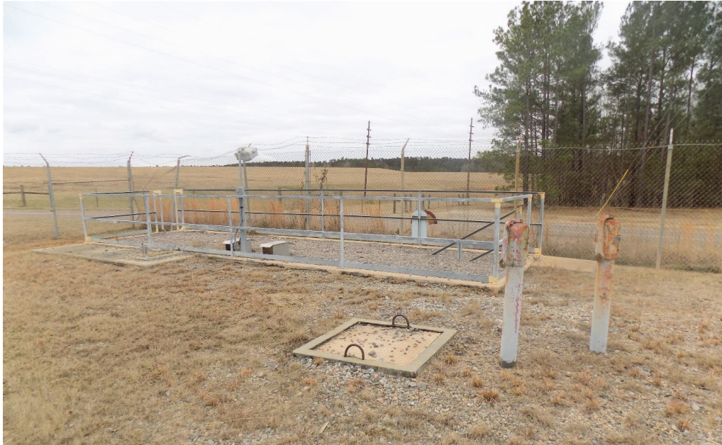
Figure A-5. Disinfestation Pit (Looking Southwest) Before Decommissioning
