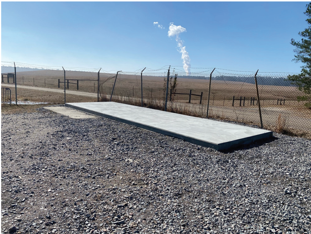
Figure A-6. Disinfestation Pit (Looking Southwest) After Decommissioning
