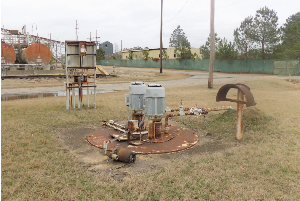
Figure A-7. 607-12D (Looking Southwest) Before Decommissioning
