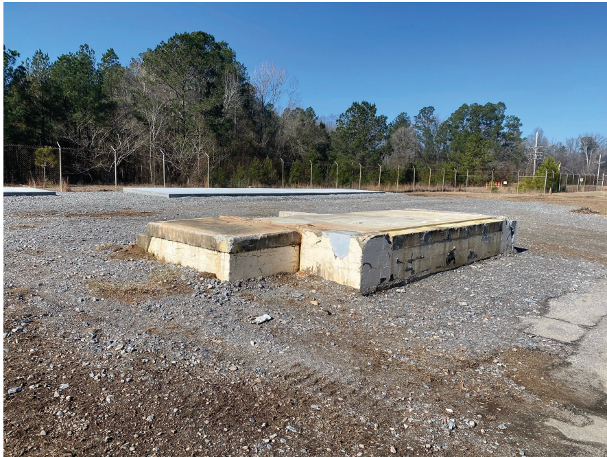
Figure A-2. 607-14D (Looking Northwest) After Decommissioning
