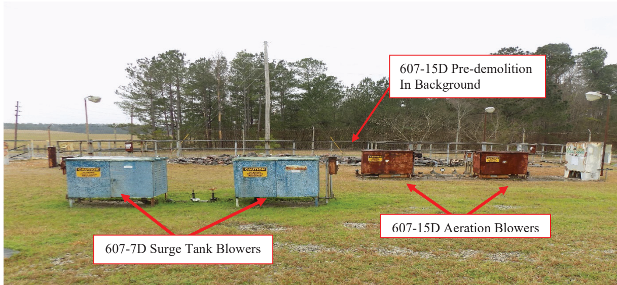
Figure A-9. 607-7D and 607-15D Blowers (Looking West) Before Decommissioning
