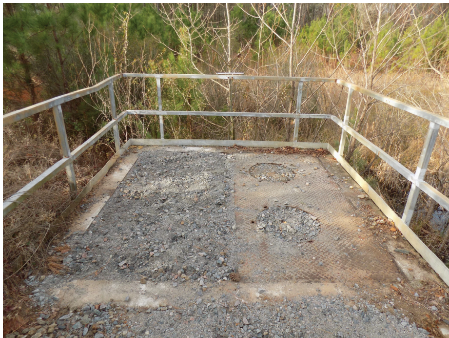
Figure A-14. 483-6D Surge Basin (Looking West) After Decommissioning
