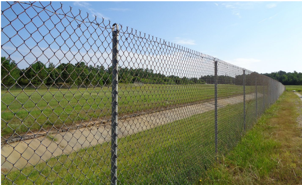
Figure G-4. Current On-Unit Photographs of the Cover System of the HHWMF OU (2020)
