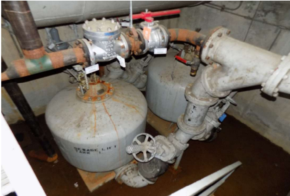
Figure 3: Interior Below Grade Tanks of 607-3F (Before)
