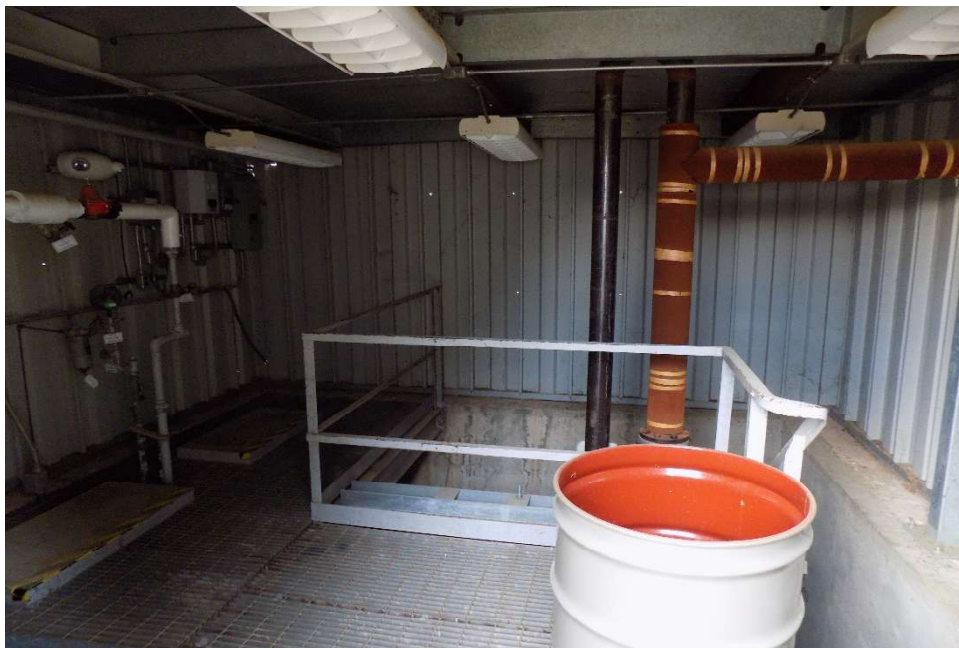
Figure 2: 607-3F Grade Level Area (Before)
