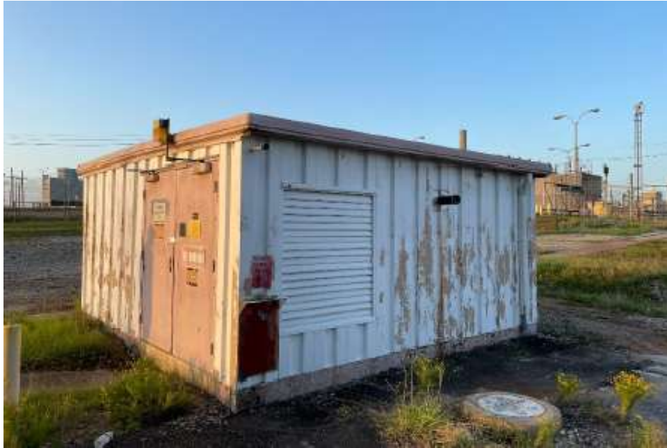
Figure 1: 607-3F Metal Structure (Before)
