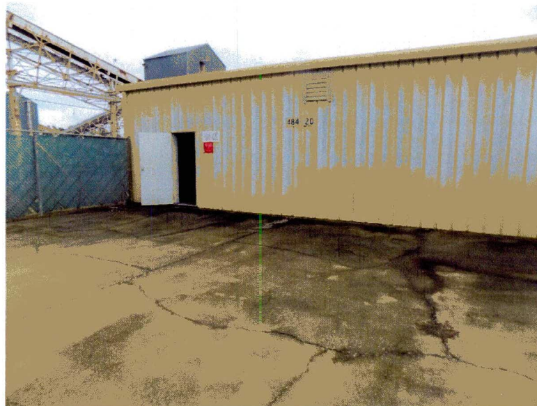
Figure 7. Ground View of 484-12D Laydown Yard
