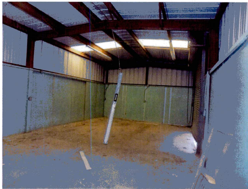
Figure 8. Interior View of Building 484-7D
