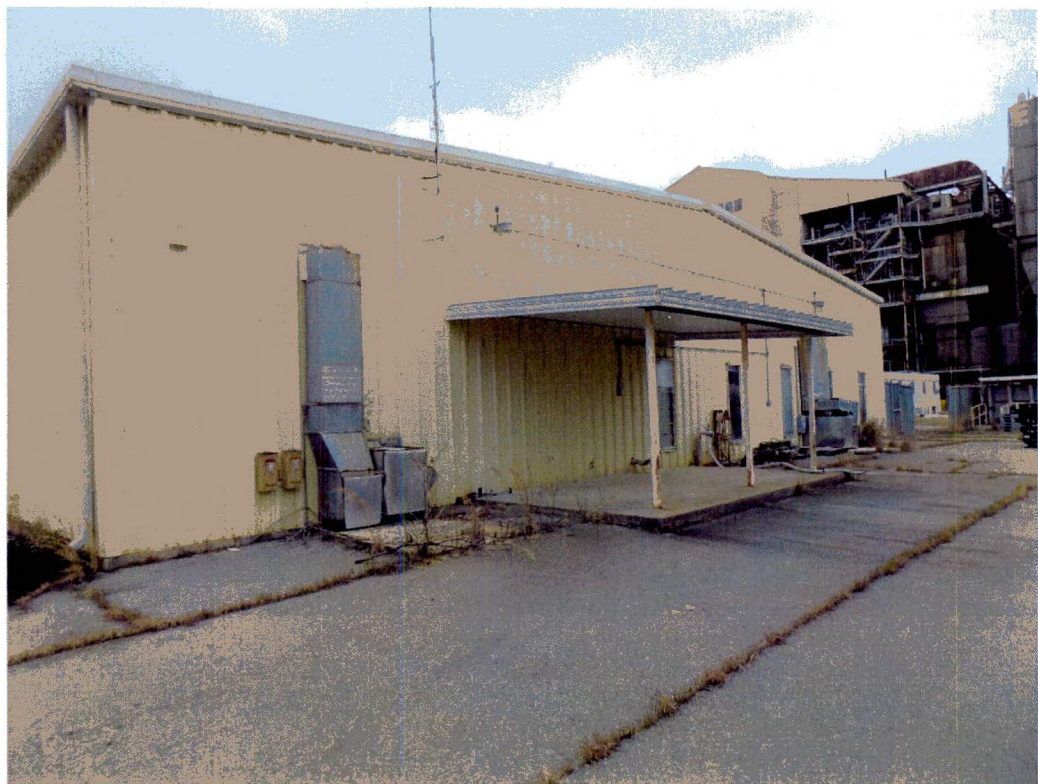
Figure 3. Photograph of Small Covered Area on East Side of Building 484-4D
