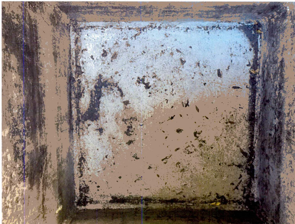
454-D Sump Interior (March 2020)
