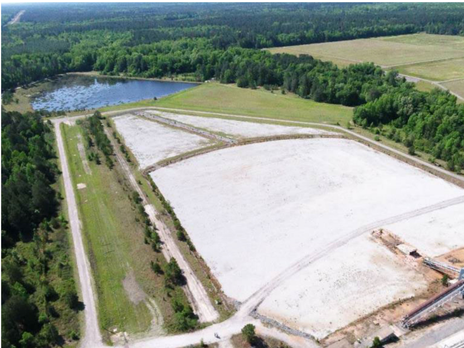
Figure 23. Photograph After Completion of the Soil Neutralization at the 484-17D DCSA
