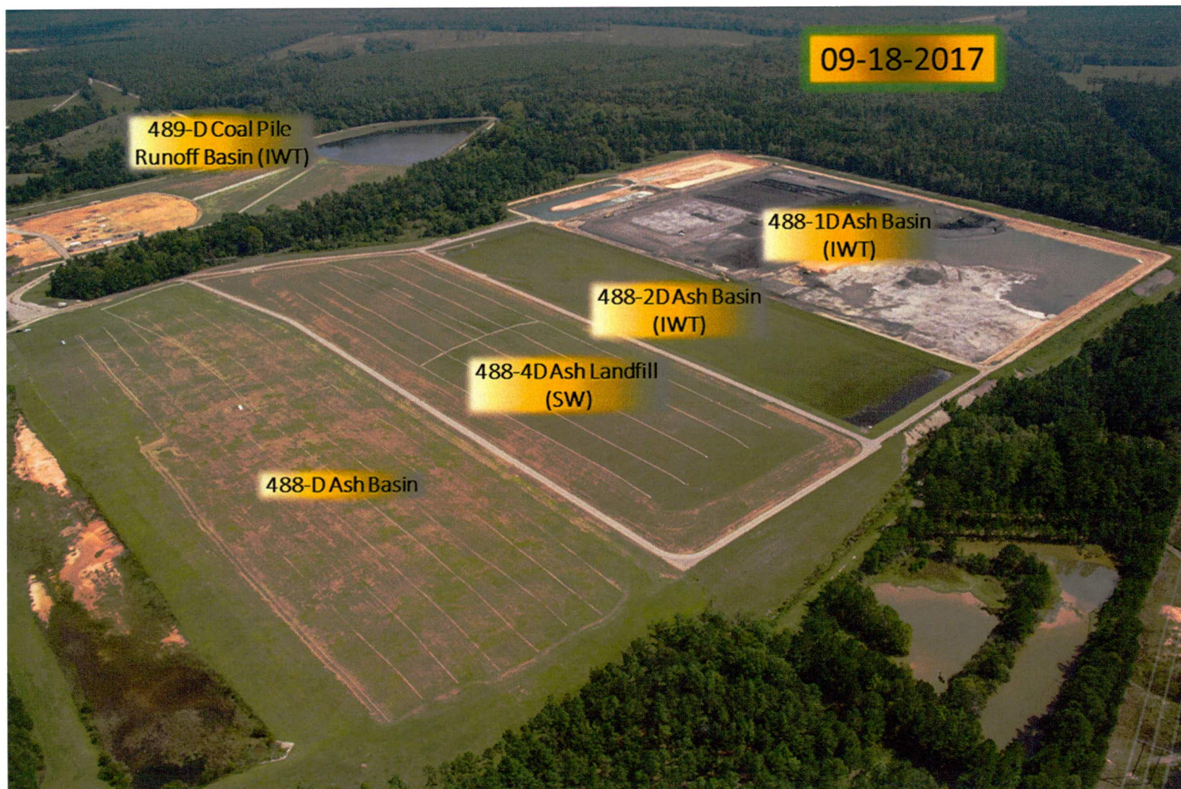
Figure 6. 488-2D Ash Basin and 488-4D Ash Landfill (Construction Complete, dated 9/18/17)
