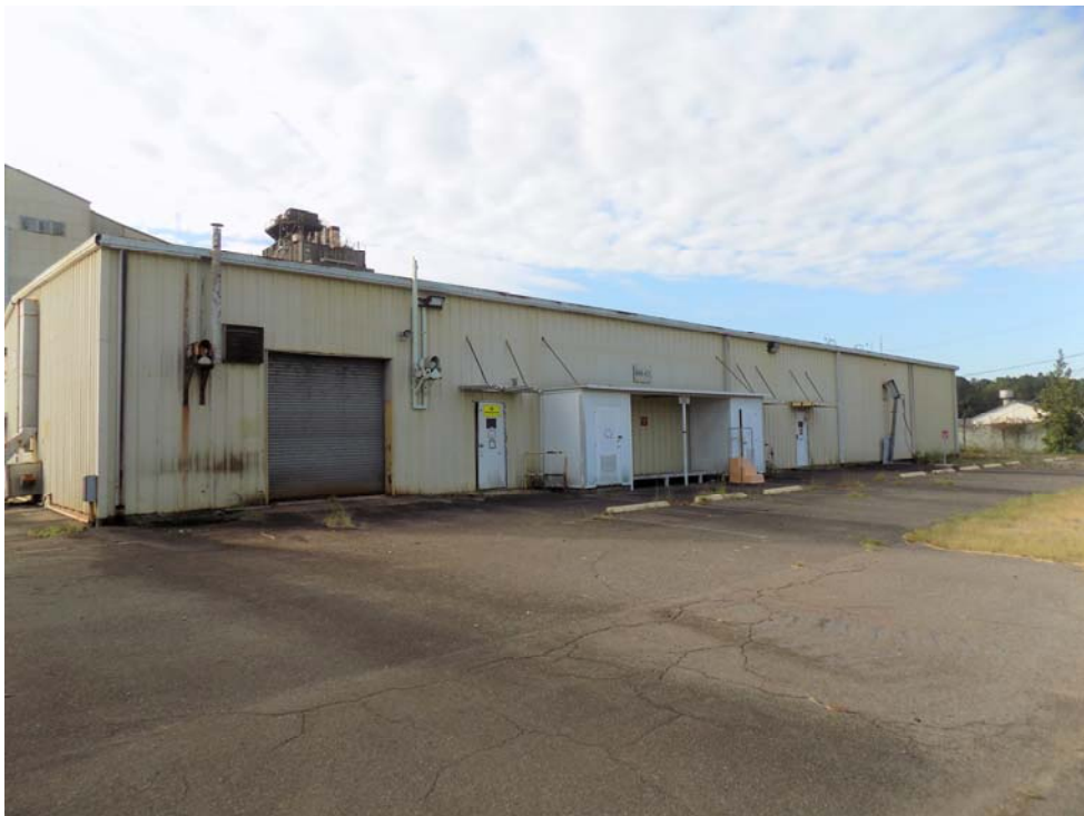
Figure 2. Building 484-4D Maintenance Facility
