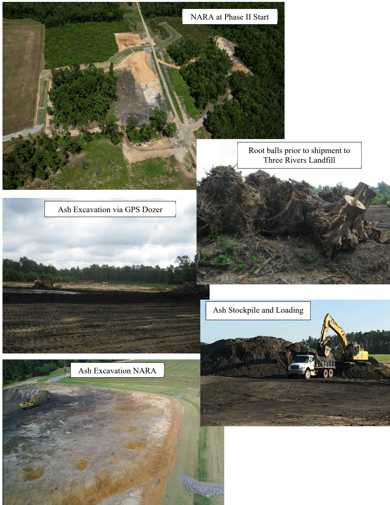
Figure 12. NARA Phase II- Clearing and Grubbing and Excavation Activities
