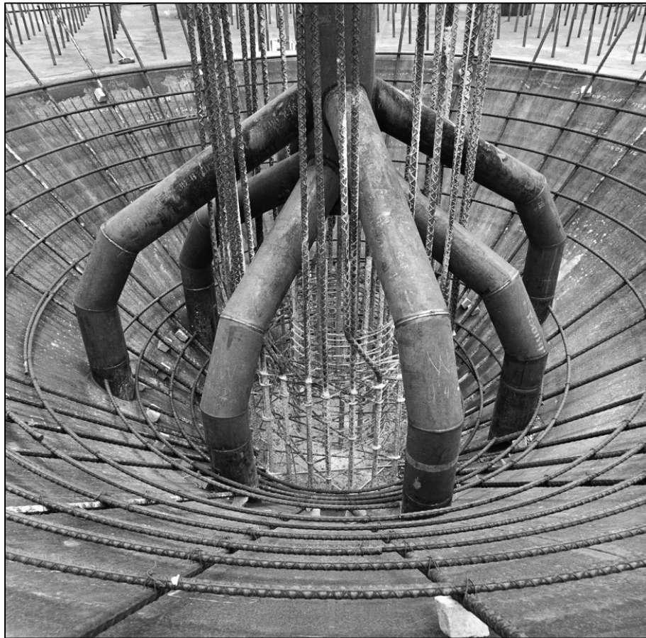
Figure 2.2-9: Type III/IIIA Tank Central Column and Vent Ductwork Construction Photo
