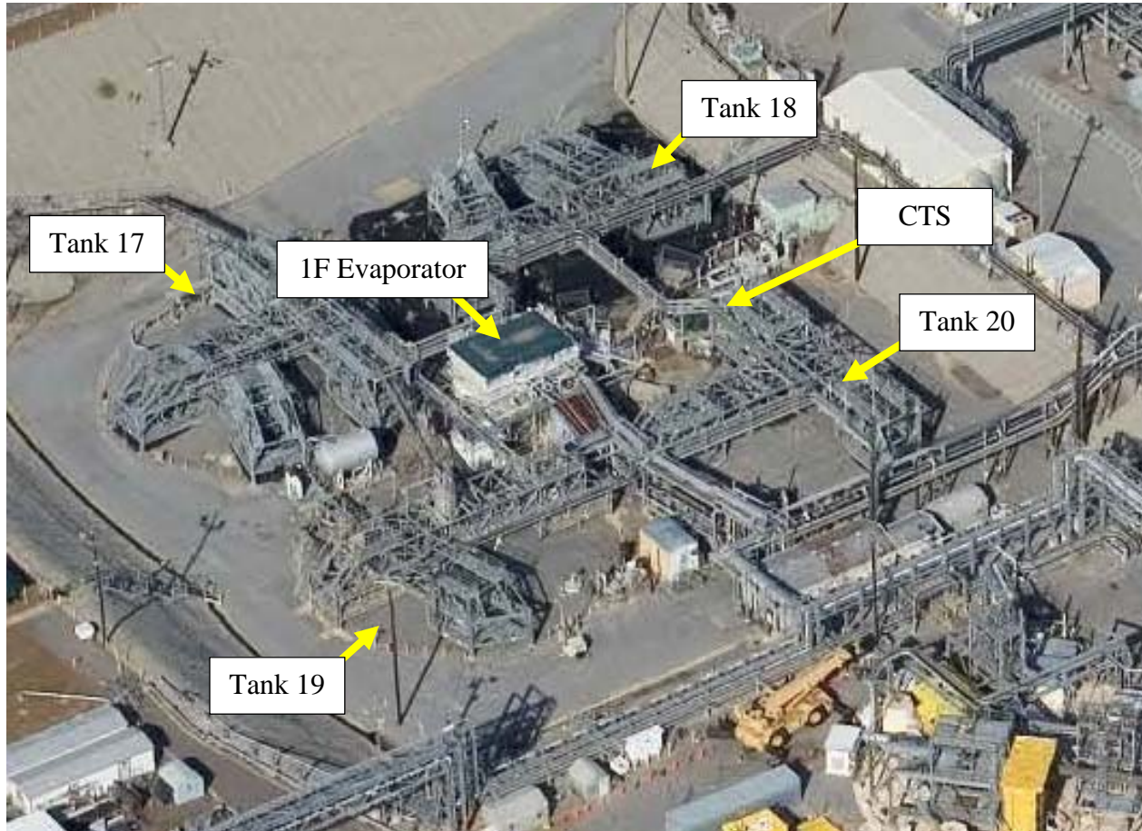
Figure 4.2-1: Tanks 17 and 19, 1F Evaporator, and CTS
