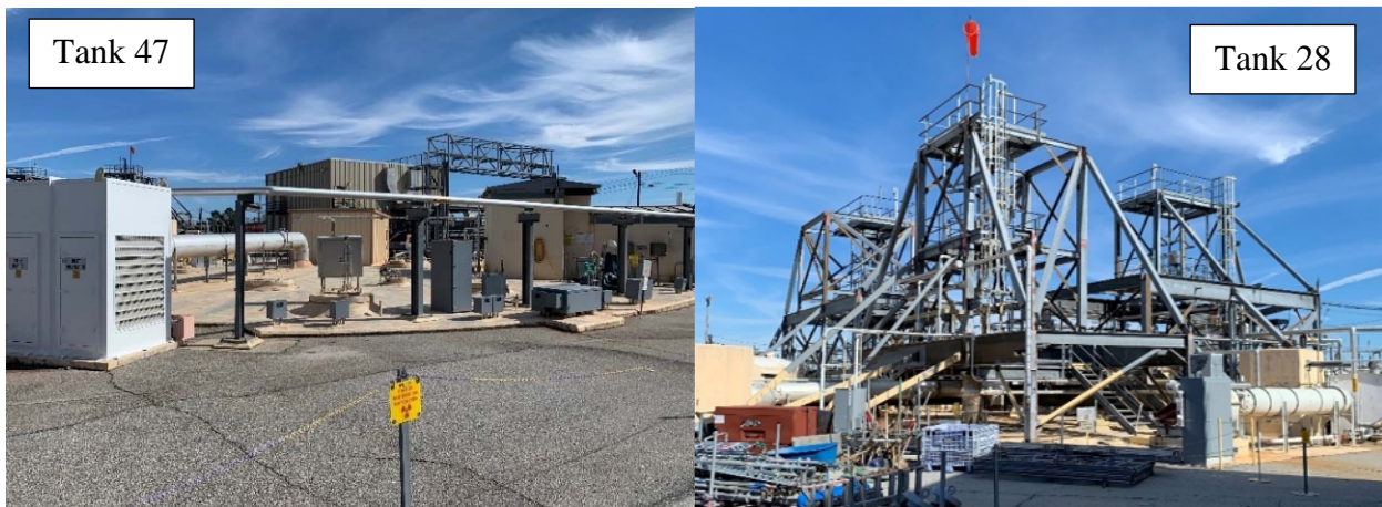
Figure 4.4-6: Tank 47 and Tank 28
