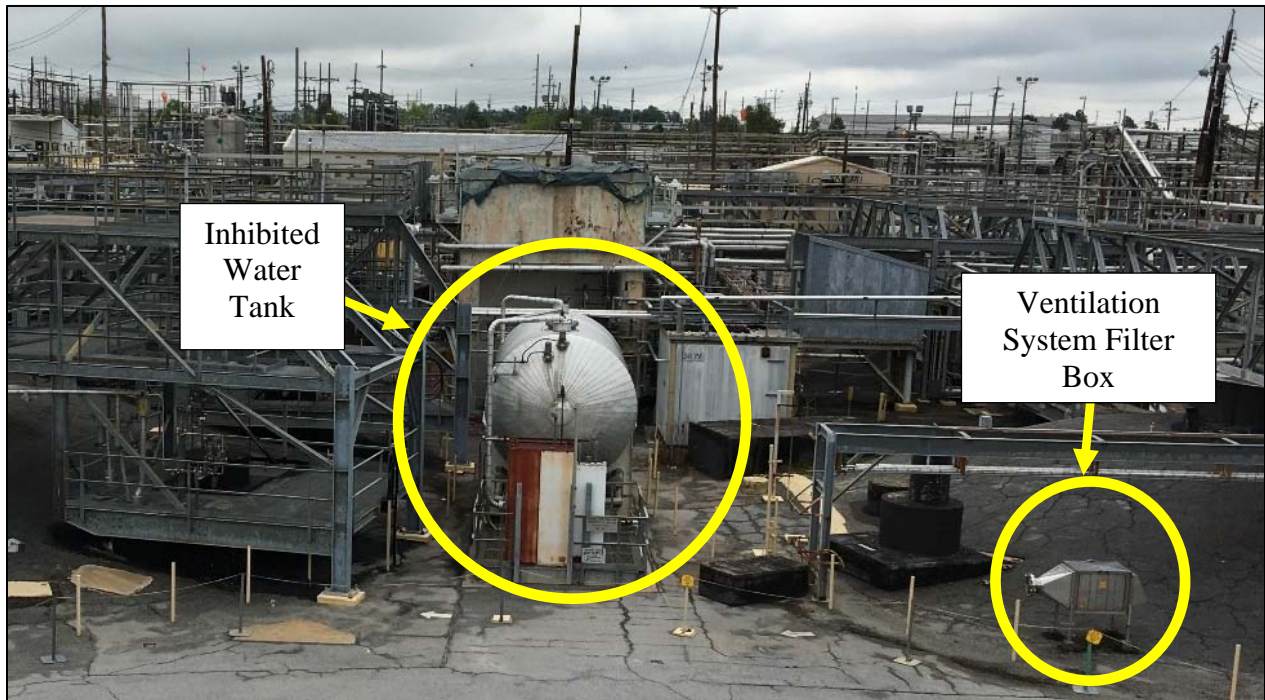
Figure 2.4-1: View of Tank 17, Tank 19 and the 1F Evaporator
