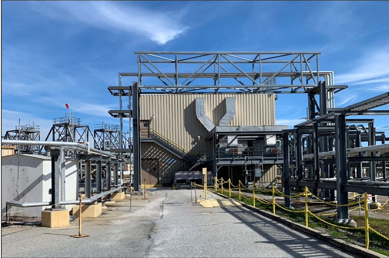
Figure 4.4-7: 241-18F Control Room
