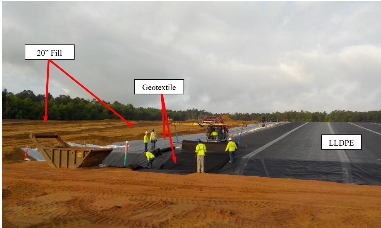
Photo 83. Geotextile Placement over the LLDPE Geomembrane (1)
