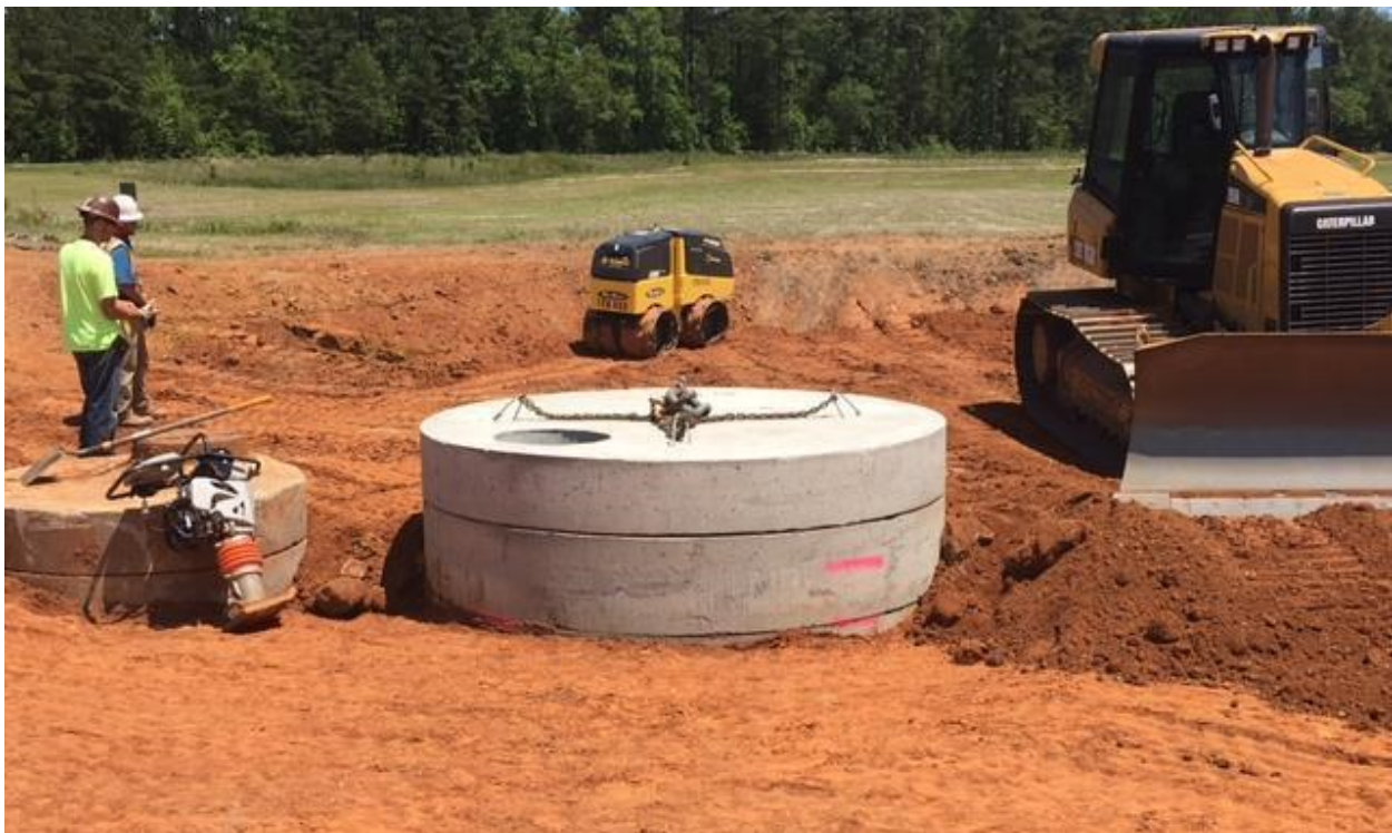
Photo 42. 489-D CPRB Backfilling in Progress
