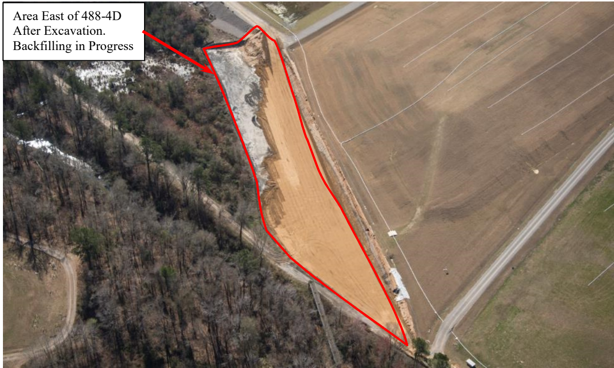
Photo 27. Area East of 488-4D Ash Landfill (February 2017)
