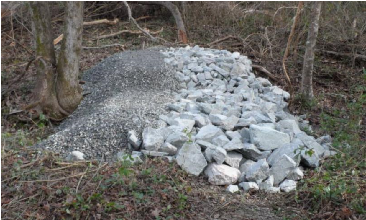
Photo 22. Typical Rock Check Dam
