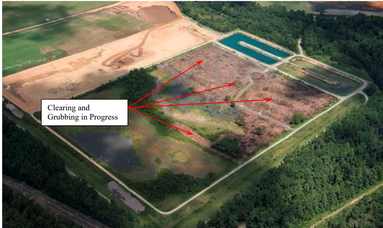
Photo 45. 488-1D Ash Basin (August 2016)
