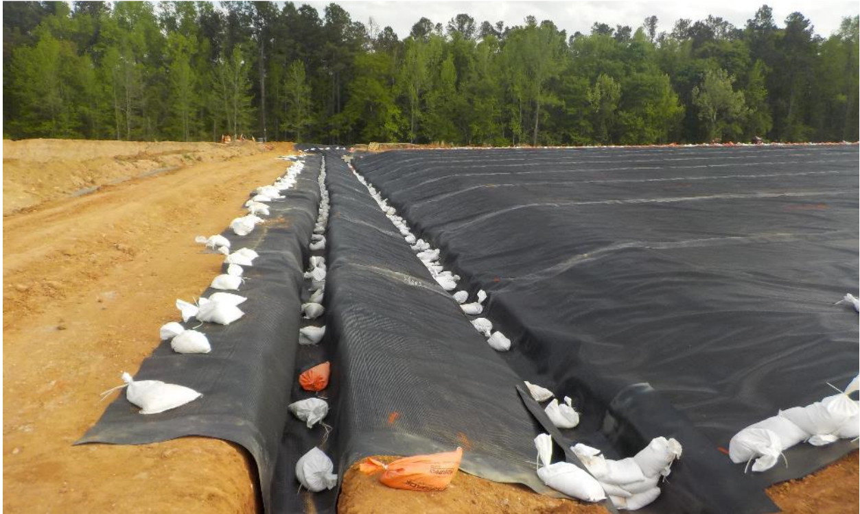
Photo 73. LLDPE Placement at Anchor Trench and Subsurface Drainage Ditch
