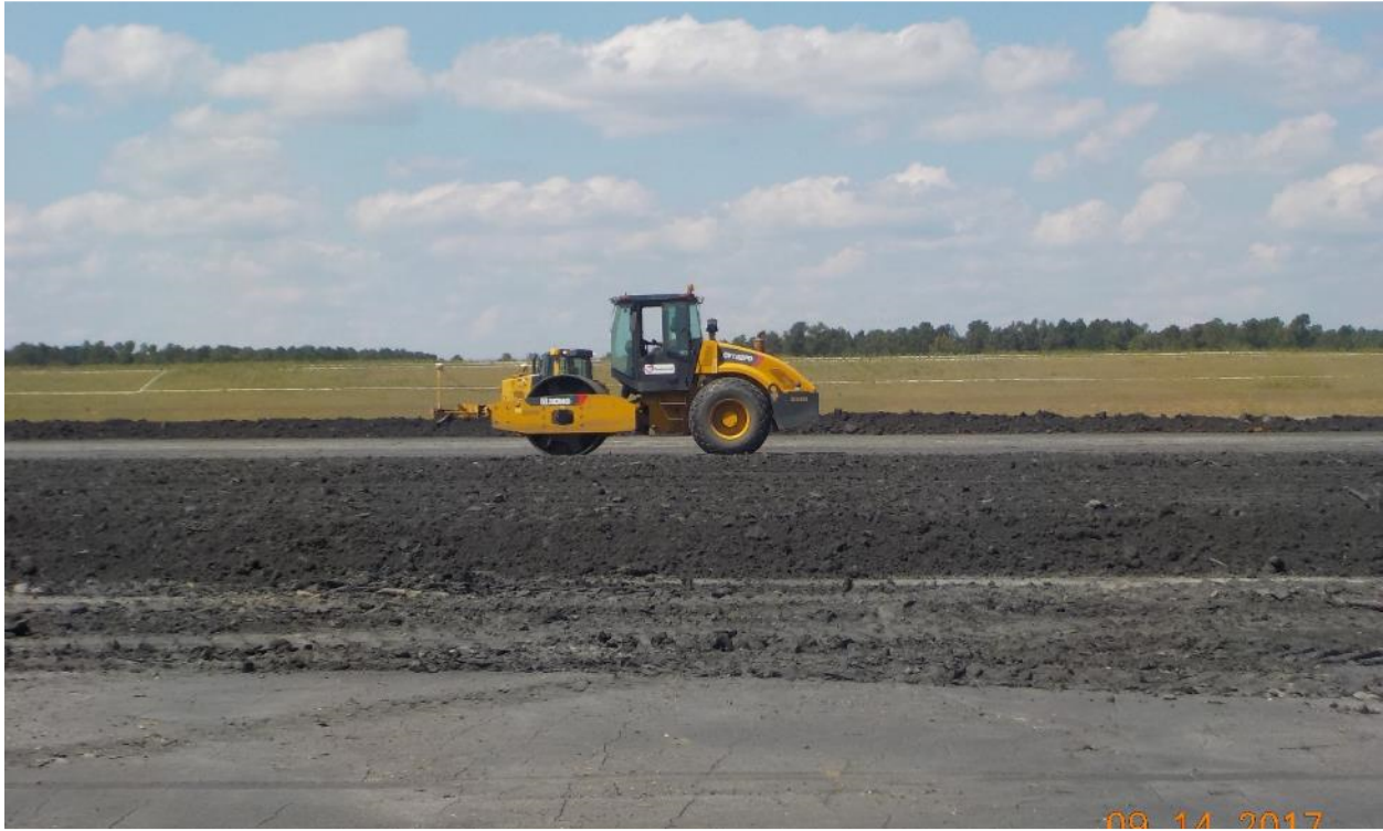
Photo 55. Compaction of Ash 488-1D Ash Basin (East End)
