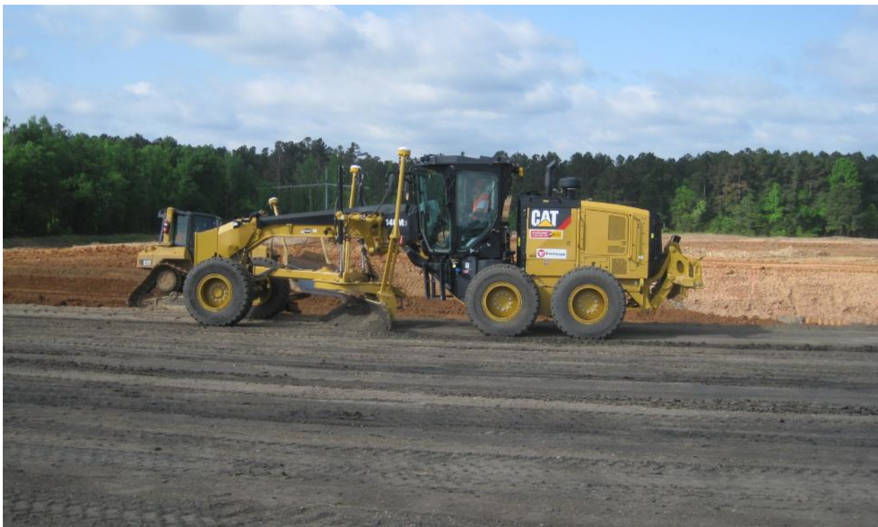
Photo 70. Fine Grading of the Ash Mound Prior to Final Ash Survey
