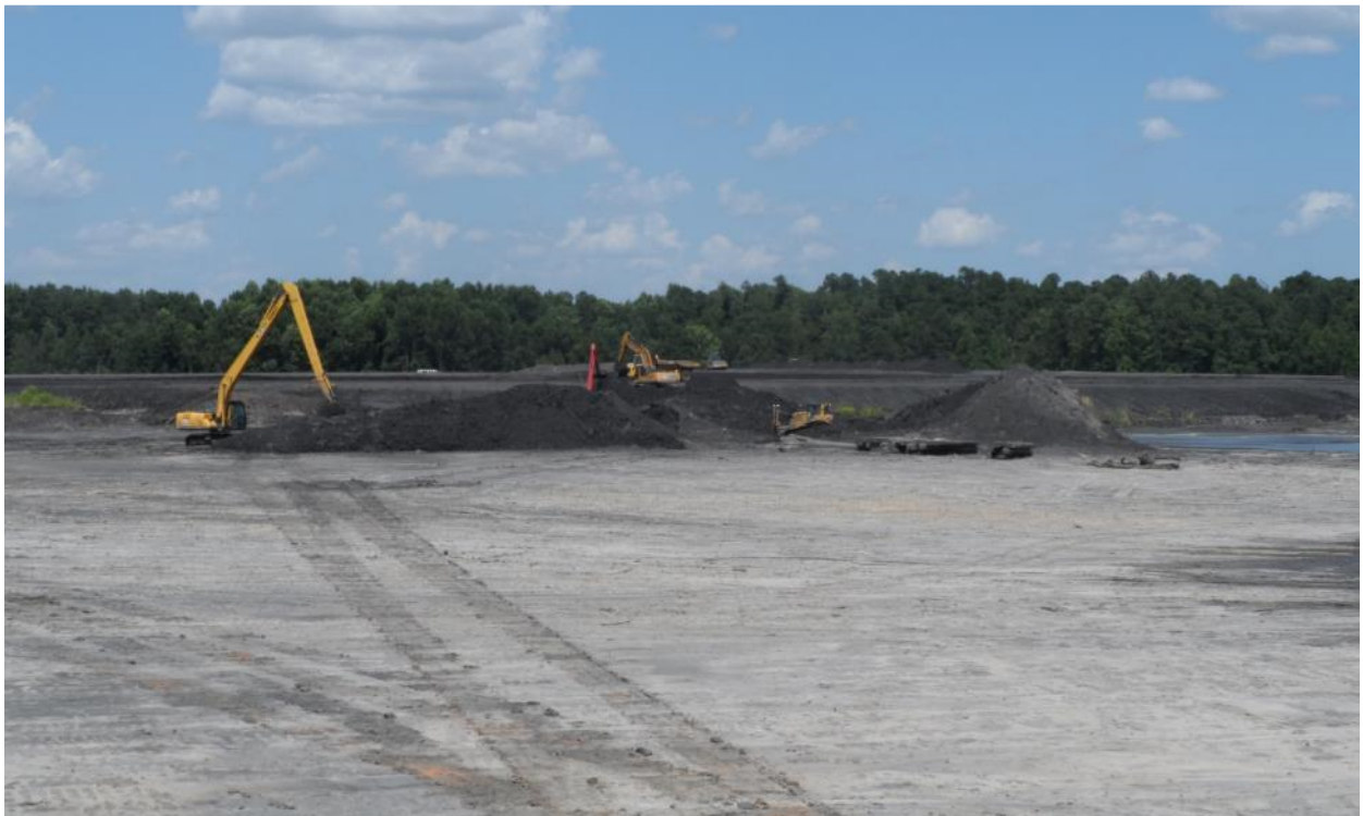
Photo 50. 488-1D Ash Basin West End Bulk Ash Removal
