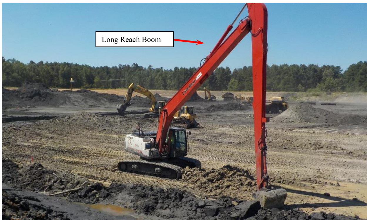
Photo 6. Long Reach Excavator
