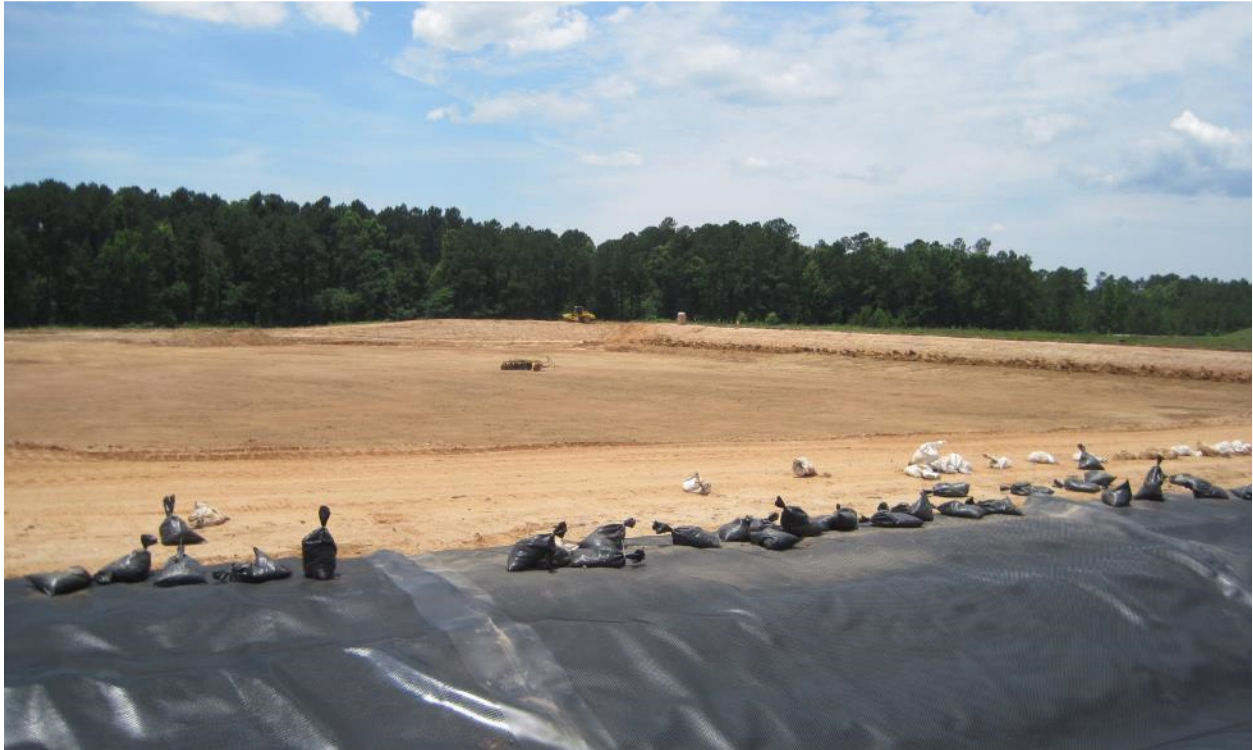
Photo 61. Backfill 488-1D Ash Basin West
