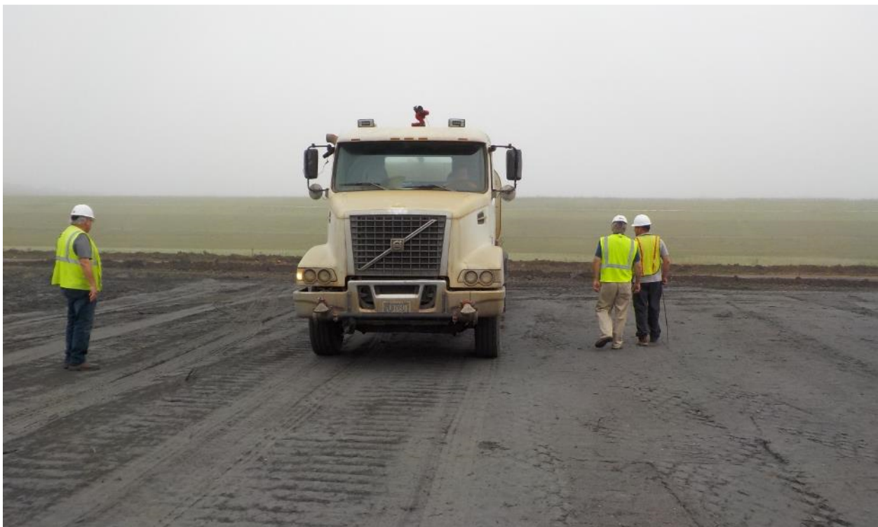
Photo 56. Proof Roll Inspection
