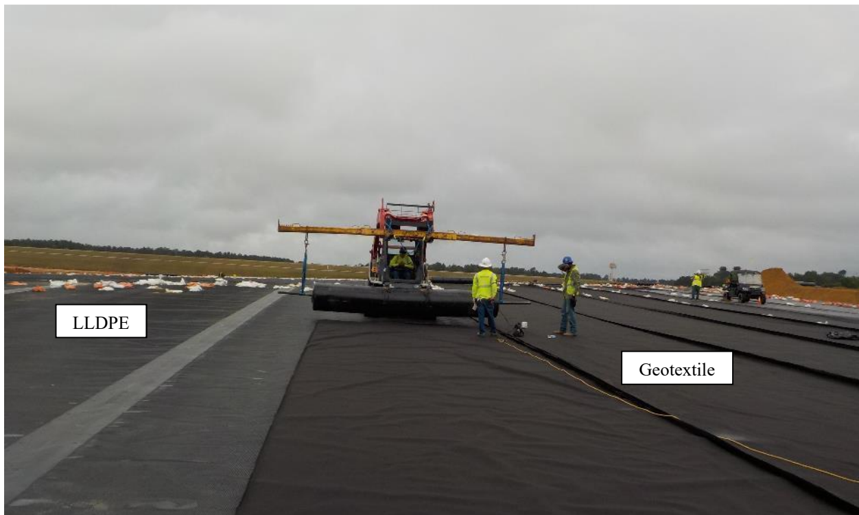
Photo 84. Geotextile Placement over the LLDPE Geomembrane (2)
