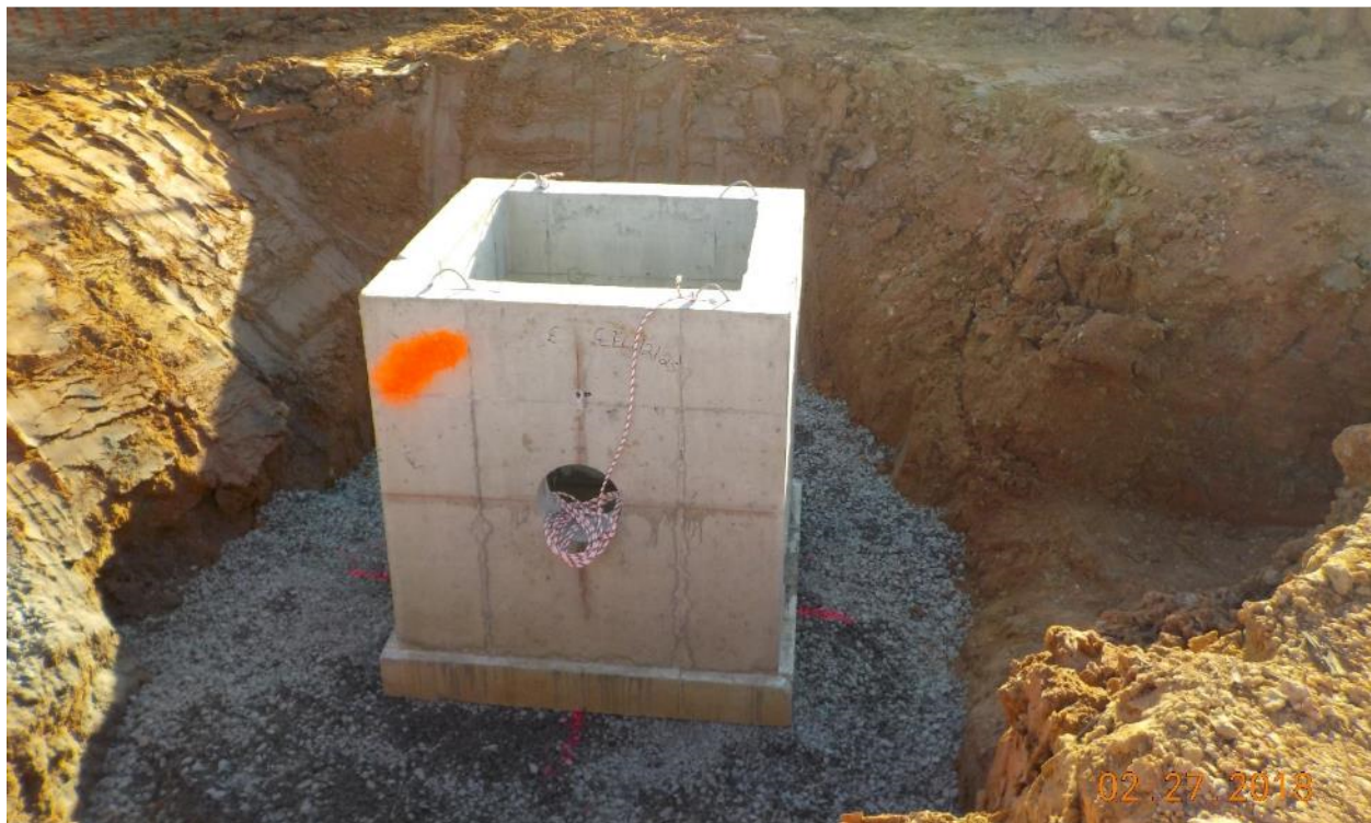
Photo 64. 488-1D Ash Basin Typical Catch Basin Installation
