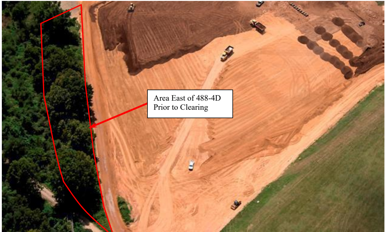
Photo 25. Area East of 488-4D Ash Landfill (August 2016)
