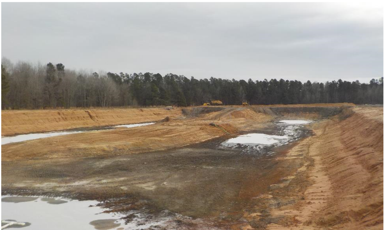
Photo 62. North Inlet Basin Removal of Residual Ash/Soil in Process
