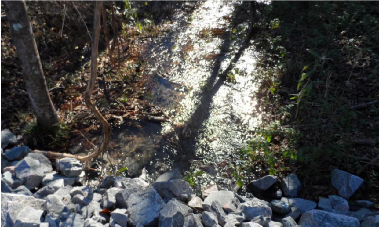
Photo 23. Stormwater Discharge through Check Dam
