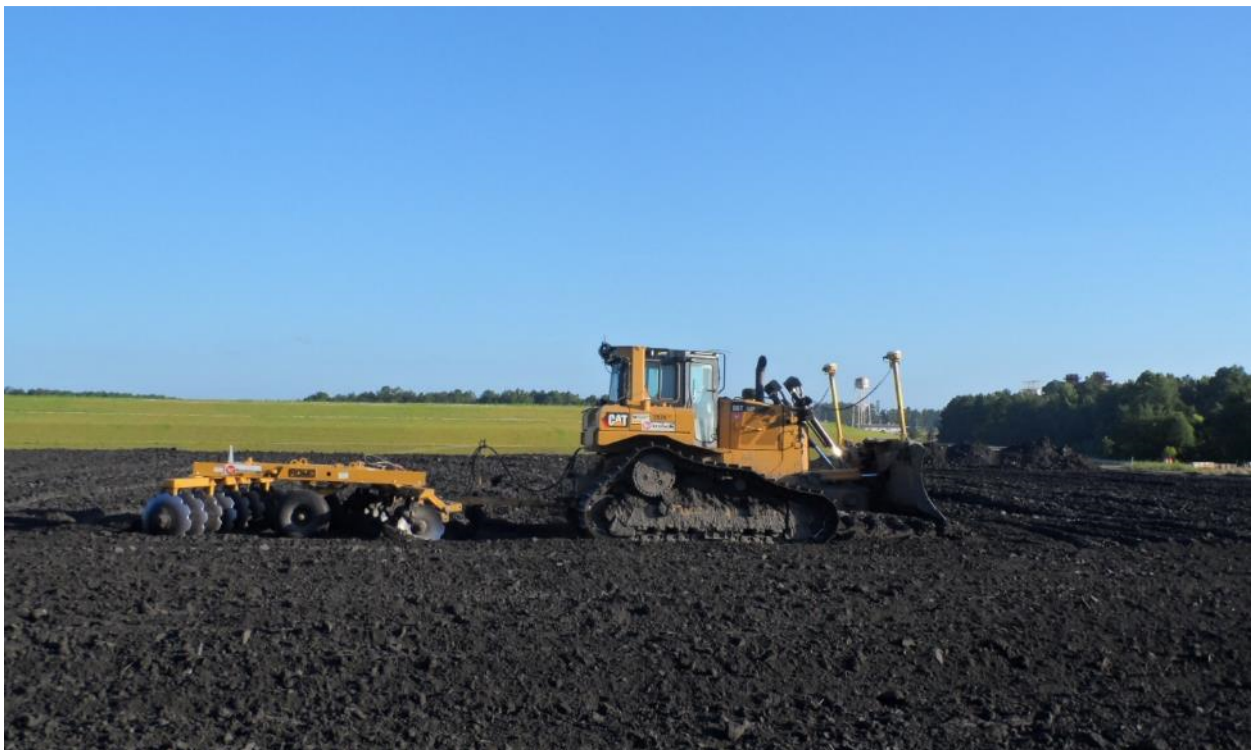
Photo 54. Disking of Ash to Allow for Additional Drying 488-1D Ash Basin (East End)
