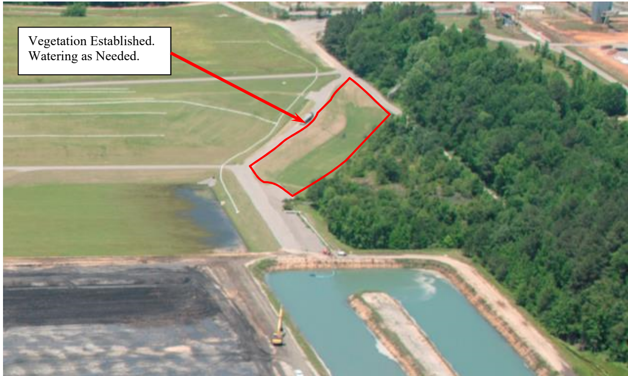
Photo 29. Area East of 488-4D Ash Landfill (April 2017)
