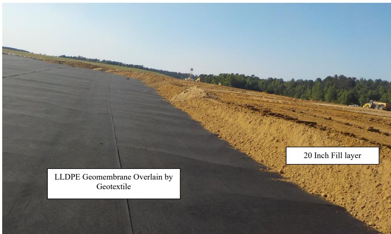
Photo 90. 488-1D Ash Basin East 20 Inch Soil Cover Placement
