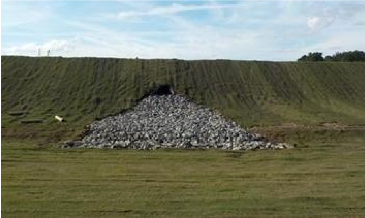
Photo 67. Typical RipRap Apron
