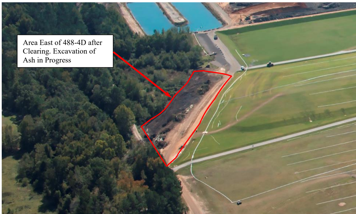
Photo 26. Area East of 488-4D Ash Landfill (October 2016)
