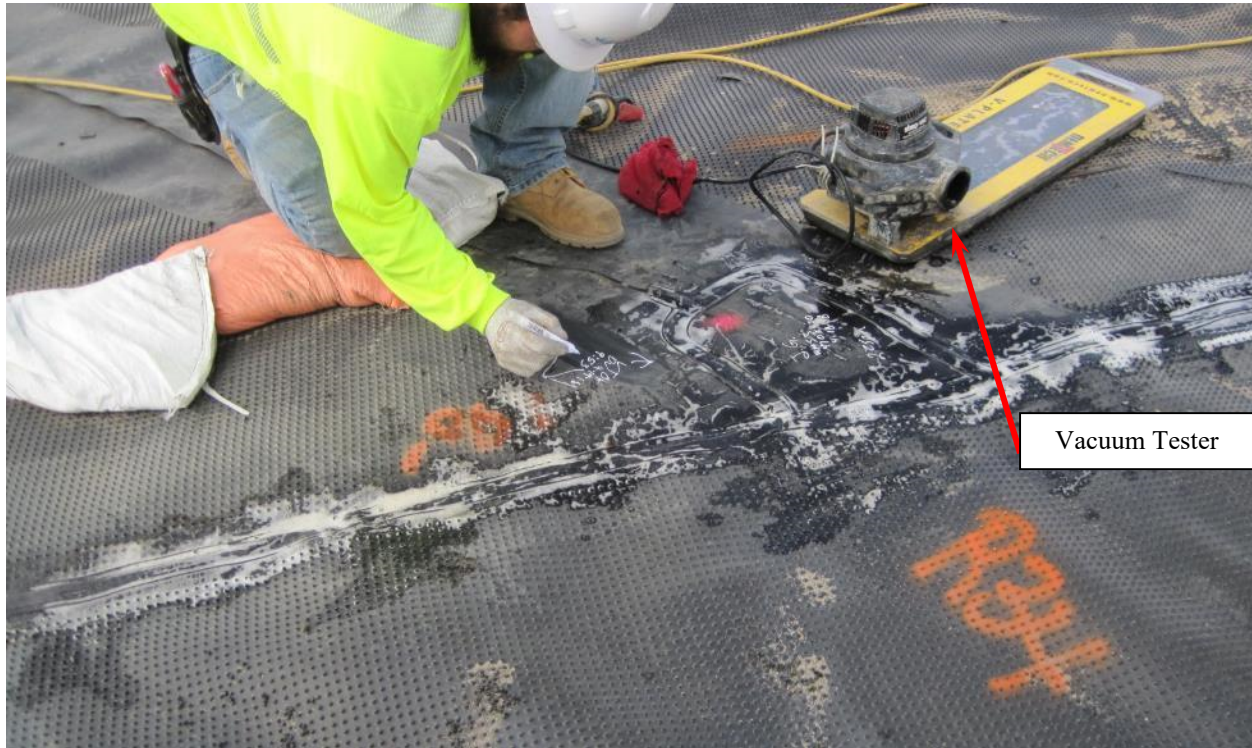
Photo 81. LLDPE Vacuum Testing of Extrusion Welds (Non-Destructive)
