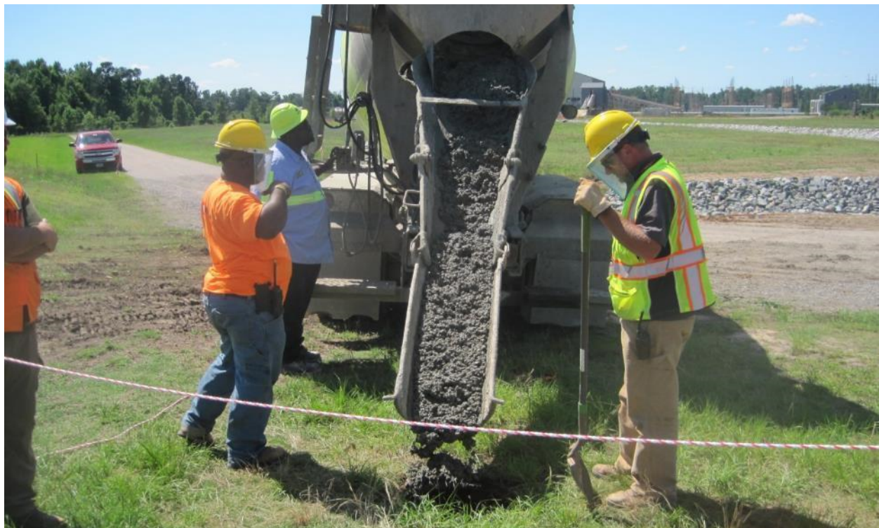
Photo 36. 489-D CPRB Plugging of Upgradient Manholes
