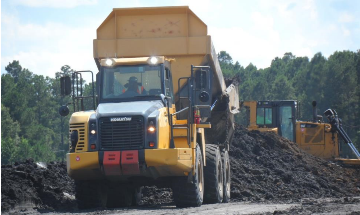
Photo 53. Placement of Ash on East End of 488-1D Ash Basin
