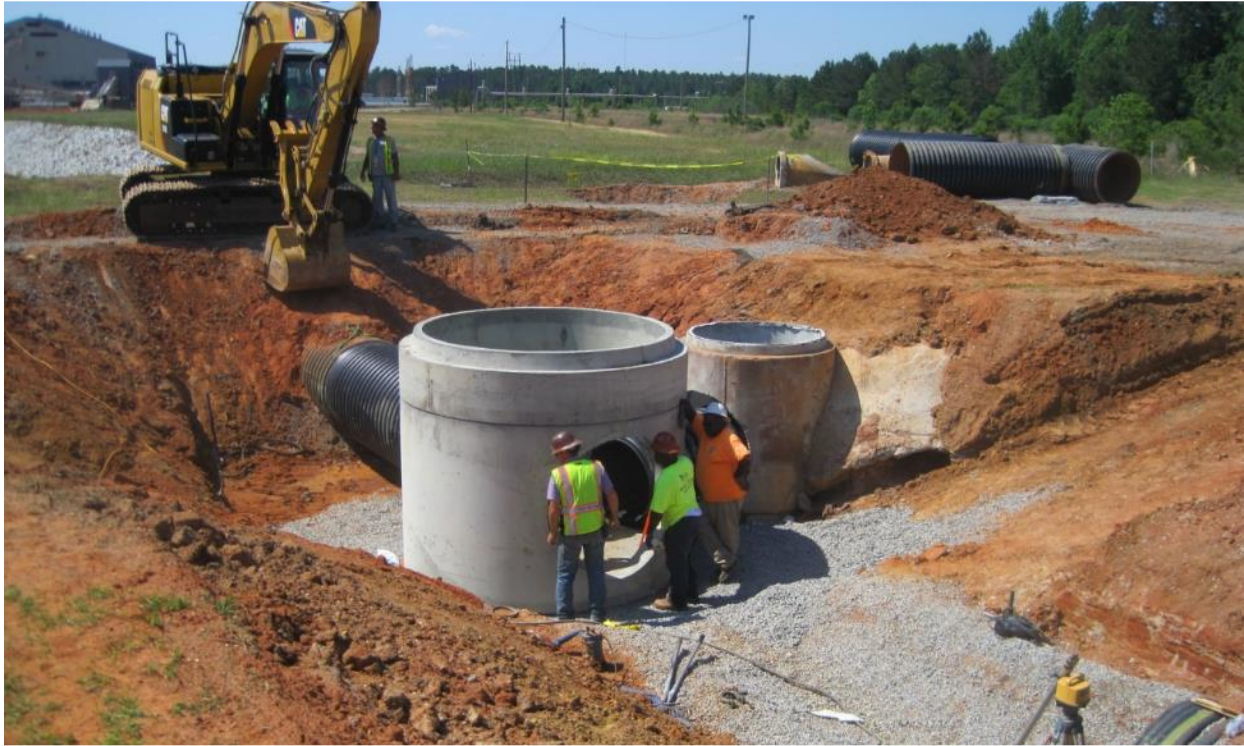
Photo 41. 489-D CPRB New Manhole in Place
