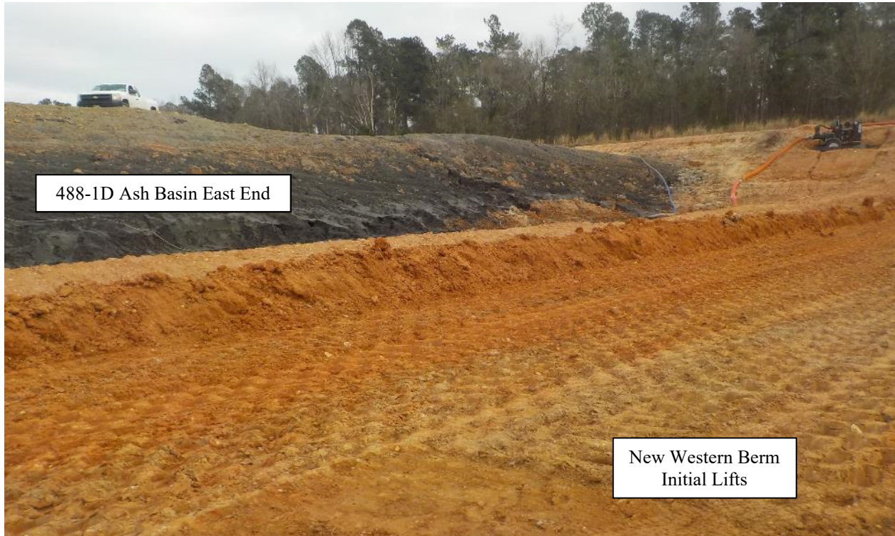
Photo 59. 488-1D Ash Basin (February 2018)
