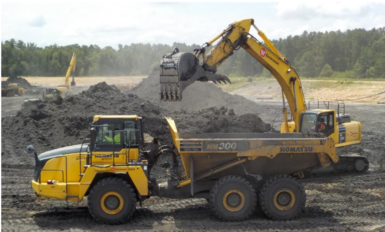
Photo 49. 488-1D Ash Basin Loading /Hauling of Processed Ash
