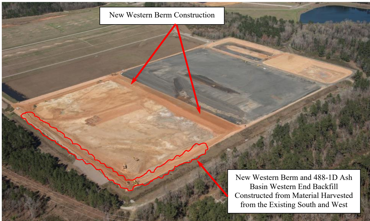
Photo 58. 488-1D Ash Basin (February 2018)
