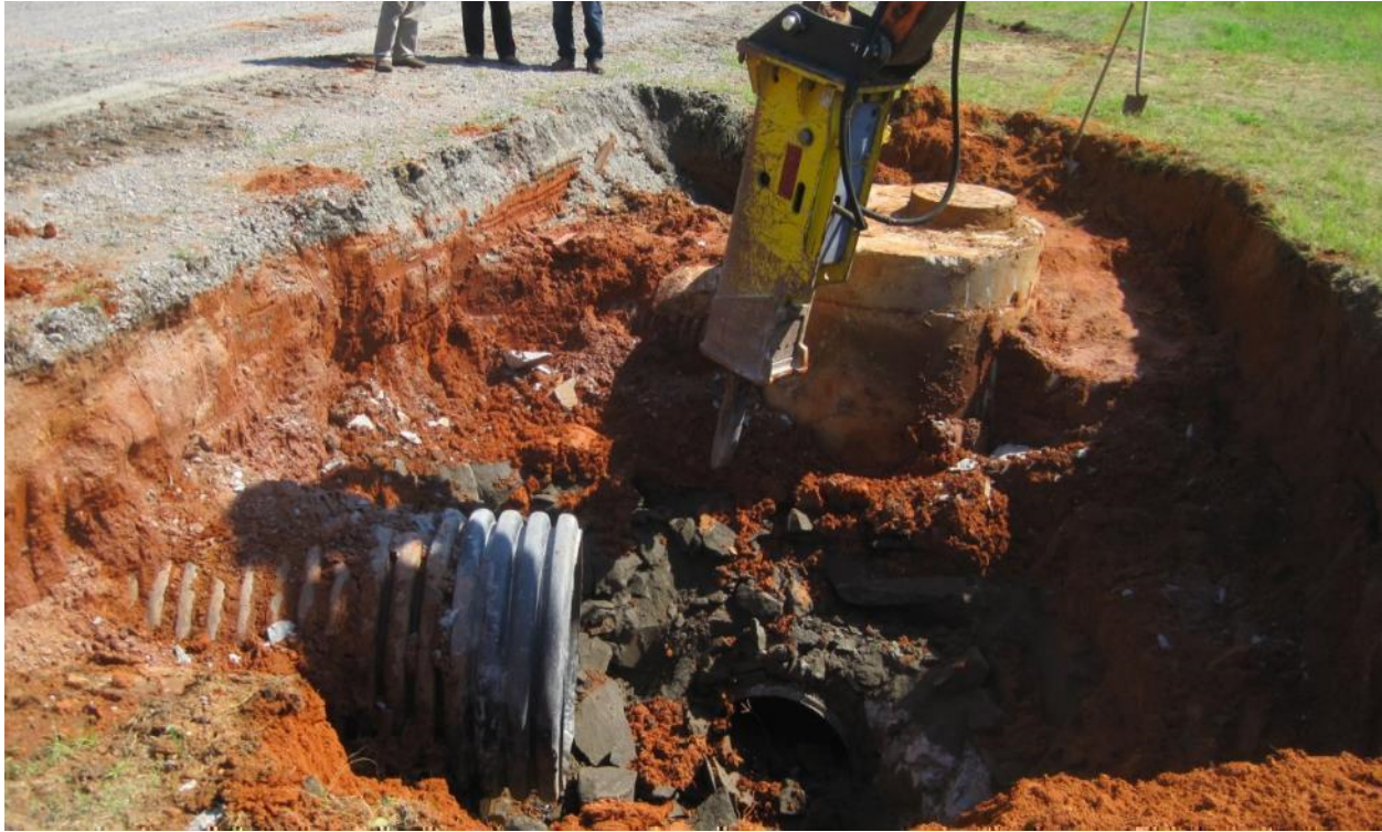
Photo 39. 489-D CPRB Removal of Existing Manhole
