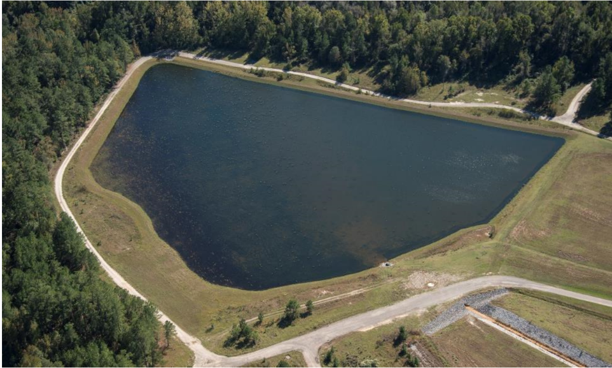
Photo 43. 489-D CPRB Aerial After Completion
