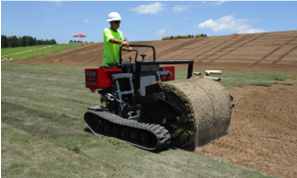
Photo 17. Tracked Sod Installer
