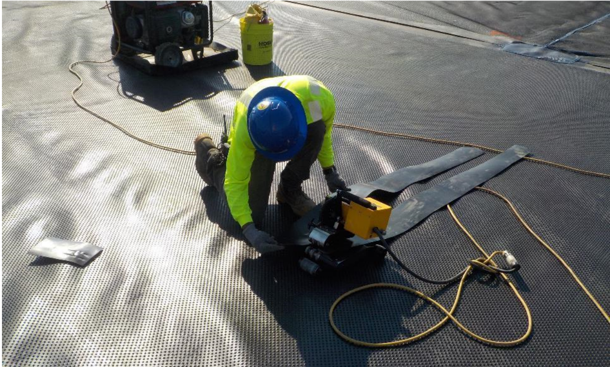
Photo 79. LLDPE Geomembrane Dual Hot Wedge Seaming (Trail Seam)
