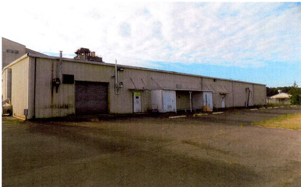
Figure 2. Building 484-4D Maintenance Facility
