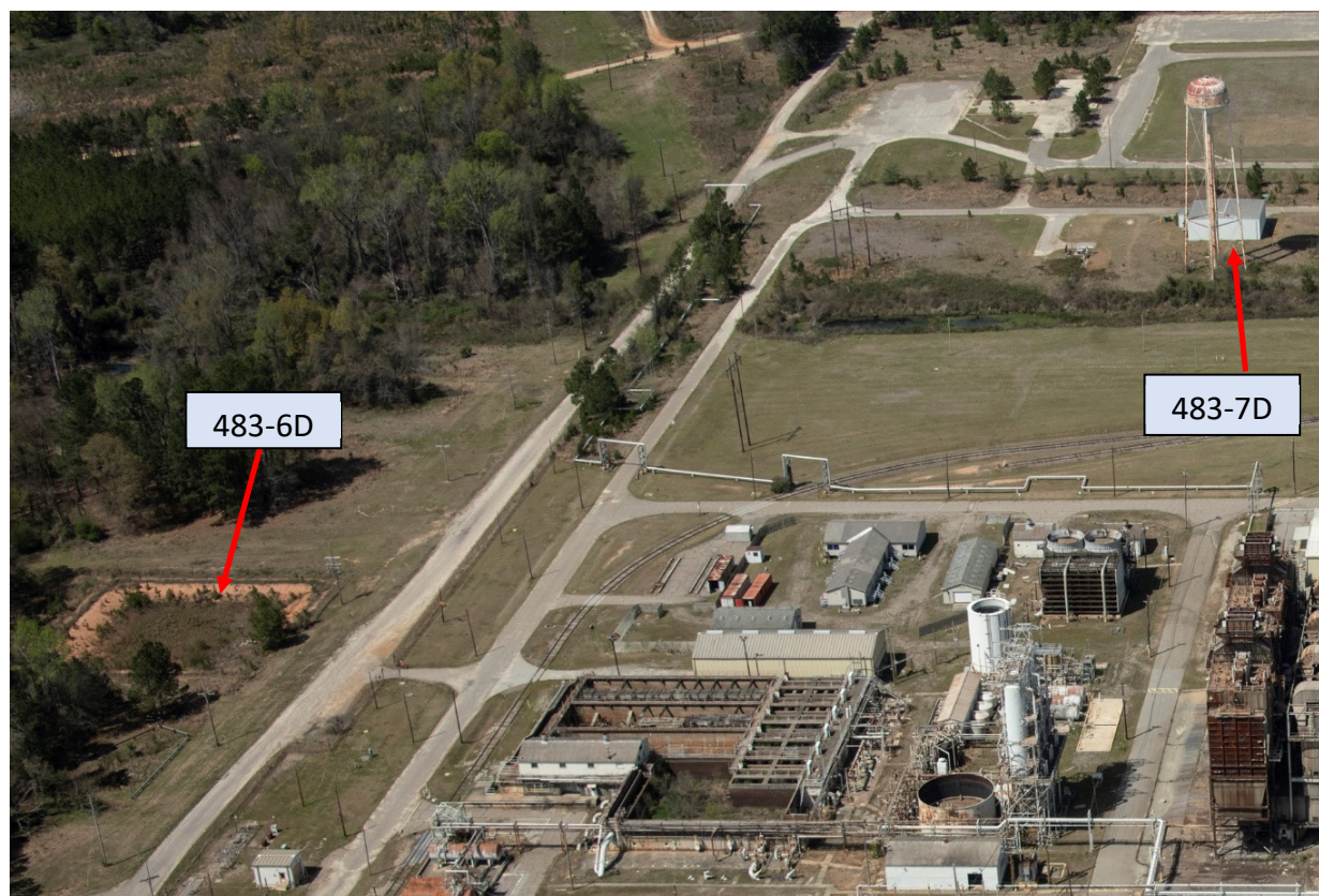
Figure 1. Location of the 483-6D Surge Basin Relative to Building 483-7D
