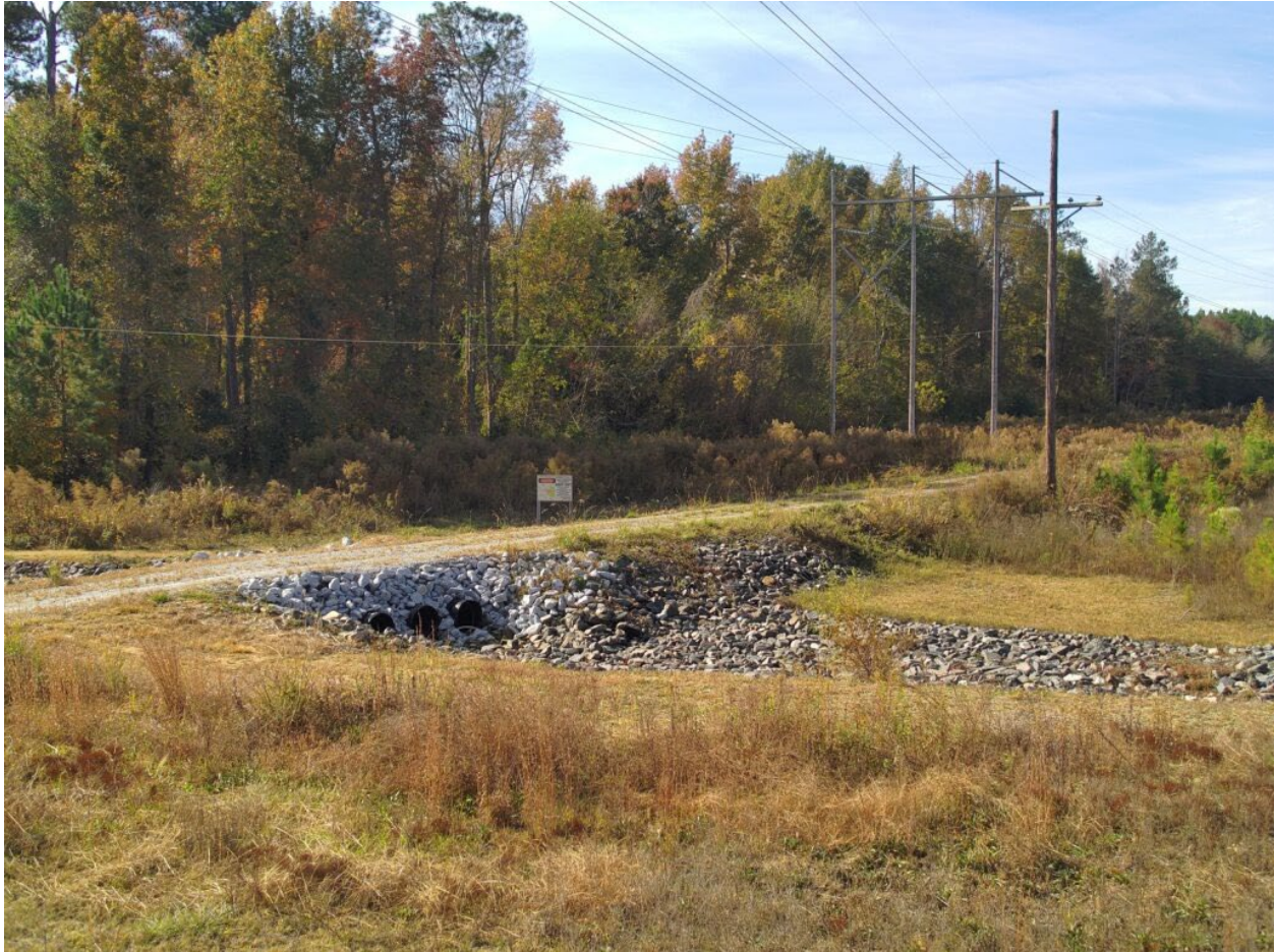
Figure 2. Wetland Area at Dunbarton Bay Entrance
