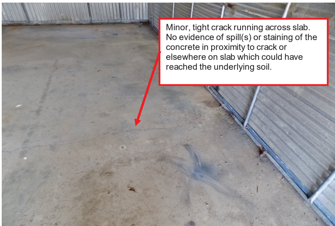
Figure 15. Building 484-5D, Interior (Looking West)
