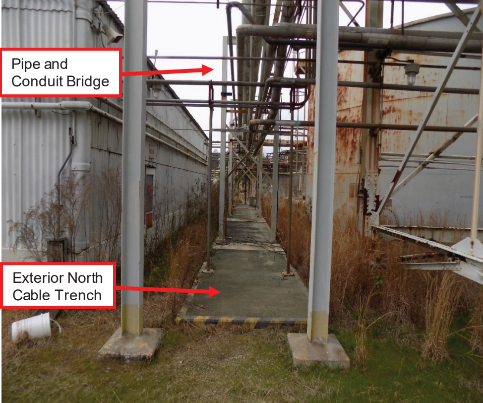
Figure 9. Building 483-3D, Cable Trench
