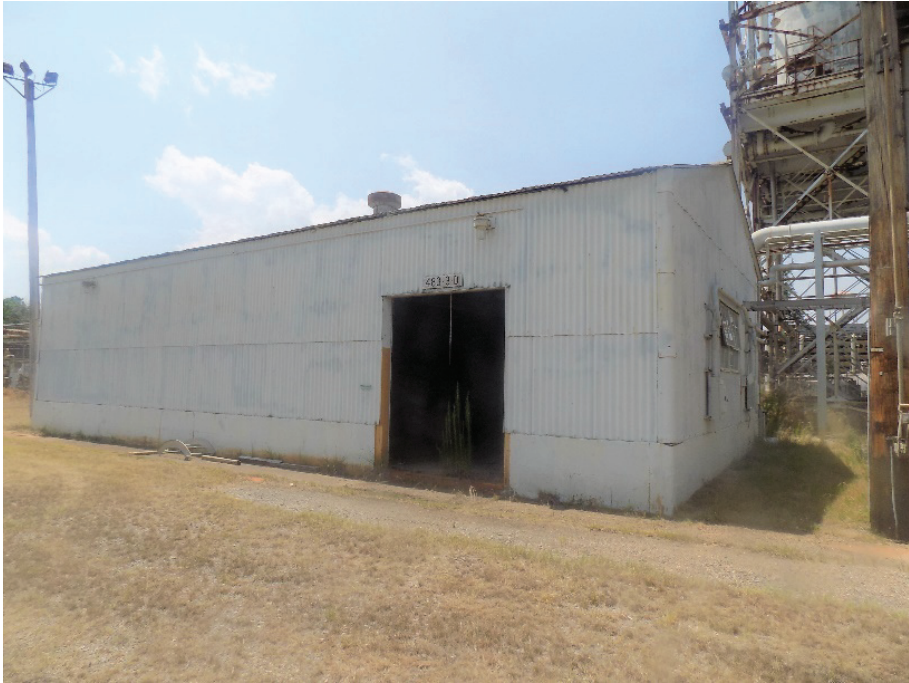
Figure 2. Building 483-3D, Electrical Control Building
