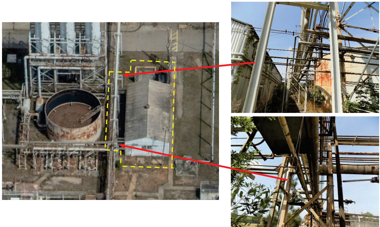
Figure 4. Building 483-3D, Above-ground Pipe Chase Showing Supports to Remain
