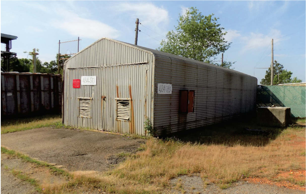
Figure 12. Building 484-5D, D-Area Powerhouse Storage Building
