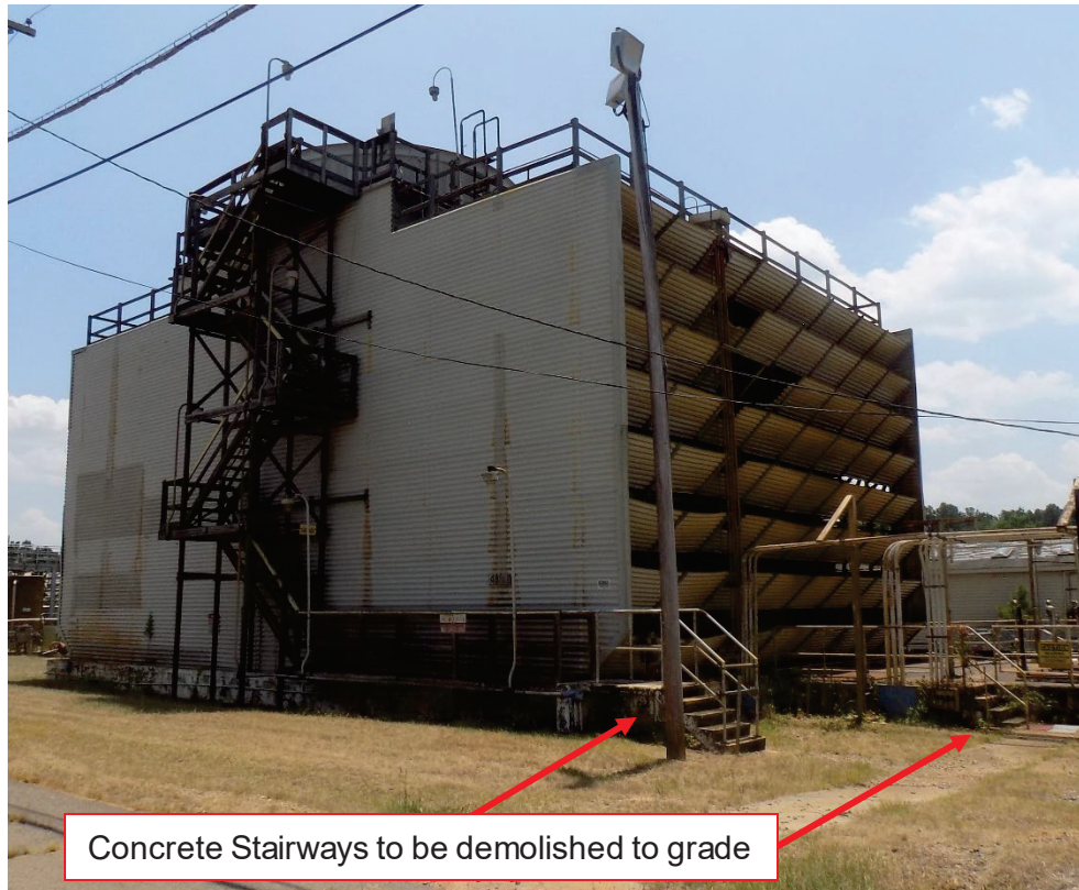
Figure 26. Building 485-D, D-Area Cooling Tower Concrete Stairways
