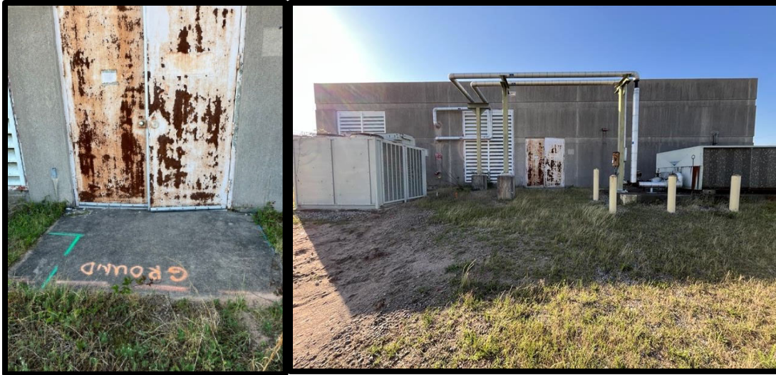
Figure 7. Doorway Pad to Mechanical Room – Northern Side of 720-F.
