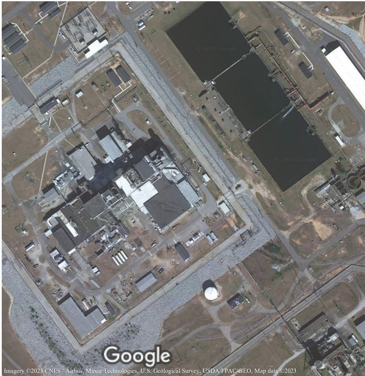
Figure D-4. Aerial View of the K-Reactor Complex (2023)
