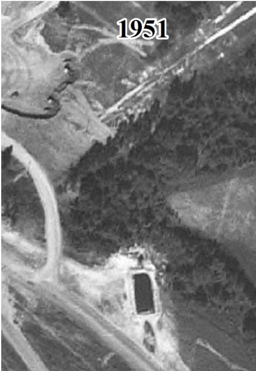
Figure H-3. Aerial Photo of the Heavy Equipment Wash Basin and Central Shops Burning/Rubble Pit (631-5G) in Operation in 1951
