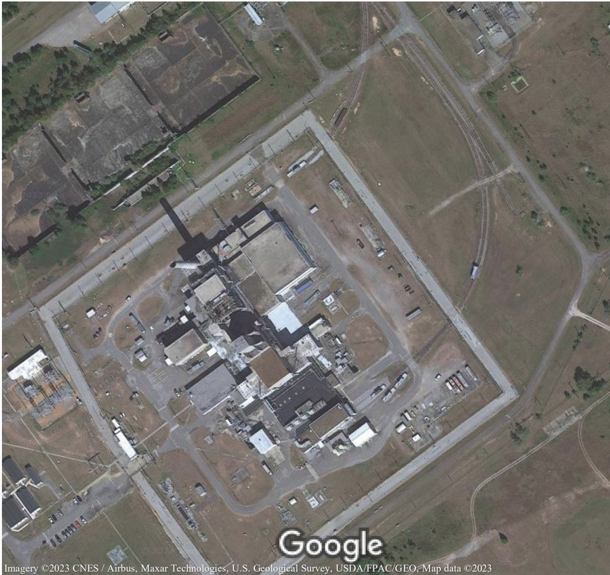
Figure D-5. Aerial View of the L-Reactor Complex (2023)
