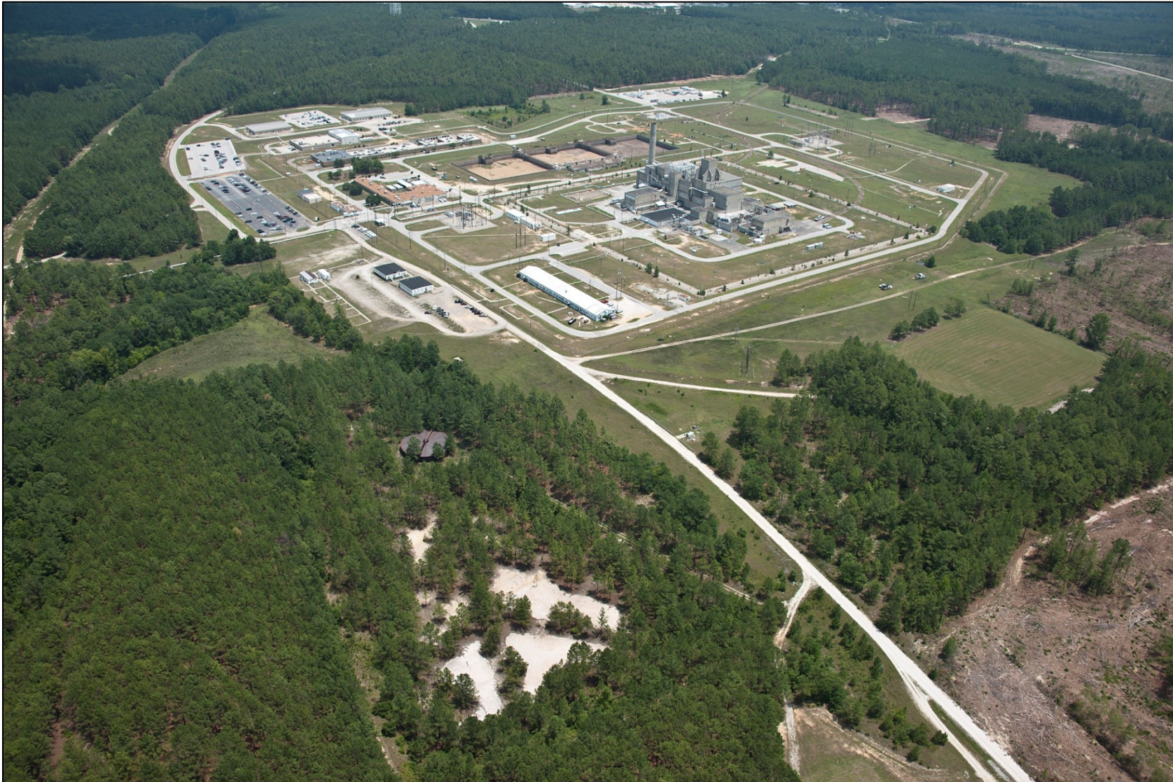
Figure C-2. Aerial Photograph of CAOU (2011)
