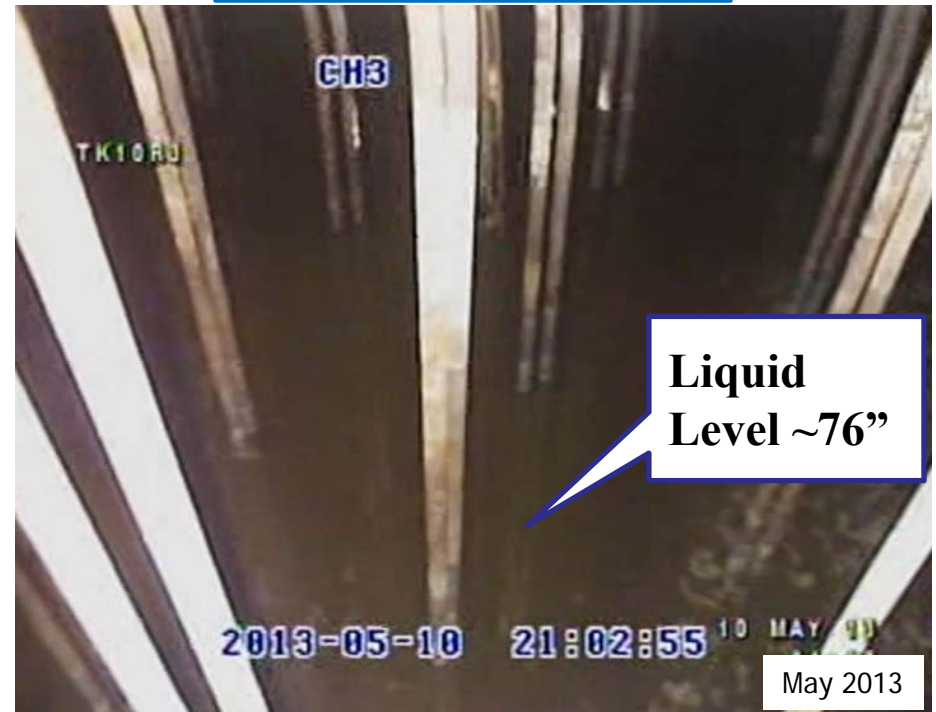
Tank 10 Riser 3 After SCD Saltcake Removal
