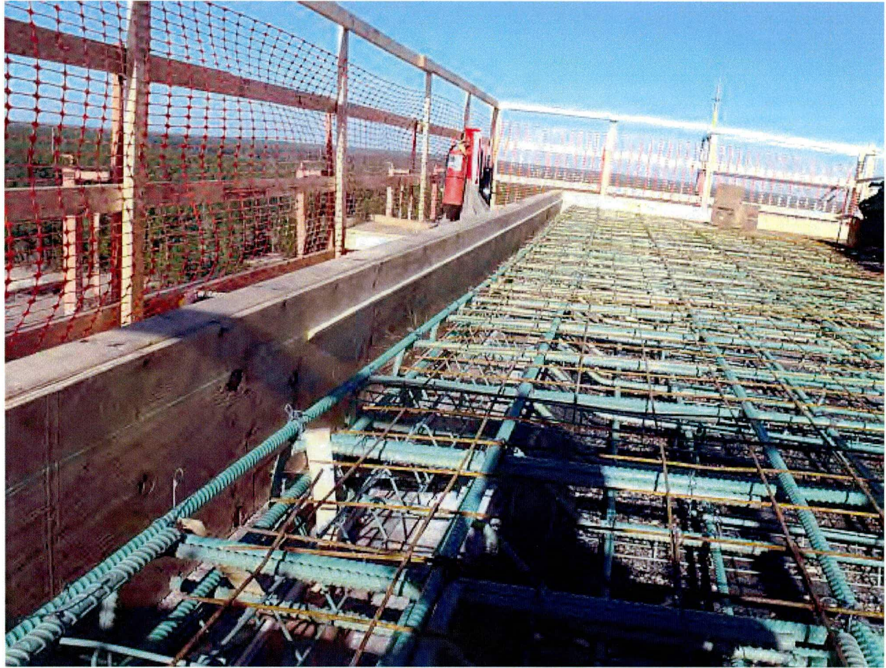
105-P Actuator Tower Roof Prep
