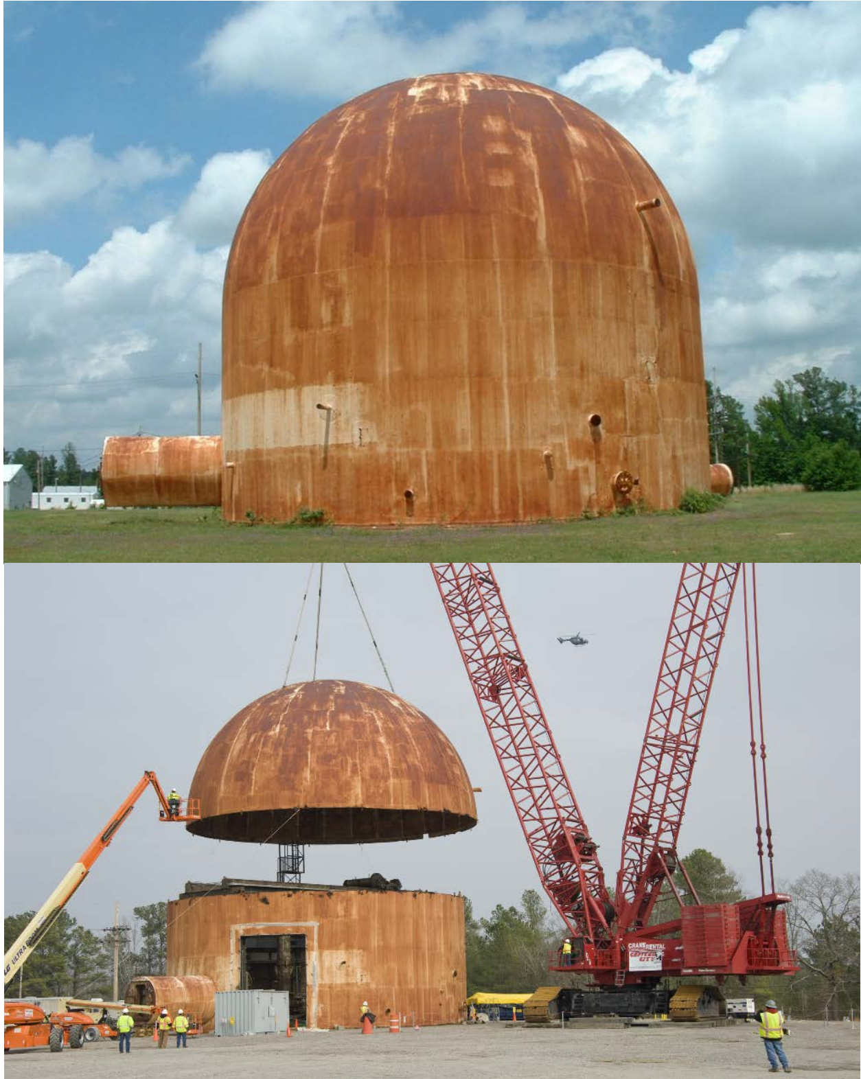
Figure C-3. Photographs of HWCTR Prior to (2009) and During Remediation (2011)
