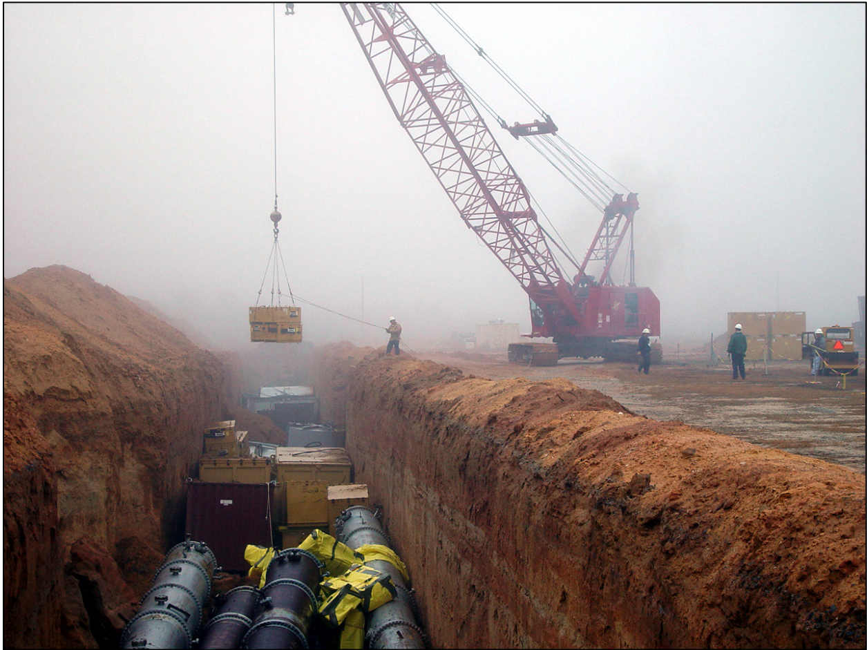
Figure F-5. Slit Trench Disposal Unit Operations (November 2008)
