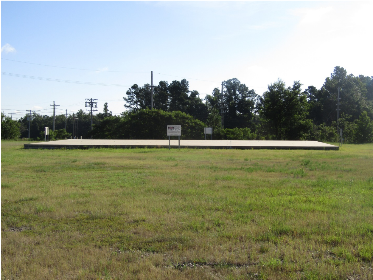
Figure C-4. Photograph of the Remediated HWCTR (2016)
