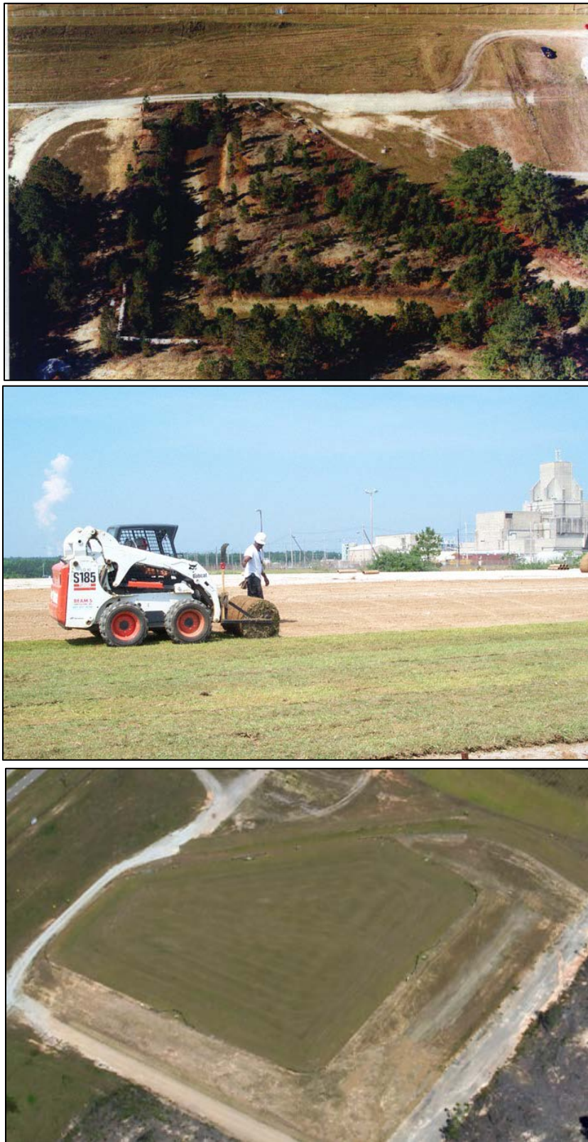
Figure L-4. Before, During, and After Remedial Action at LRSB OU
