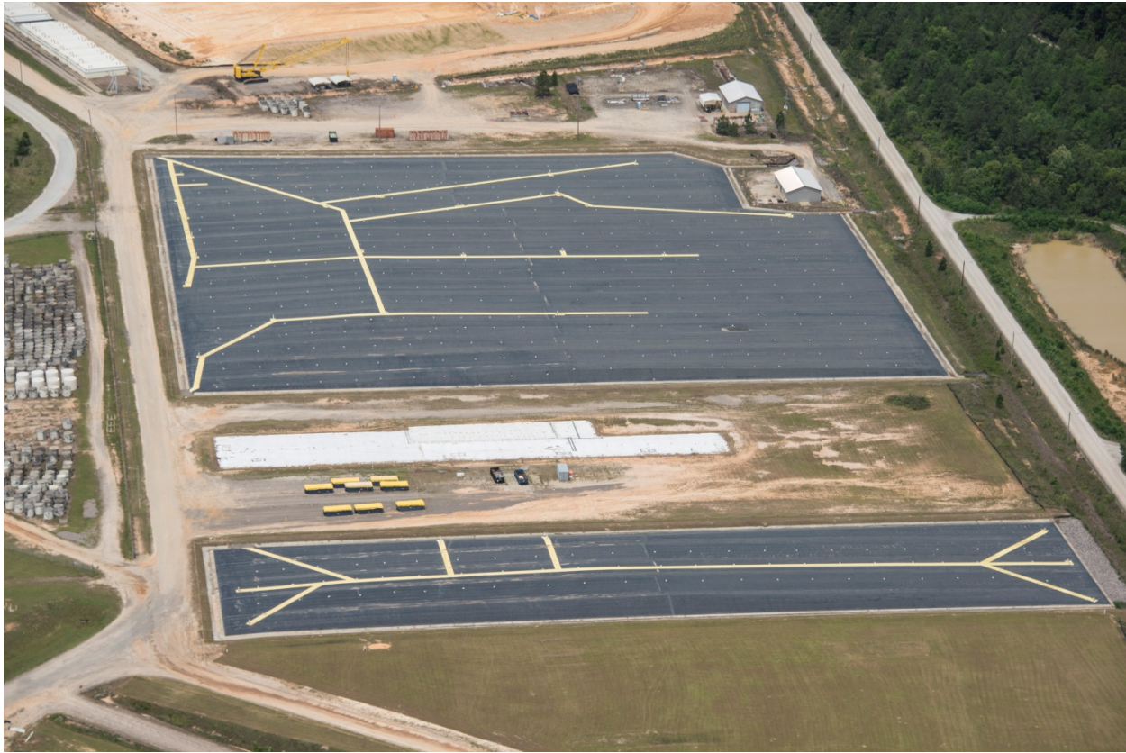
Figure F-6. E-Area LLWF Stormwater Runoff Covers for Slit Trench Disposal Units 1 – 5 (2015)
