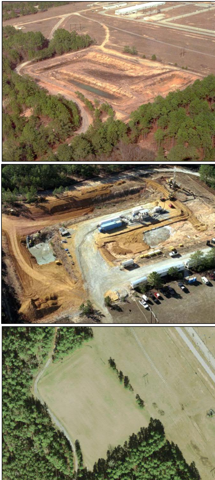
Figure L-5. Before, During, and After Remedial Action at CRSB OU Basin 2
