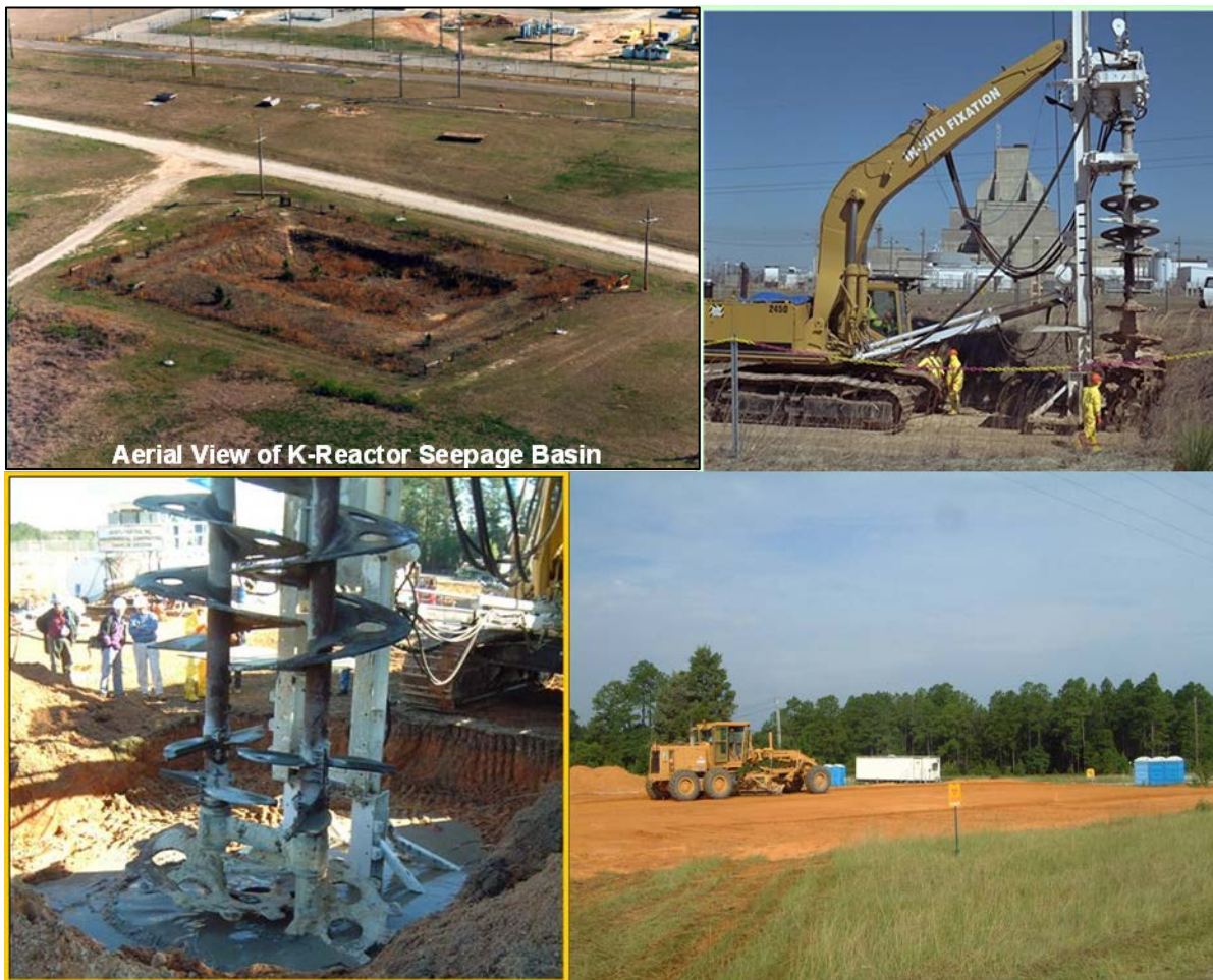
Figure J-3. Photographs Before and During Remedial Action
