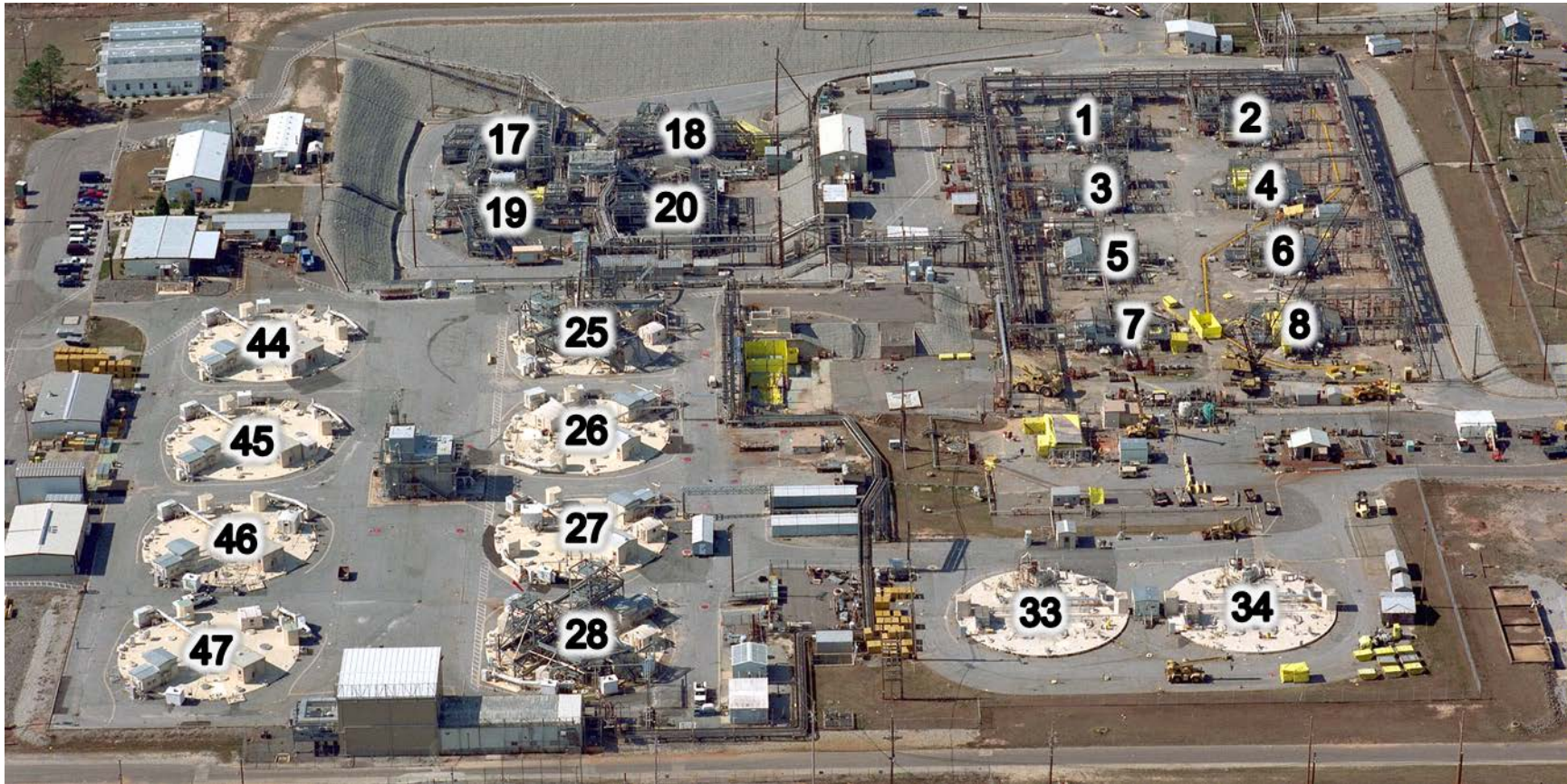
Figure H-6. Current Photograph of FTF (2015)
