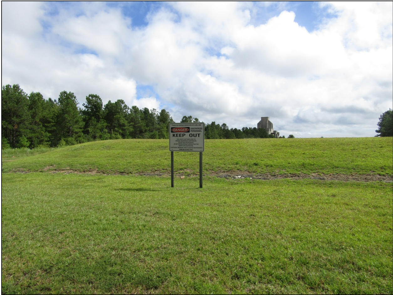
Figure O-5. Photograph of the PRSB OU Cover System (P-Reactor in the Background) (2016)
