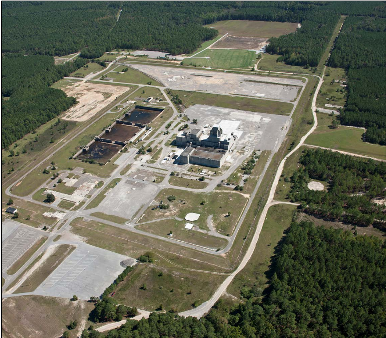
Figure N-3. Photograph of PAOU after Remedial Activities (2011)
