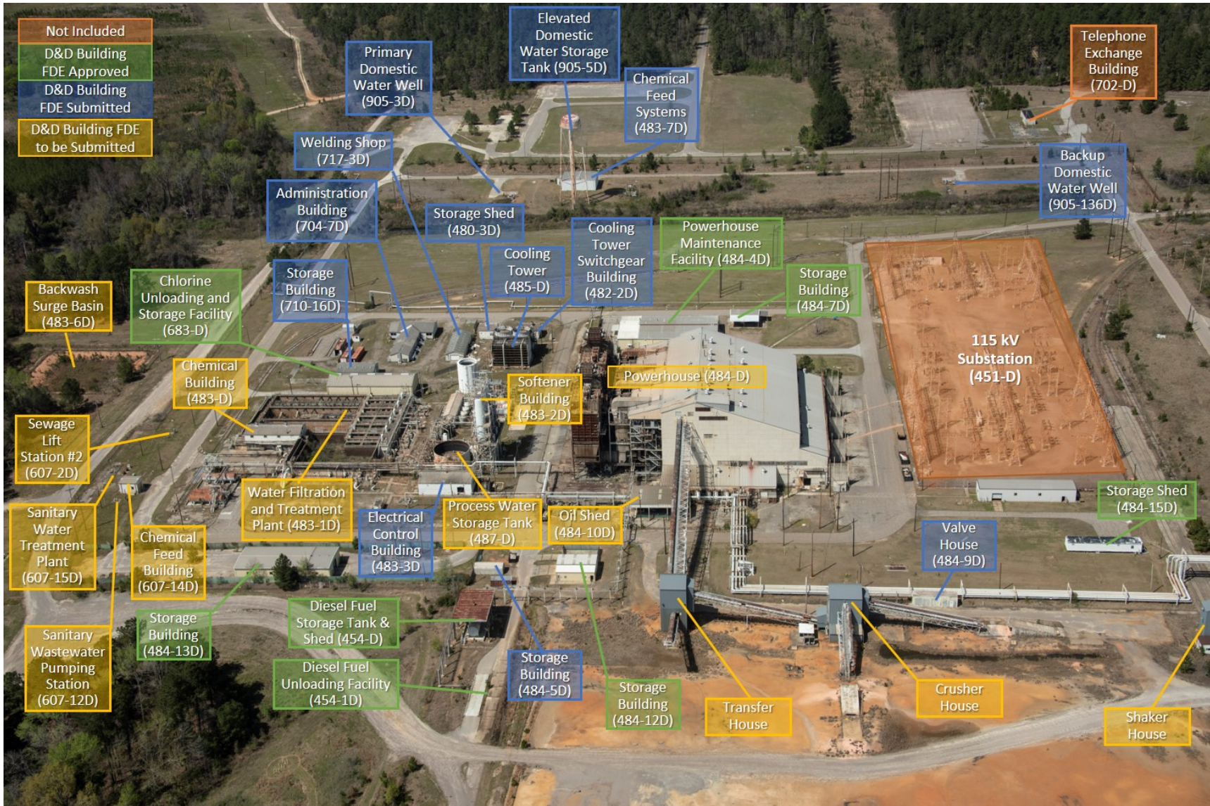
Figure 9. DAOU D&D Facilities and FFA Waste Units
