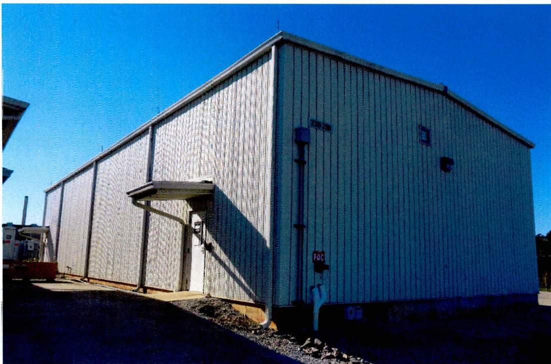
Figure 4. Building 233-23H Looking Northwest
