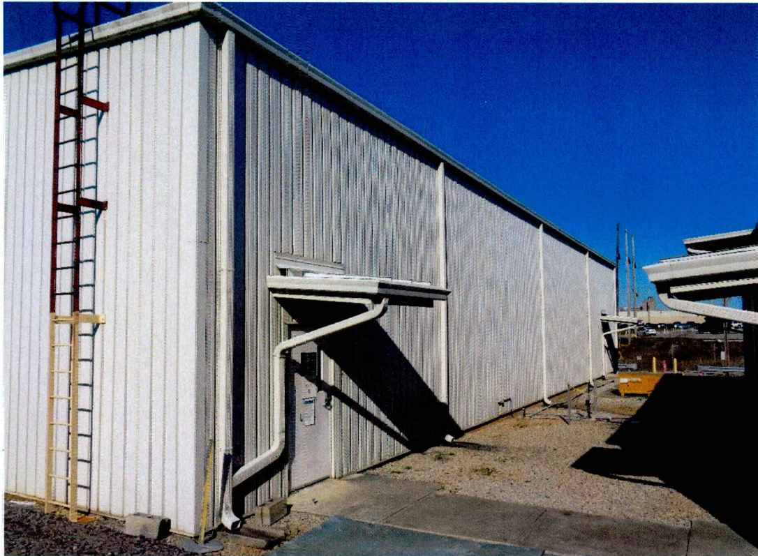
Figure 3: Building 233-23H Looking Northeast
