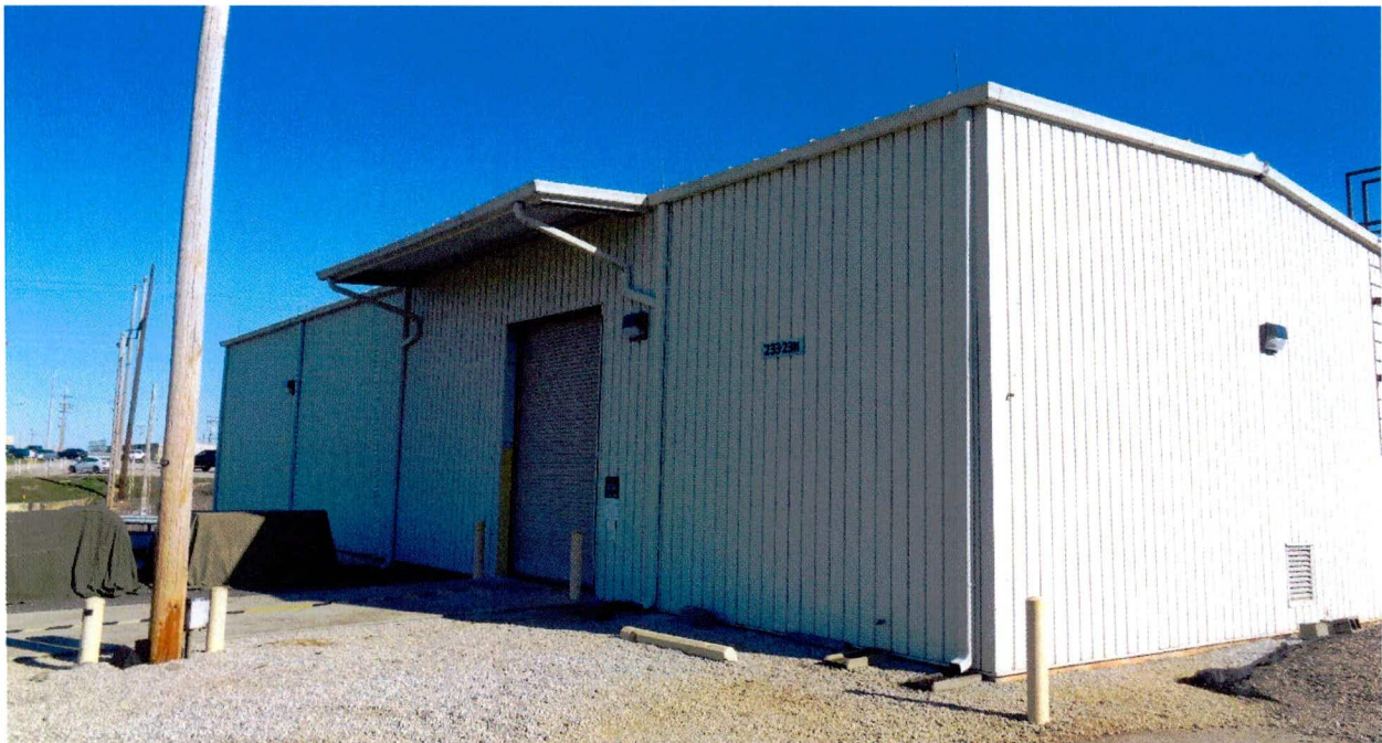
Figure 2. Building 233-23H Looking Southeast
