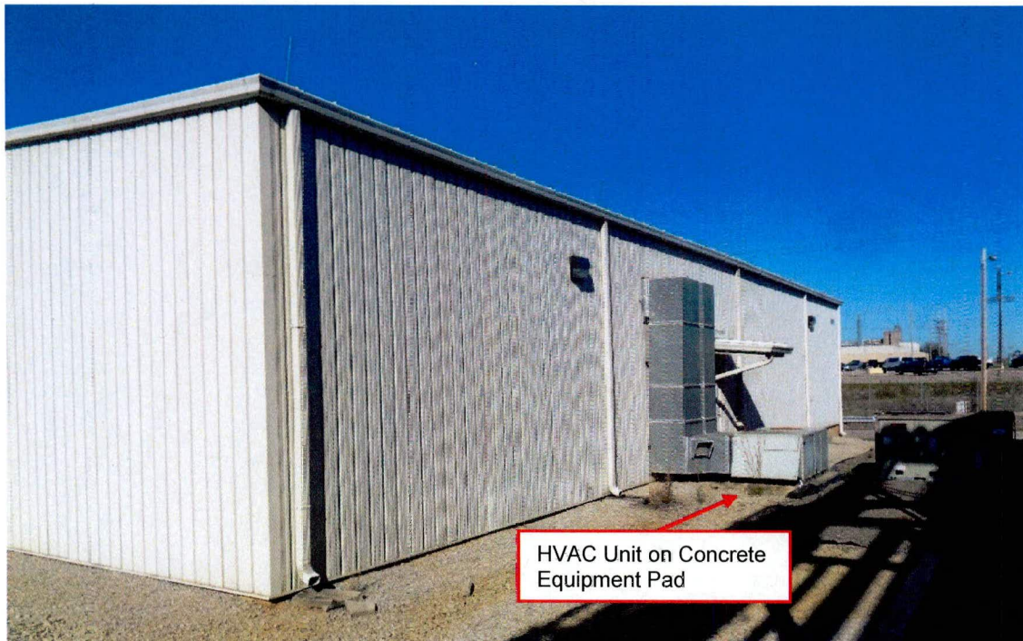
Figure 7: 233-24 H Looking Northeast
