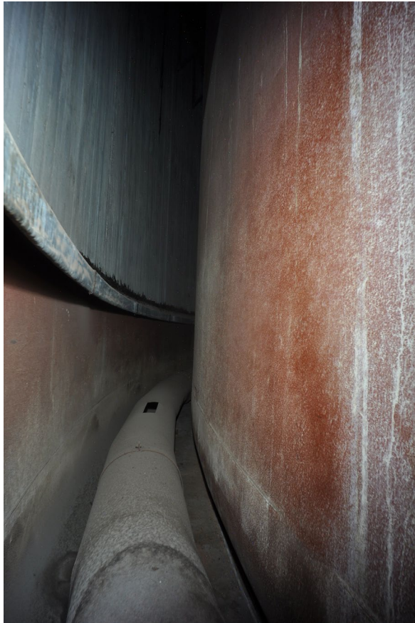
South Looking West
