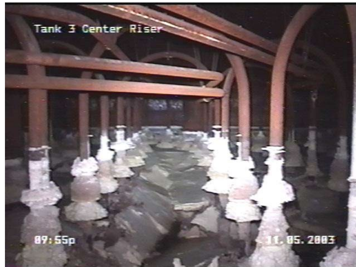
Tank 3 During Interstitial Liquid Removal
