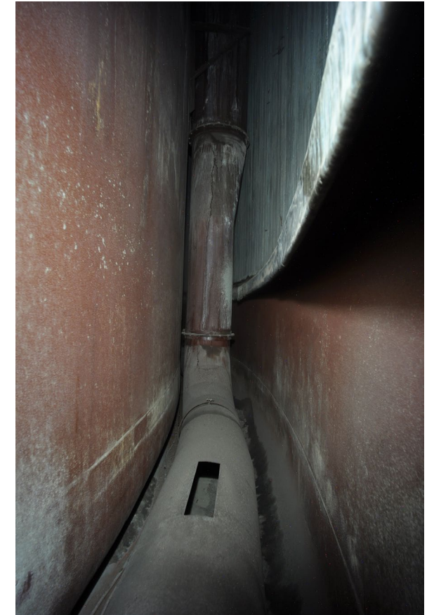
West Looking South
