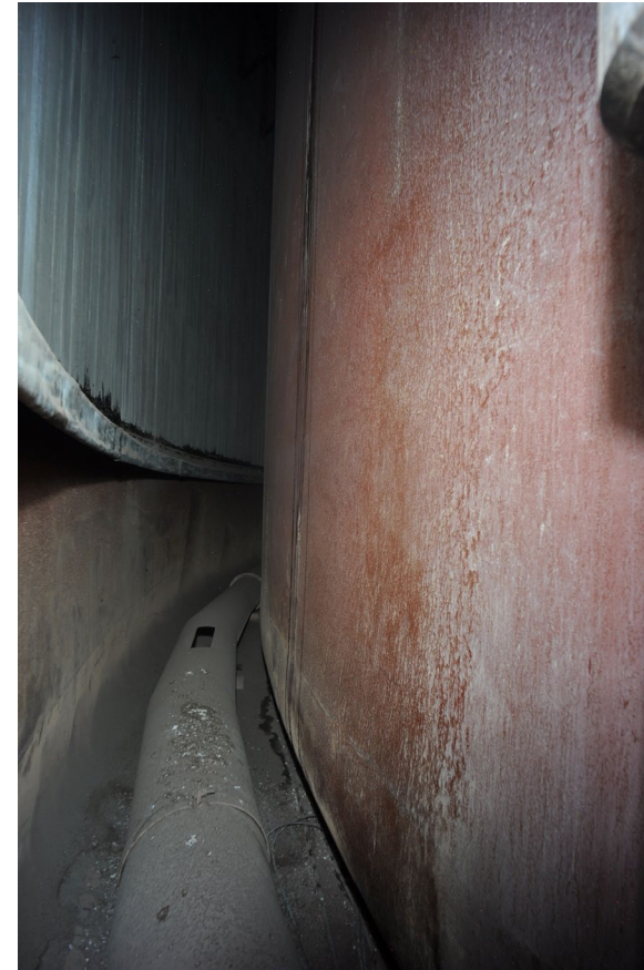
North Looking West
