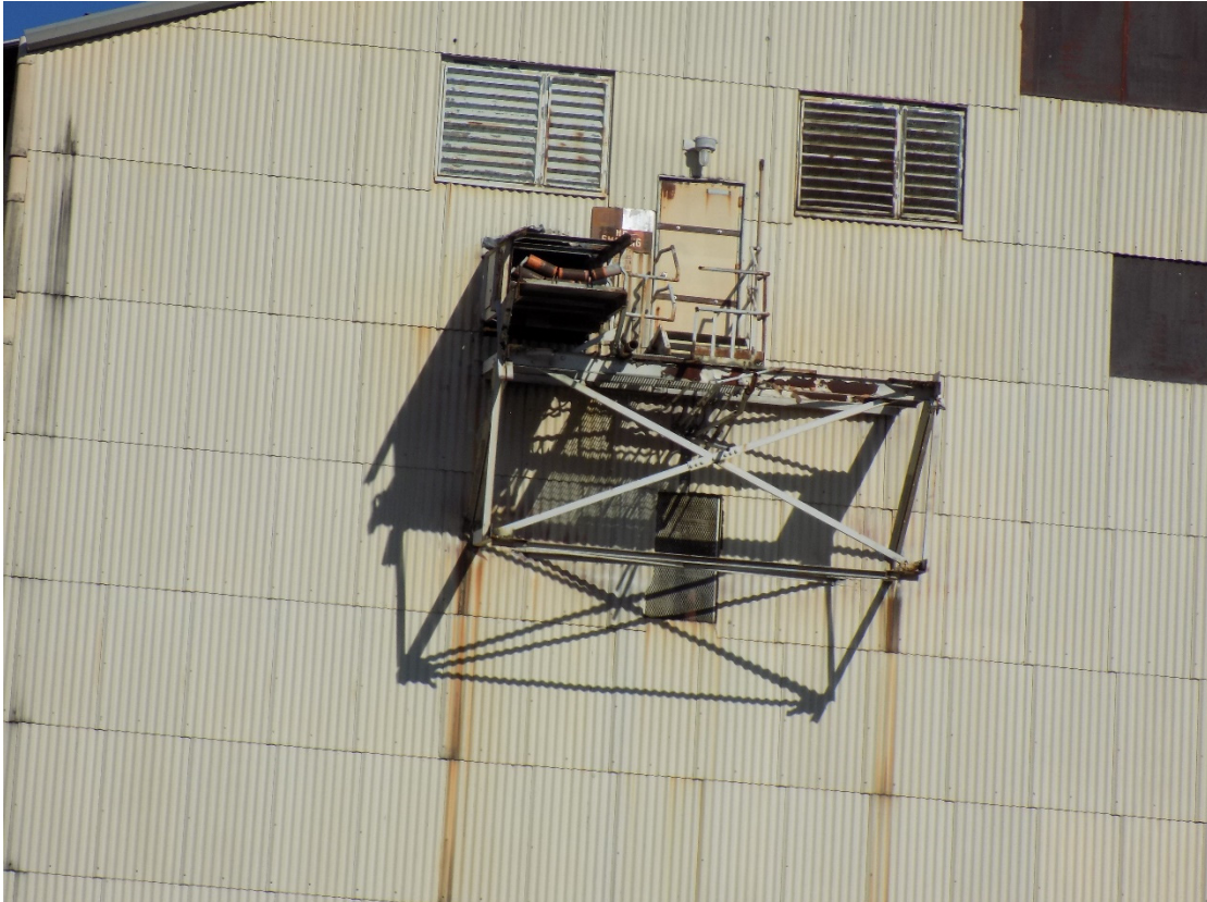
Figure A-23: Conveyor #3 After Decommissioning
