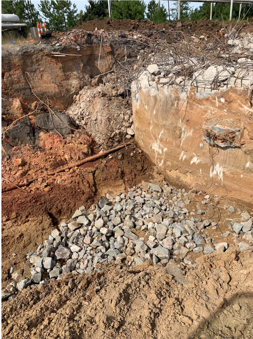
Figure B-1: Conveyor #1 Tunnel during Excavation/Fill
