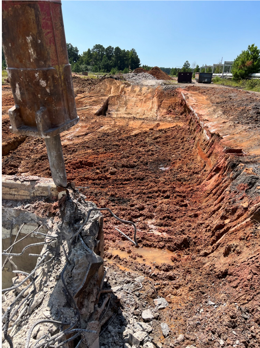
Figure B-2: Conveyor #1 Tunnel during Excavation/Fill
