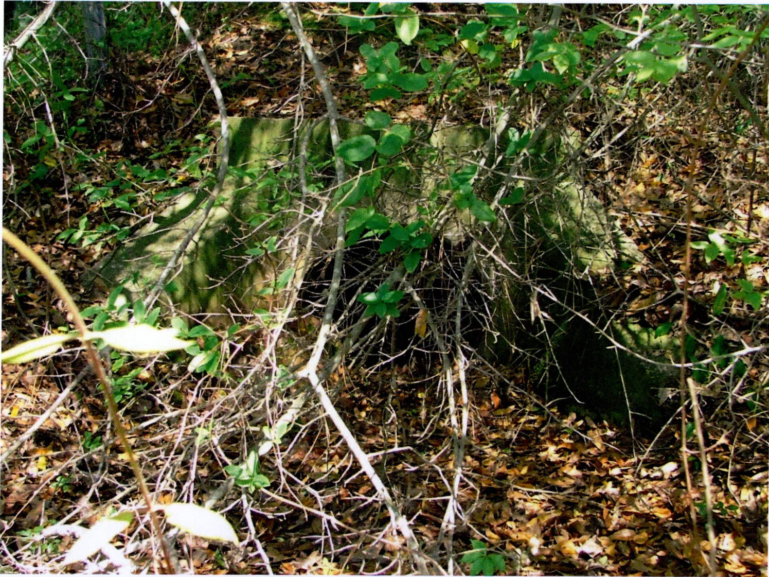
Figure 2. Photo of Stormwater Outfall A-013 (2010)
