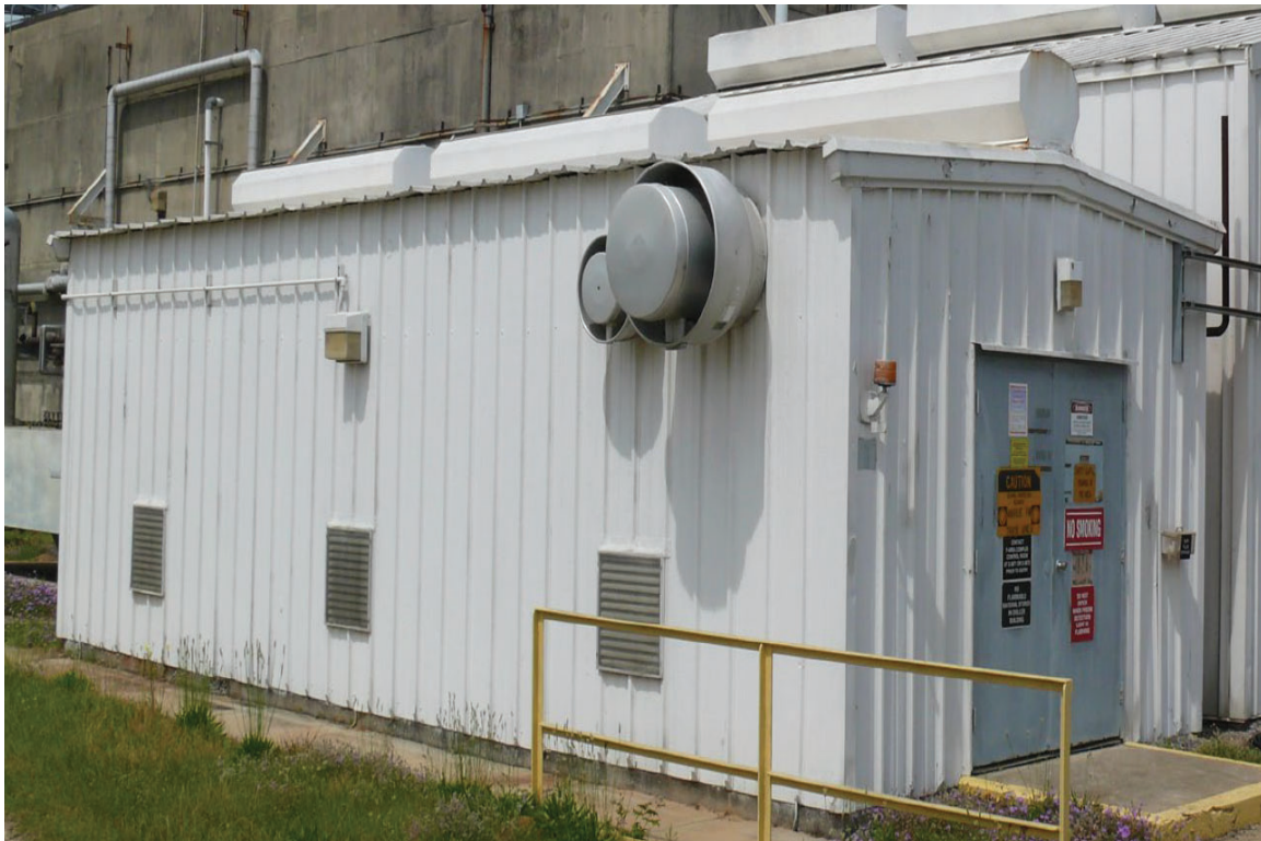
Photo 2 – Refrigeration Building No. 2 235-2F taken from south.
