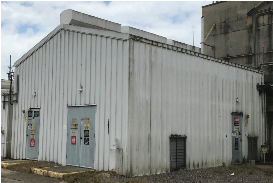
Photo 1 – Refrigeration Building No. 1 235-1F taken from east.
