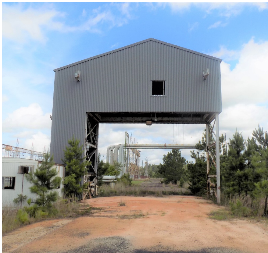
Figure 3. Coal Handling Shaker House (484-24D)
