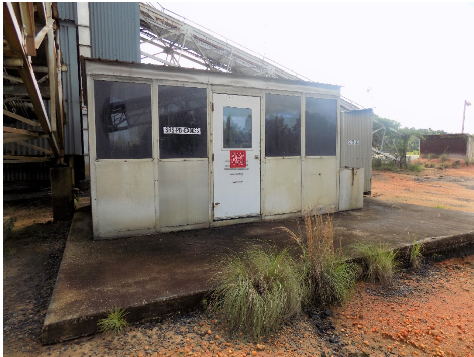
Figure 13. SRS-PB-EX0033 Coal Handling Breakroom Building for Crusher House
