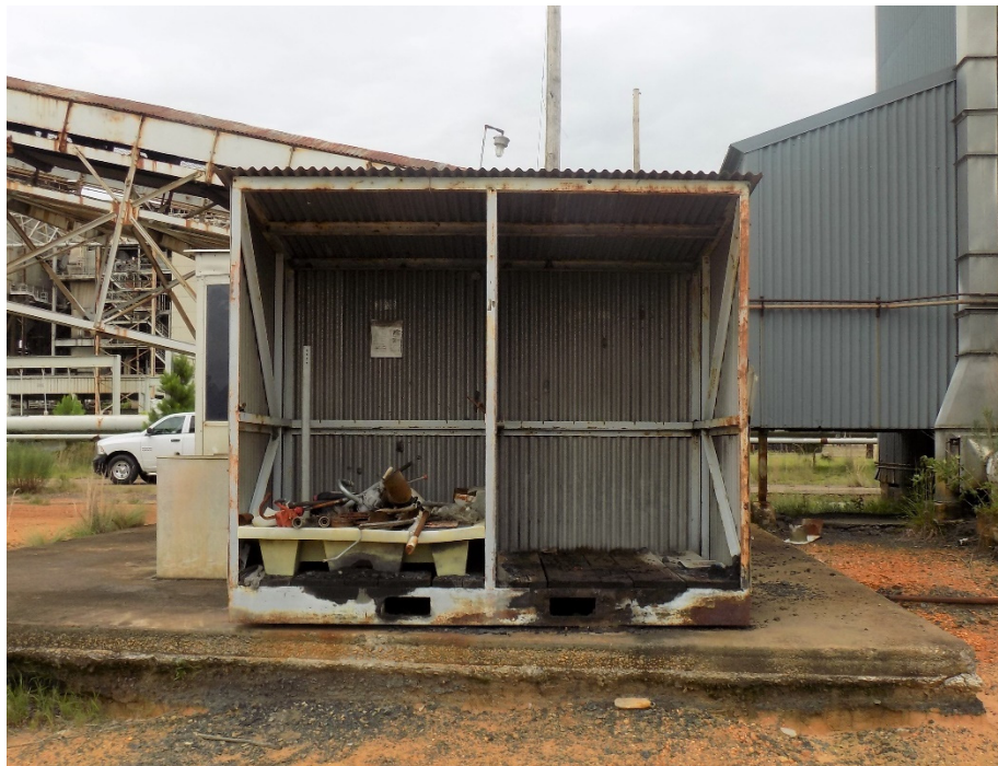
Figure 14. SRS-PB-EX0035 Storage Shed for Portable Equipment, Lube and Spare Parts
