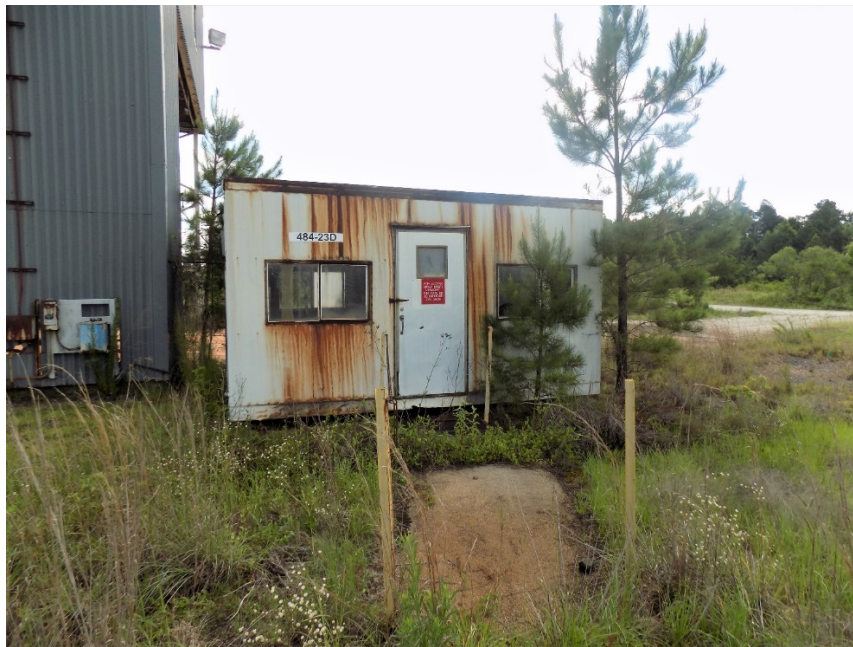
Figure 6. 484-23D Coal Handling Breakroom Building (aka SRS-EX-0032)
