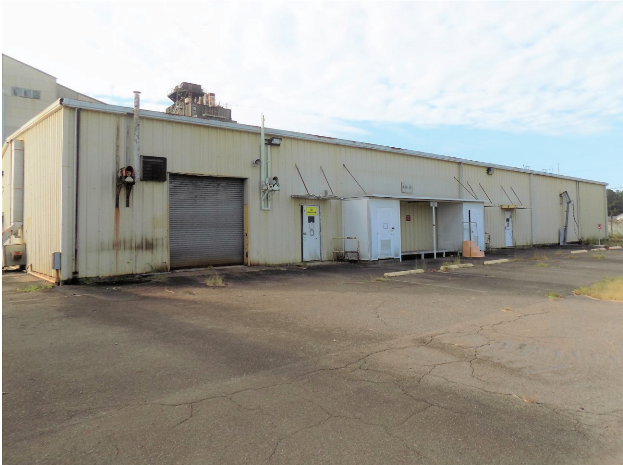
Figure A-1. Building 484-4D Before
