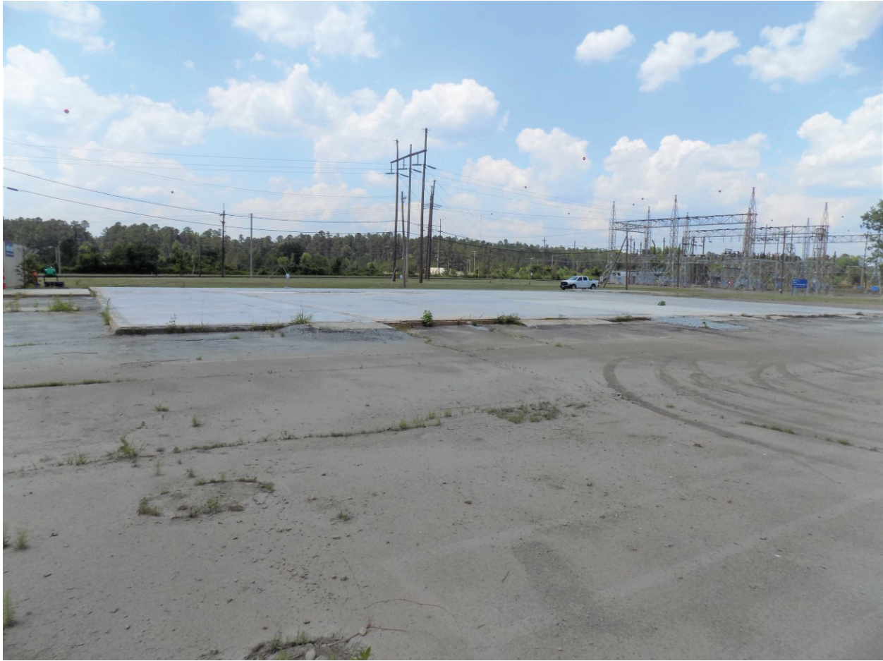
Figure A-2. Building 484-4D After
