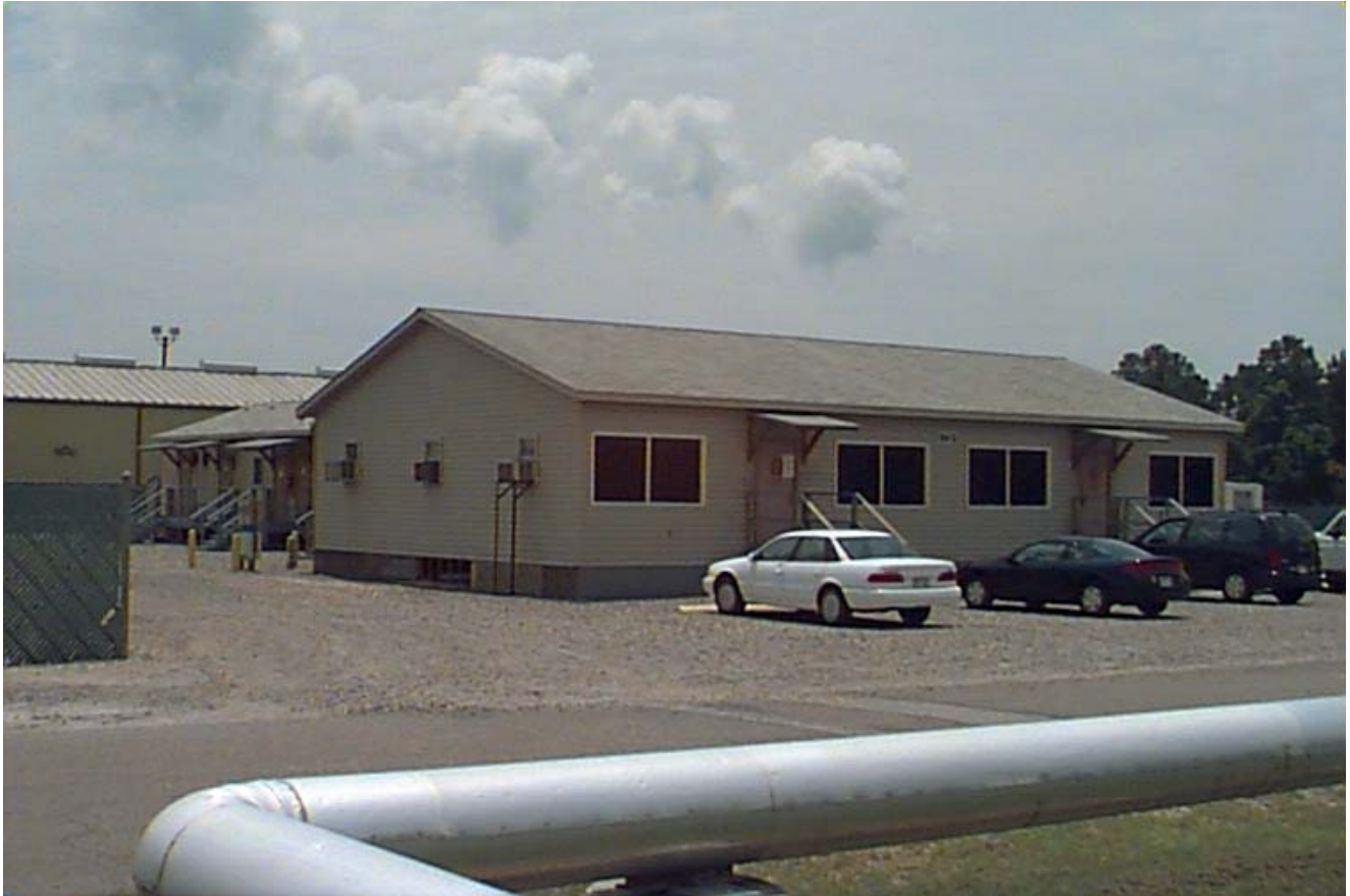
Figure 1. Building 704-7D, Maintenance Building
