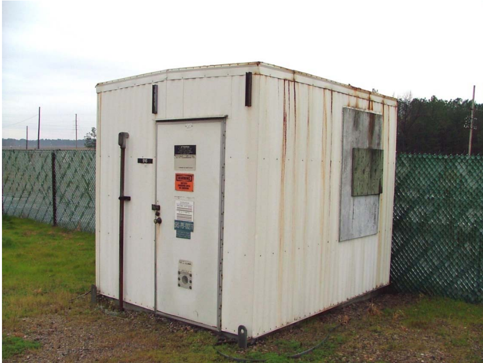
Figure 3. Building 704-7D, Ancillary Skid-Mounted Shed (PB00277)
