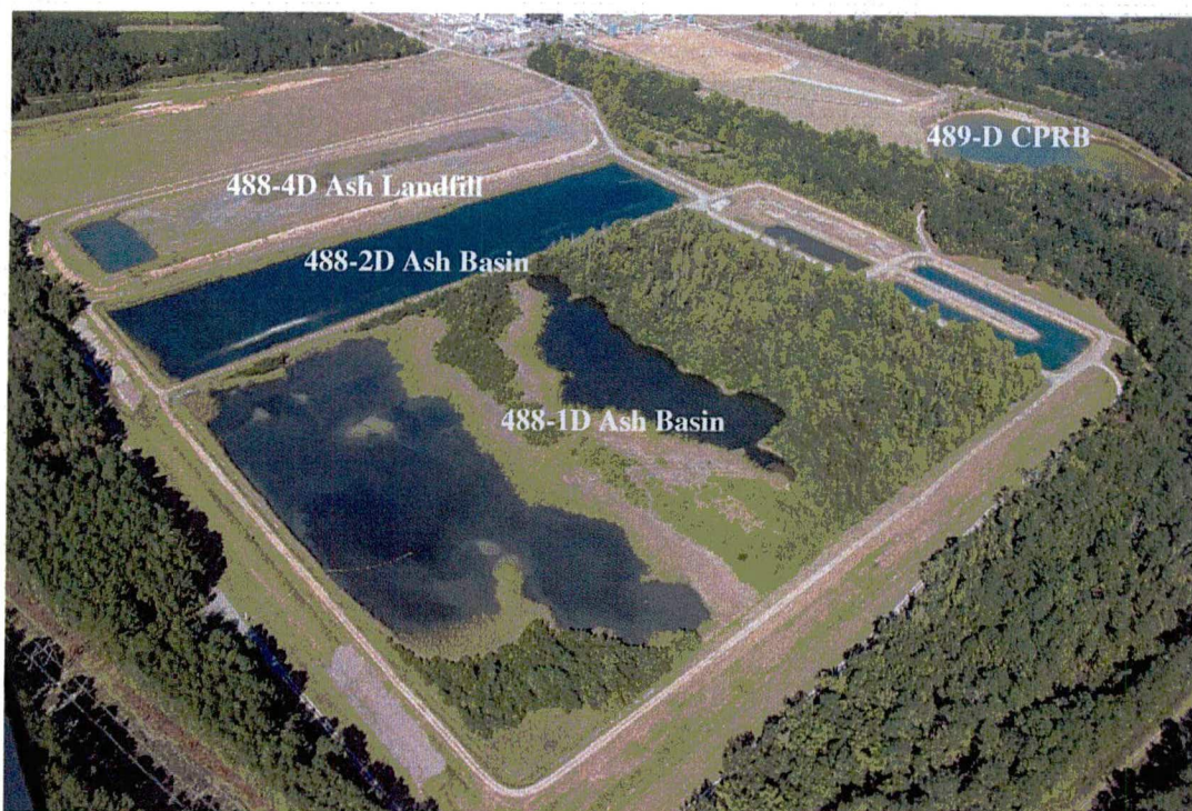
Figure 4. D-Area Project in October 2013 (Before Project Initiation)
