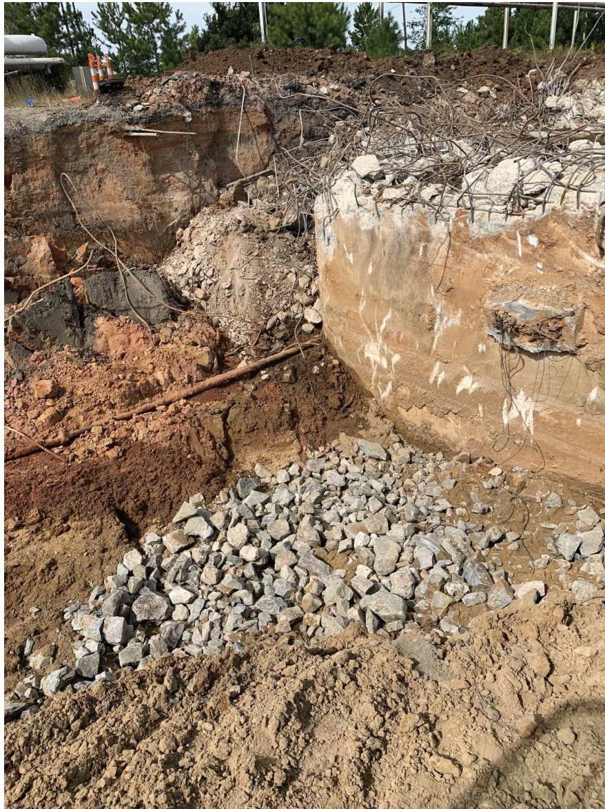
Figure B-1: Conveyor #1 Tunnel during Excavation/Fill
