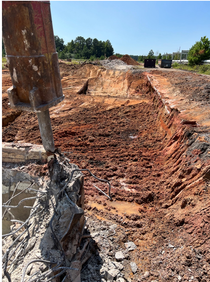
Figure B-2: Conveyor #1 Tunnel during Excavation/Fill
