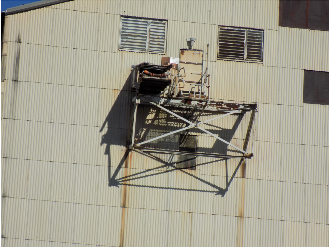
Figure A-23: Conveyor #3 and Door Exterior After Decommissioning
