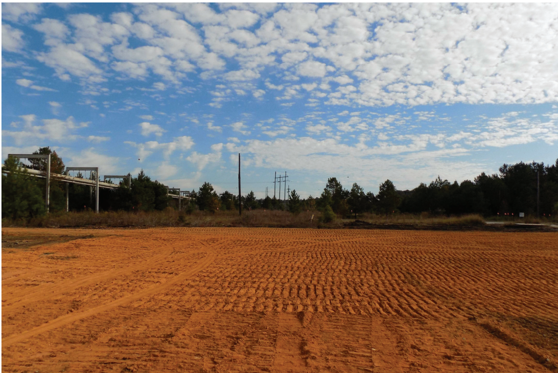
Figure A-4: 483-23D, aka SRS-PB-EX0032, (Looking East) After Decommissioning
