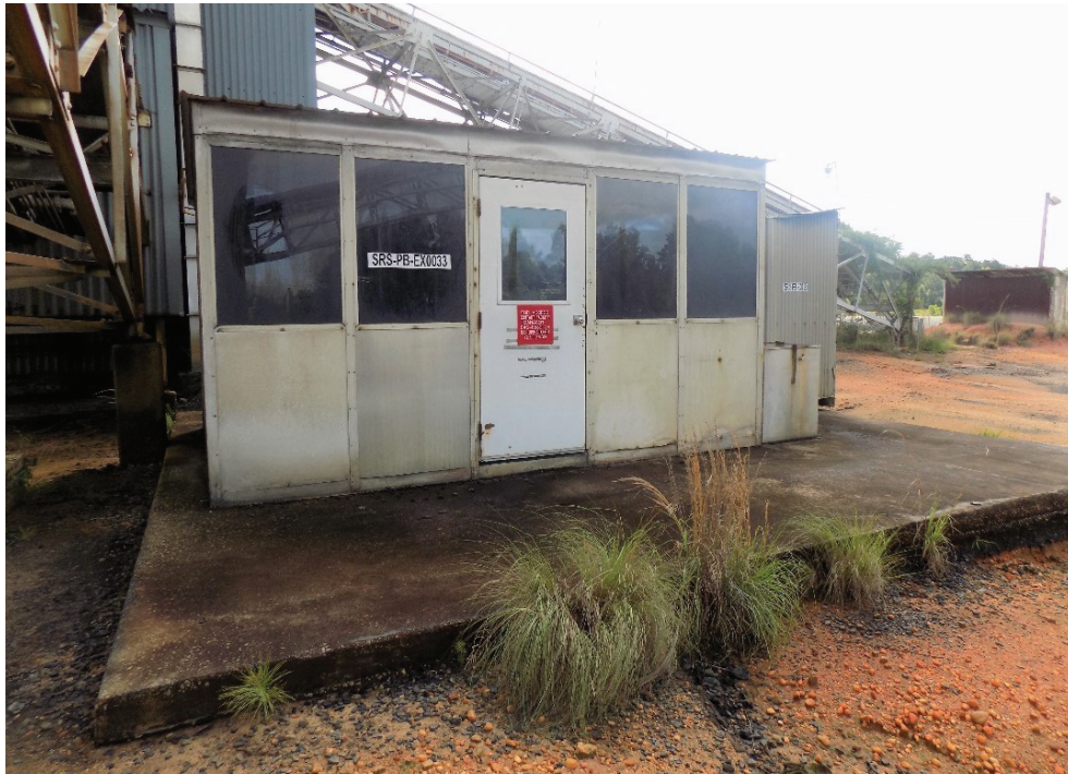
Figure A-18: SRS-PB-EX0033 (Looking Southeast) Before Decommissioning
