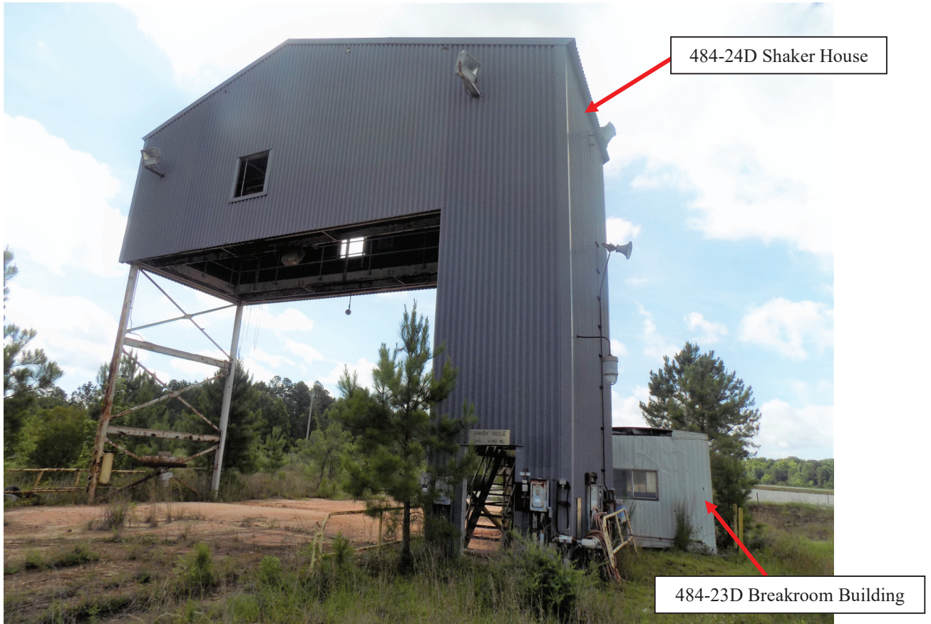
Figure A-5: 484-24D and 483-23D (Looking Southeast) Before Decommissioning
