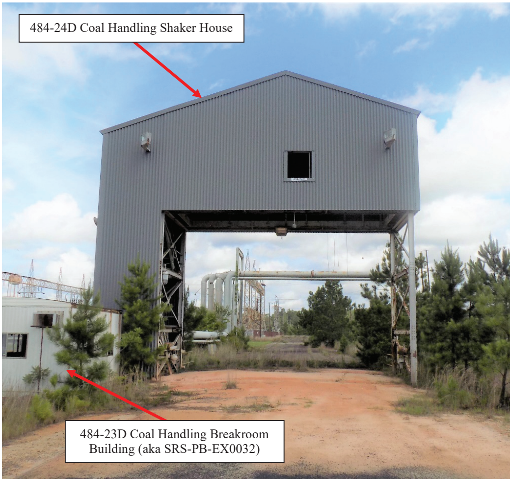
Figure A-1: Building 484-24D (Looking North) Before Decommissioning
