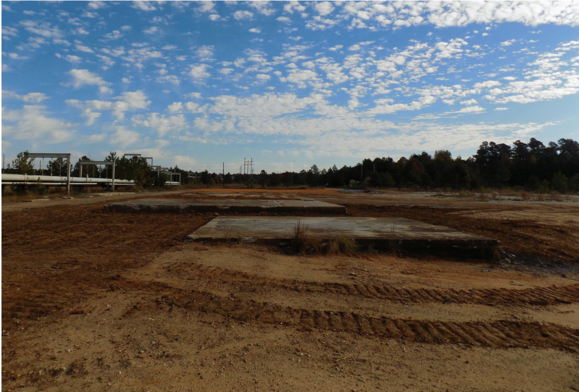
Figure A-14: 484-22D (Looking East) After Decommissioning
