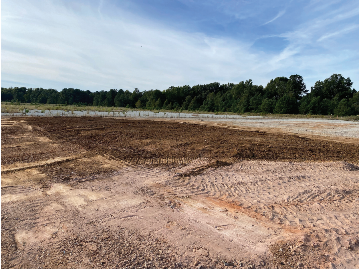
Figure A-17: Conveyor No. 4 Concrete Bunker and Reclaim Hopper (Looking Southwest) After Decommissioning
