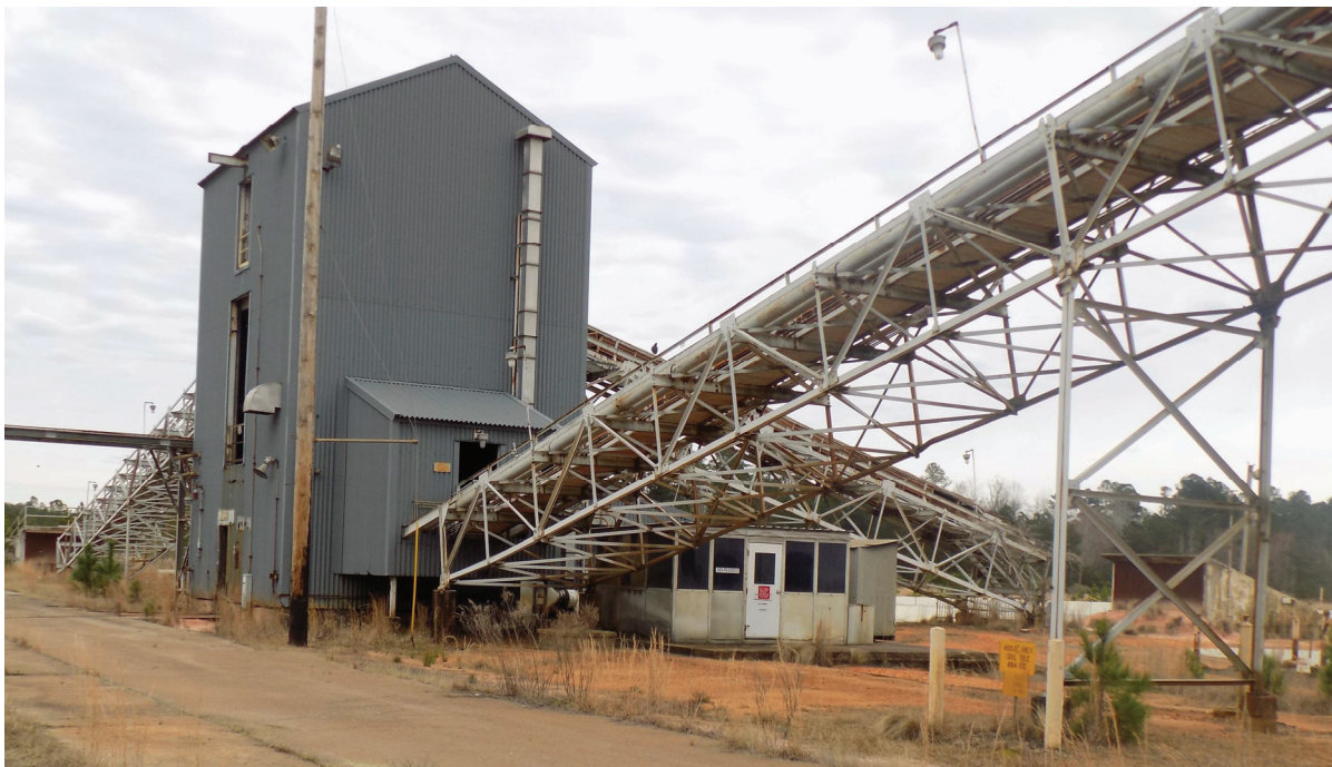
Figure A-13: 484-22D (Looking Southeast) Before Decommissioning
